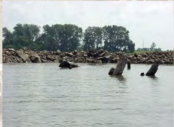
Woody structure behind dike
