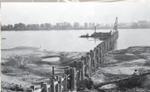
Timber piling clump dike, Chester to Ste. Genevieve, Mo., 1947
