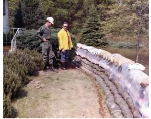
Sandbagging at Arnold, Mo. during 1973 flood
