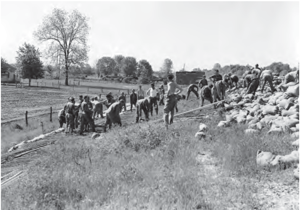
Flood fighting efforts at Swan Drainage and Levee District, Illinois River, 1943
