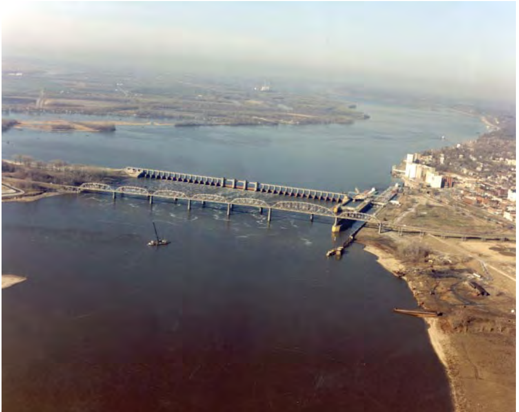
Aerial view of old L&D 26 just before beginning construction of Melvin Price Locks and Dam
