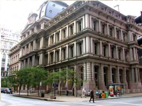
Old Post Office Building
