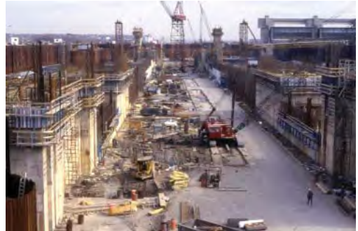
Second stage construction of main lock, November 1987
