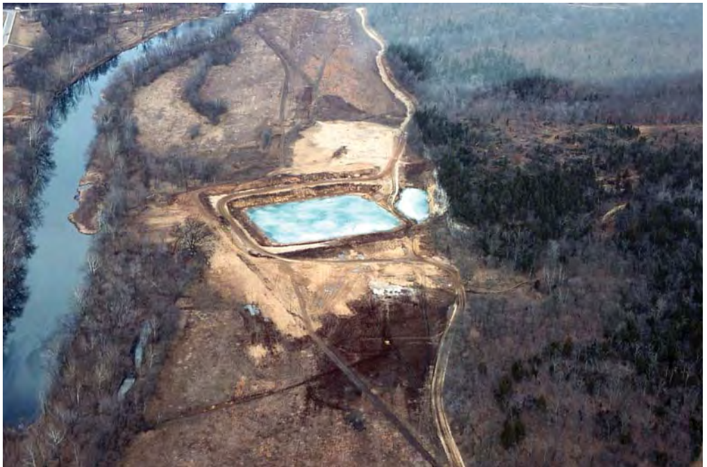
Aerial showing the site of Meramec Dam during early construction phase
