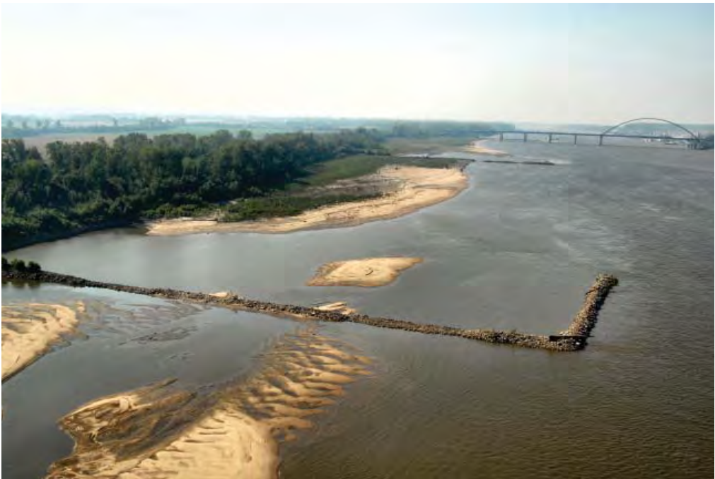
L-Dike north of St. Louis
