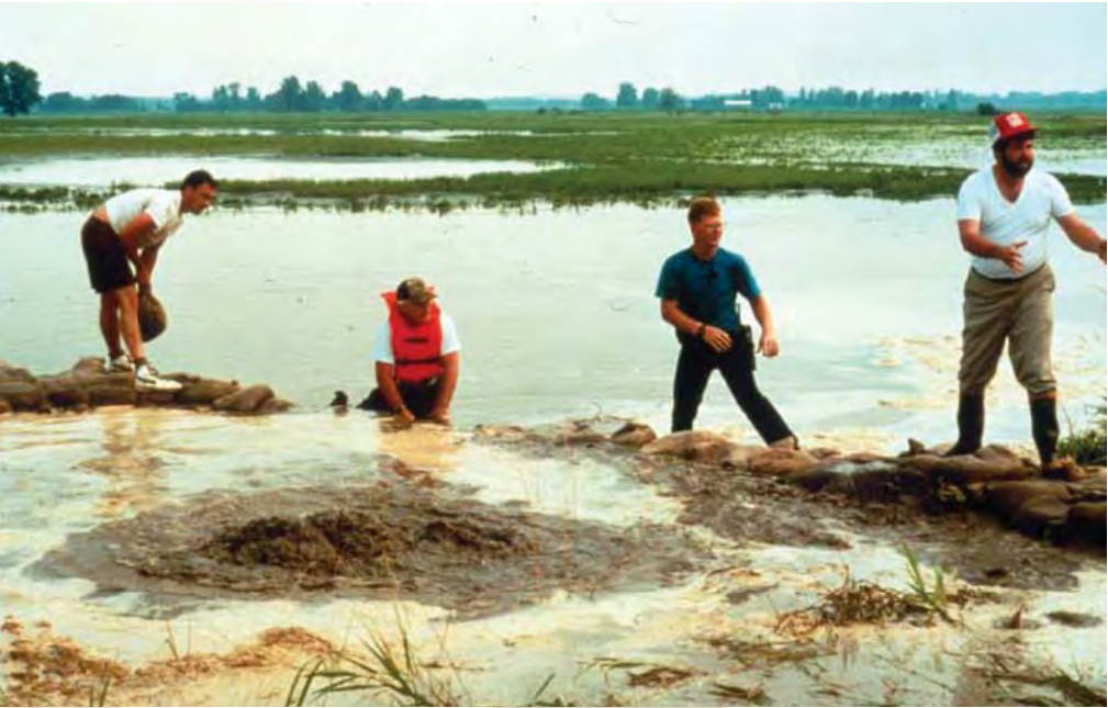
Mark Alvey, far right, and others ringing a sandboil on Kaskaskia Island
