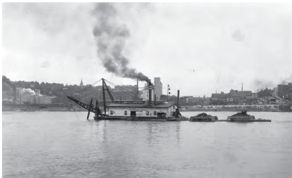
Dipper dredge St. Paul removing trailer dike near Lock and Dam No. 26
