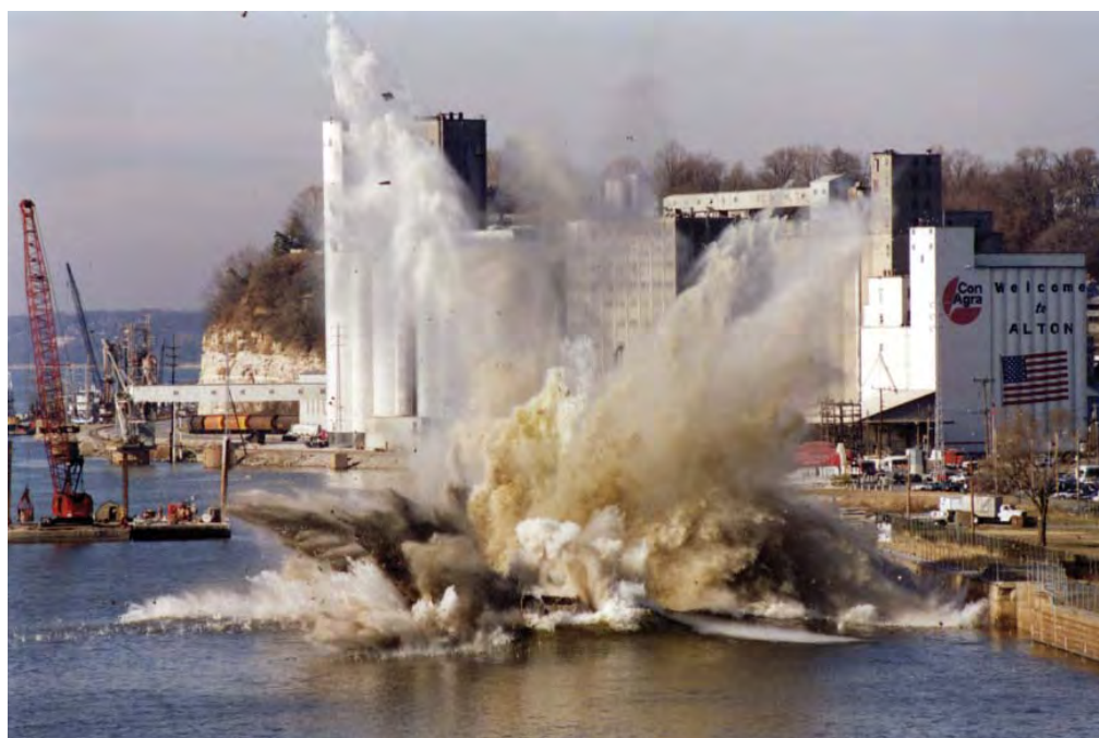
Last blast of old Lock and Dam 26
