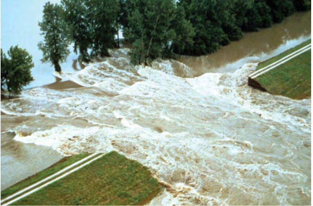
Levee overtopping during 1993 flood
