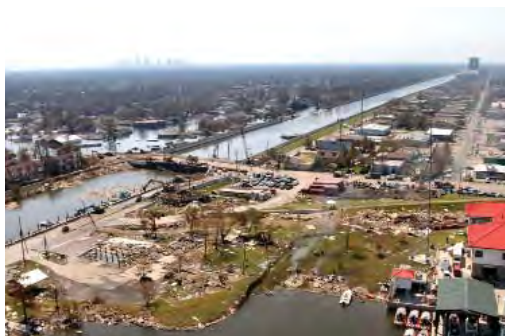
Aerial shot of 17th Street after Hurricane Katrina
