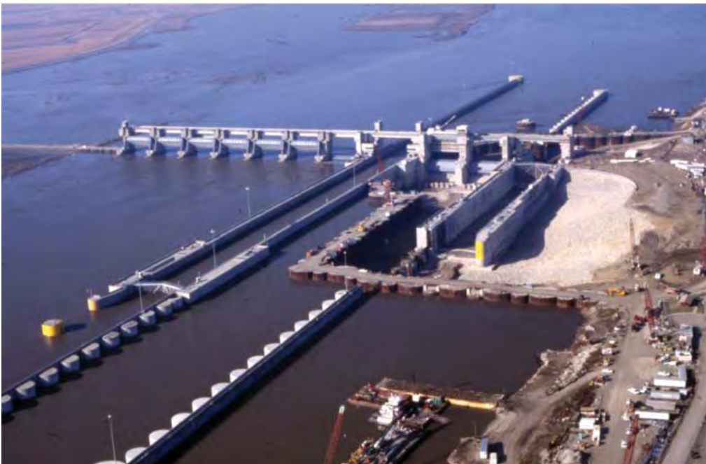
Third stage construction of auxiliary lock
