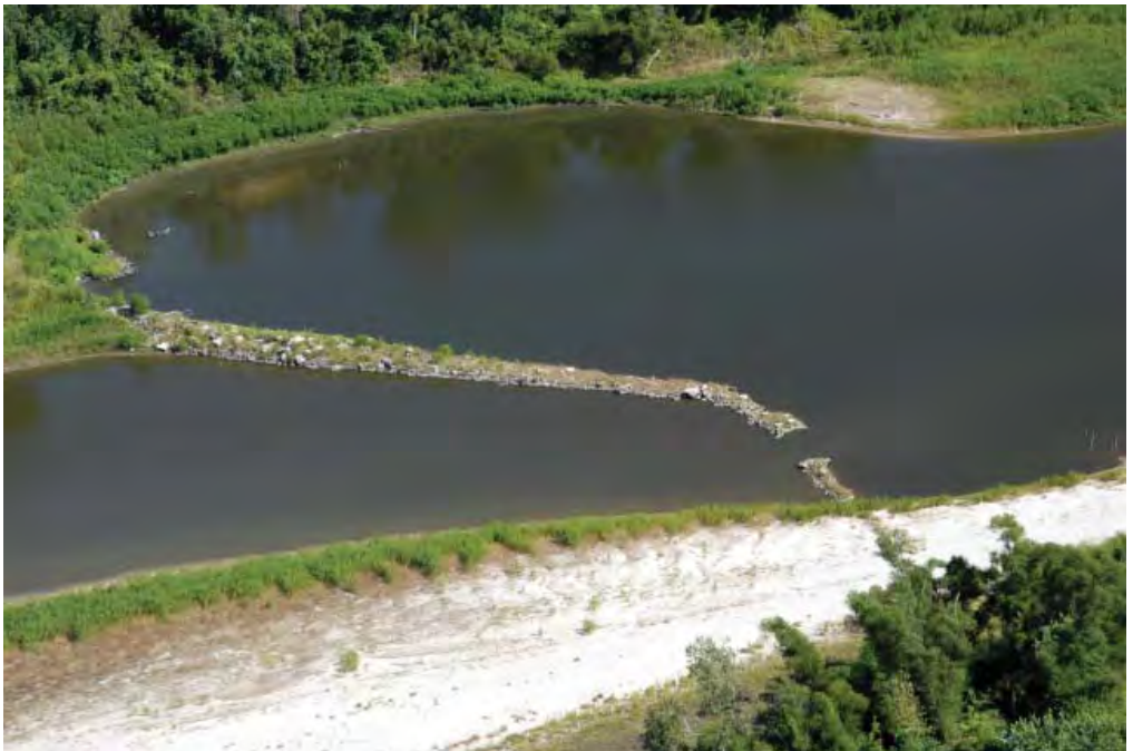
Notched closure structure
