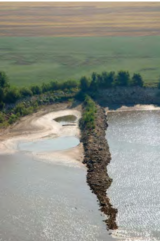
Dike using various sizes of rocks allowing for a greater diversity of habitats
