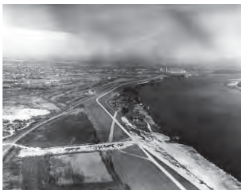
St. Louis Project, aerial view NE from Humboldt St. showing levee and Baden pumping station
