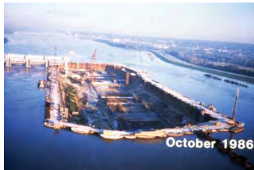
Second stage cofferdam during October 1986 flood
