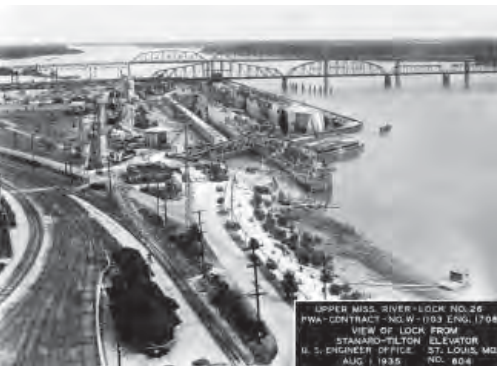
Lock and Dam 26 construction, 1935
