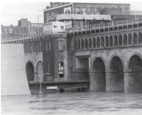
St. Louis floodwall just downstream of Eads Bridge during 1973 flood
