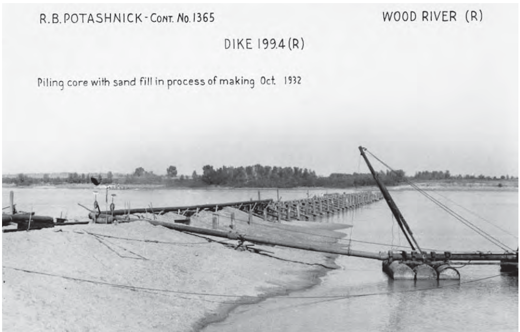
Early river training structure
