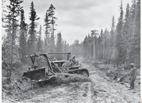
Construction of Alaska Highway, 1942
