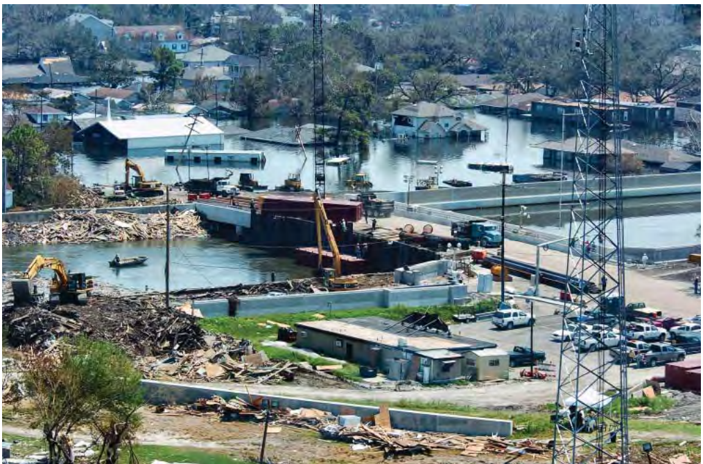
Construction of sheet piling on 17th Street
