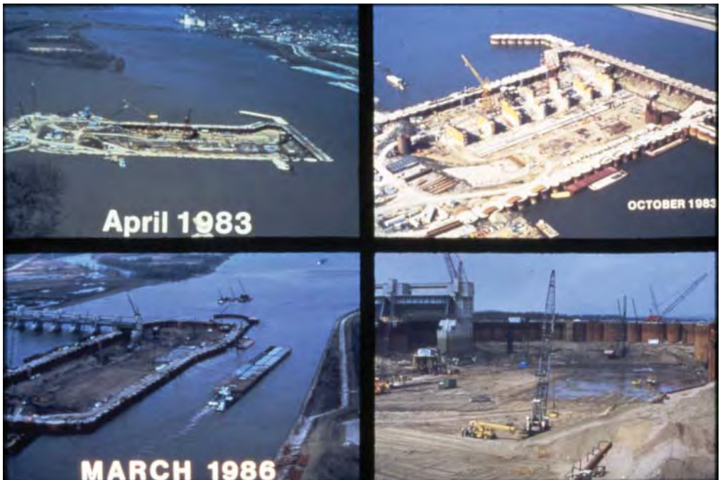
Construction stages at Lock and Dam 26R
