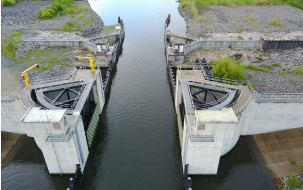
Figure B-20: Bayou Bienvenue and Bayou Dupre Sector Gates
