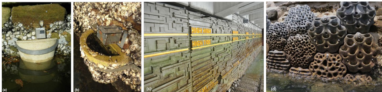
Figure 8. Examples of living seawall/vertical enhancements that could be installed on vertical shorelines. These could consist of pre-cast pots as shown in (a), (b), or (d) and pre-cast panels (c).
