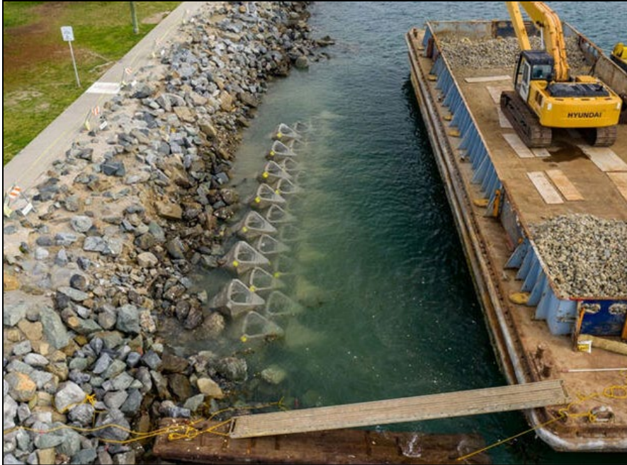
Figure 16. Example of ecological armoring from the EConcrete Coastalock Blue Economy Pilot Project in San Diego, CA.
