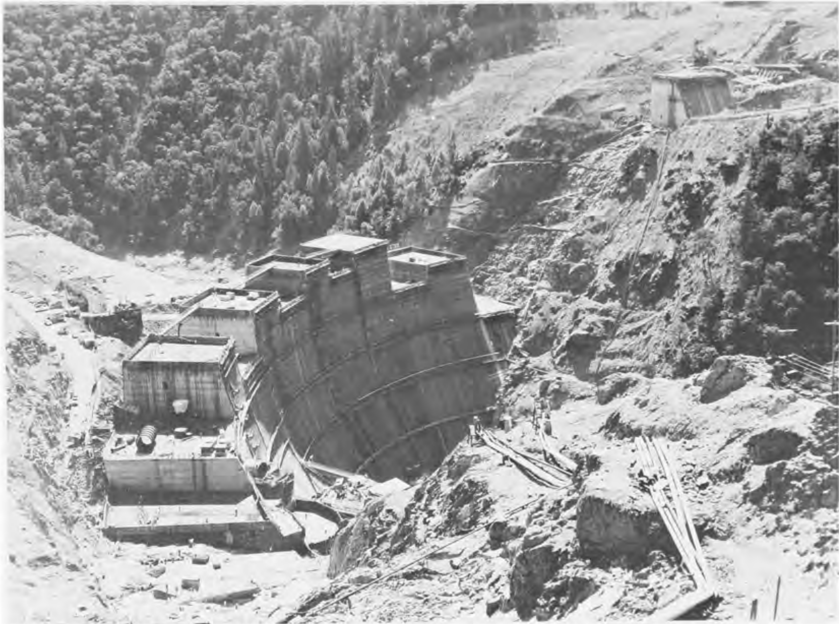
BULLARDS BAR DAM — 5 JUNE 1968 (Army Corps of Engineers Photo)
