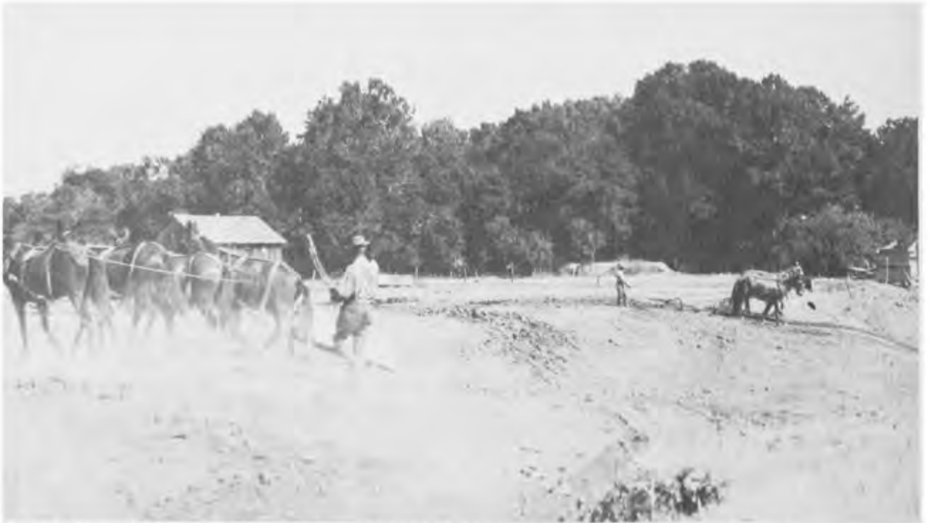
LEVEE CONSTRUCTION DURING THE EARLY DAYS, WITHIN THE SACRAMENTO DISTRICT, MEANT LONG DAYS AND A LOT OF MULE POWER. (National Archives Photos)
