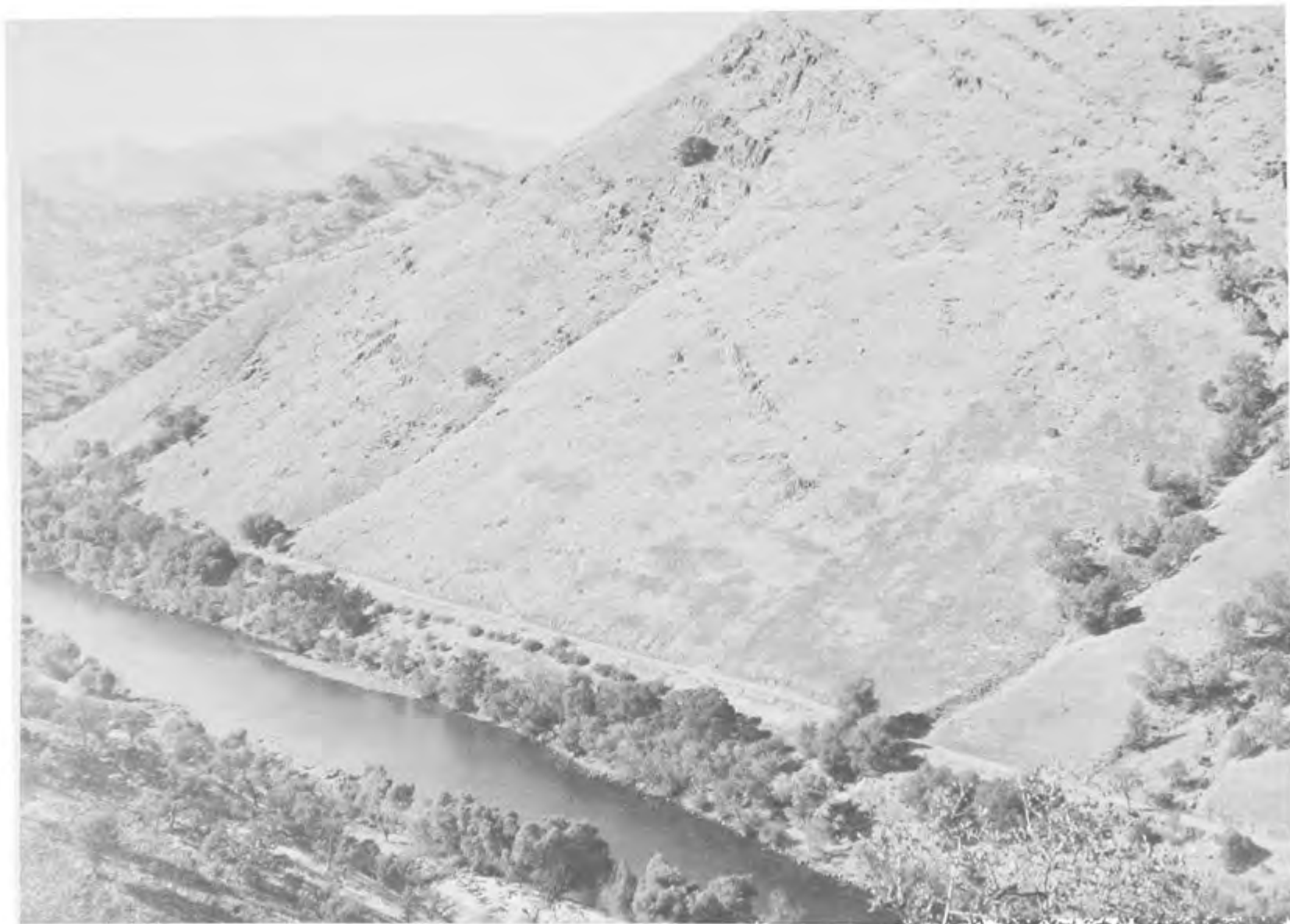
PINE FLAT: ONE OF THE LAST GREAT NATURAL DAM SITES ON THE SIERRA FRONT. THIS IS THE SITE OF THE DAM, ON THE KINGS RIVER, FRESNO COUNTY, PRIOR TO CONSTRUCTION.
