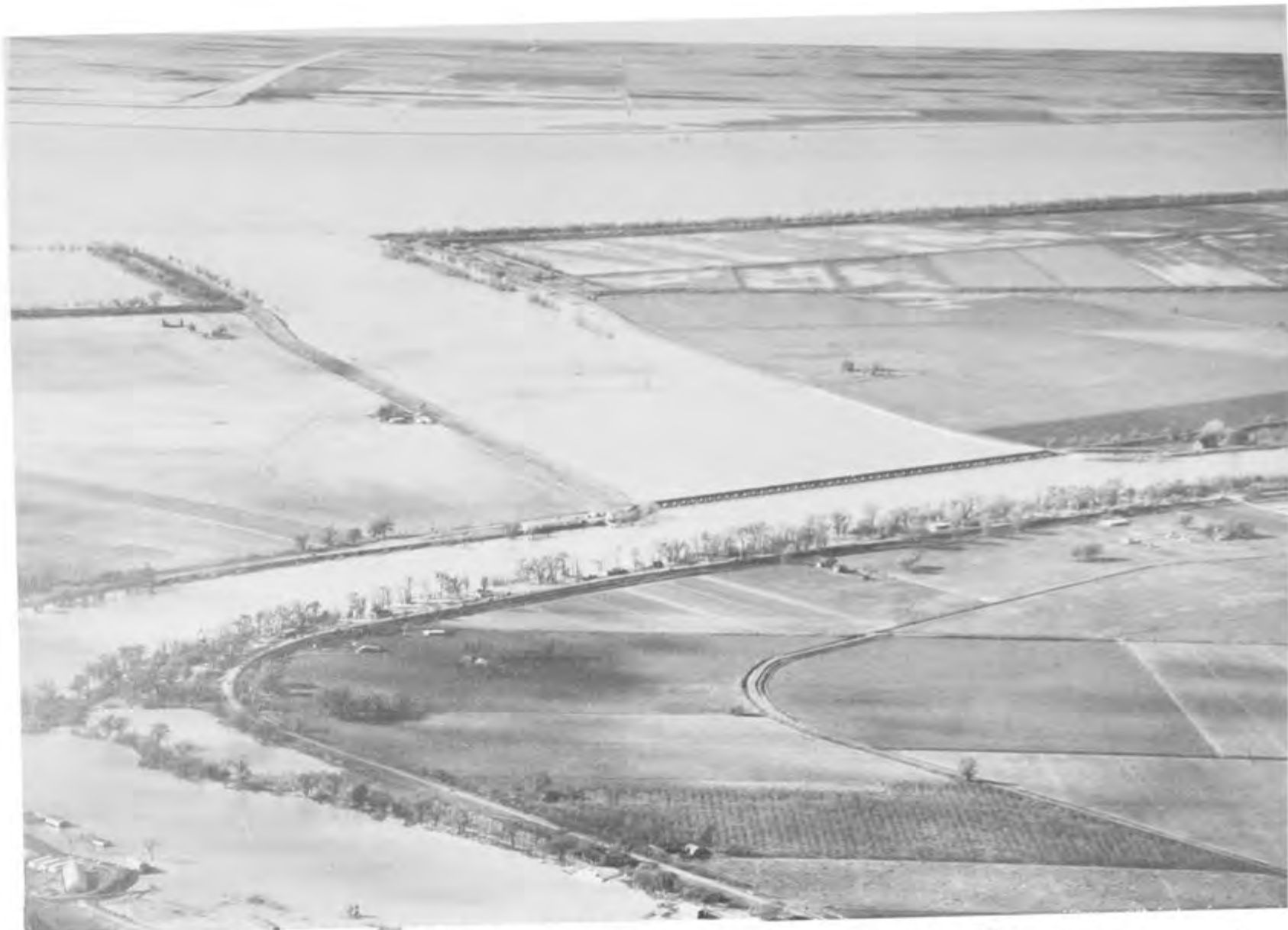
SACRAMENTO WEIR CONNECTING THE SWOLLEN SACRAMENTO RIVER WITH YOLO BYPASS — PHOTO TAKEN DECEMBER 1955. (Army Corps of Engineers Photo)
