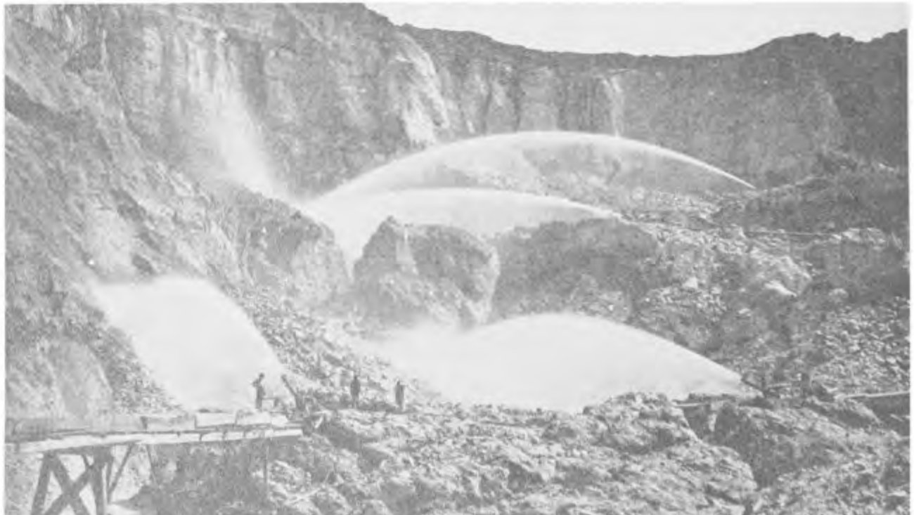
PHOTOS SHOWING EARLY HYDRAULIC MINING ACTIVITIES AT "MALAKOFF DIGGINGS" IN THE UPPER WATERSHED OF YUBA RIVER. THIS SITE IS NOW PART OF A 7,000-ACRE STATE PARK.
