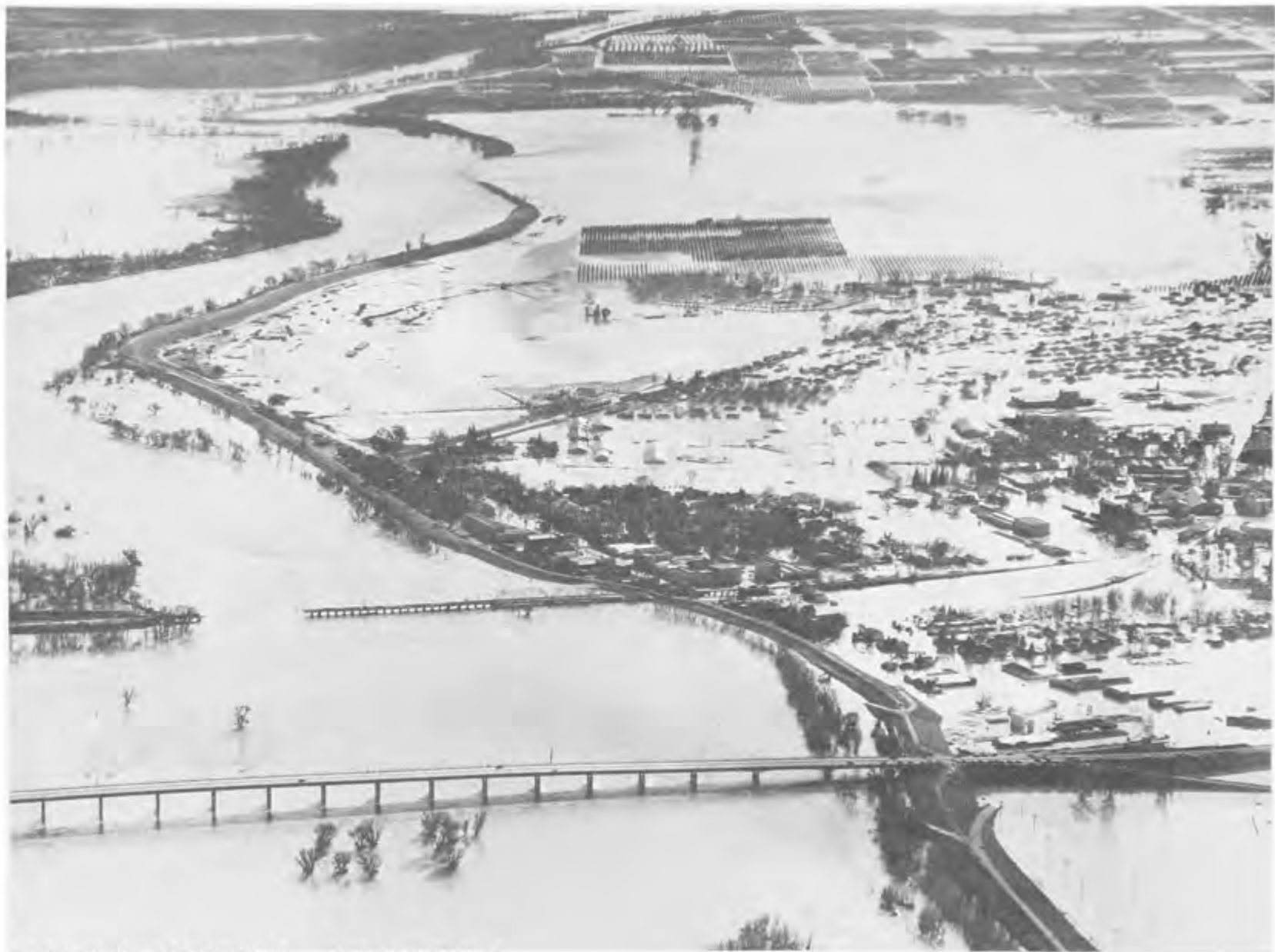
YUBA CITY, CALIFORNIA — DECEMBER 1955 (Army Corps of Engineers Photo)
