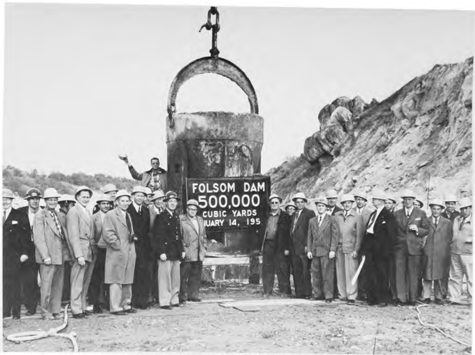
BY JANUARY 1954 THE HALF-WAY POINT HAD BEEN REACHED IN THE PLACING OF CONCRETE. DISTRICT PERSONNEL POSE FOR THE OCCASION.
