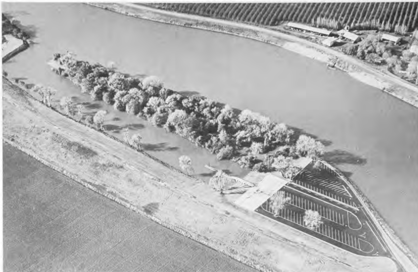
HOGBACK ISLAND AQUATIC PARK AND RECREATION SITE ON STEAMBOAT SLOUGH IN THE SACRAMENTO-SAN JOAQUIN DELTA. THE PROJECT FEATURES TWO BOAT LAUNCHING RAMPS, PARKING FACILITIES, A SANDY BEACH, TRAILS AND PICNIC AREAS. THE SACRAMENTO DISTRICT, U. S. ARMY CORPS OF ENGINEERS, CONVERTED THE ISLAND FROM ITS FORMER WILD STATE AS PART OF AN ADJACENT BANK PROTECTION PROJECT. THE PARK, WHICH TOOK EIGHTEEN MONTHS TO COMPLETE, HAS BEEN TURNED OVER TO THE STATE RECLAMATION BOARD FOR OPERATION AND MAINTENANCE.
