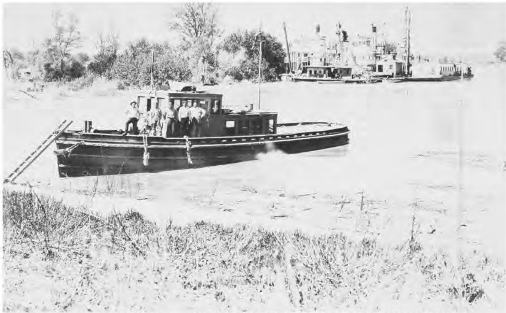
STOCKTON CHANNEL — APRIL 12, 1926 — DREDGE TENDER FALL , FOREGROUND. SNAG BOATS YUBA AND BEAR ALONGSIDE A PILE DRIVER, BACKGROUND. NOTE HOUSEBOATS ALONGSIDE; THIS IS WHERE THE CREWS LIVED.
