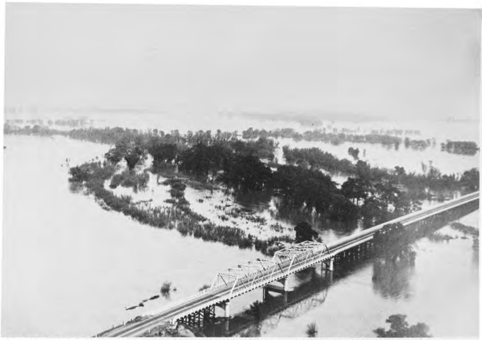
MAZE ROAD BRIDGE OVER SAN JOAQUIN RIVER BETWEEN TUOLUMNE AND STANISLAUS RIVERS. VIEW LOOKING NORTHEAST. DECEMBER — 1950.
