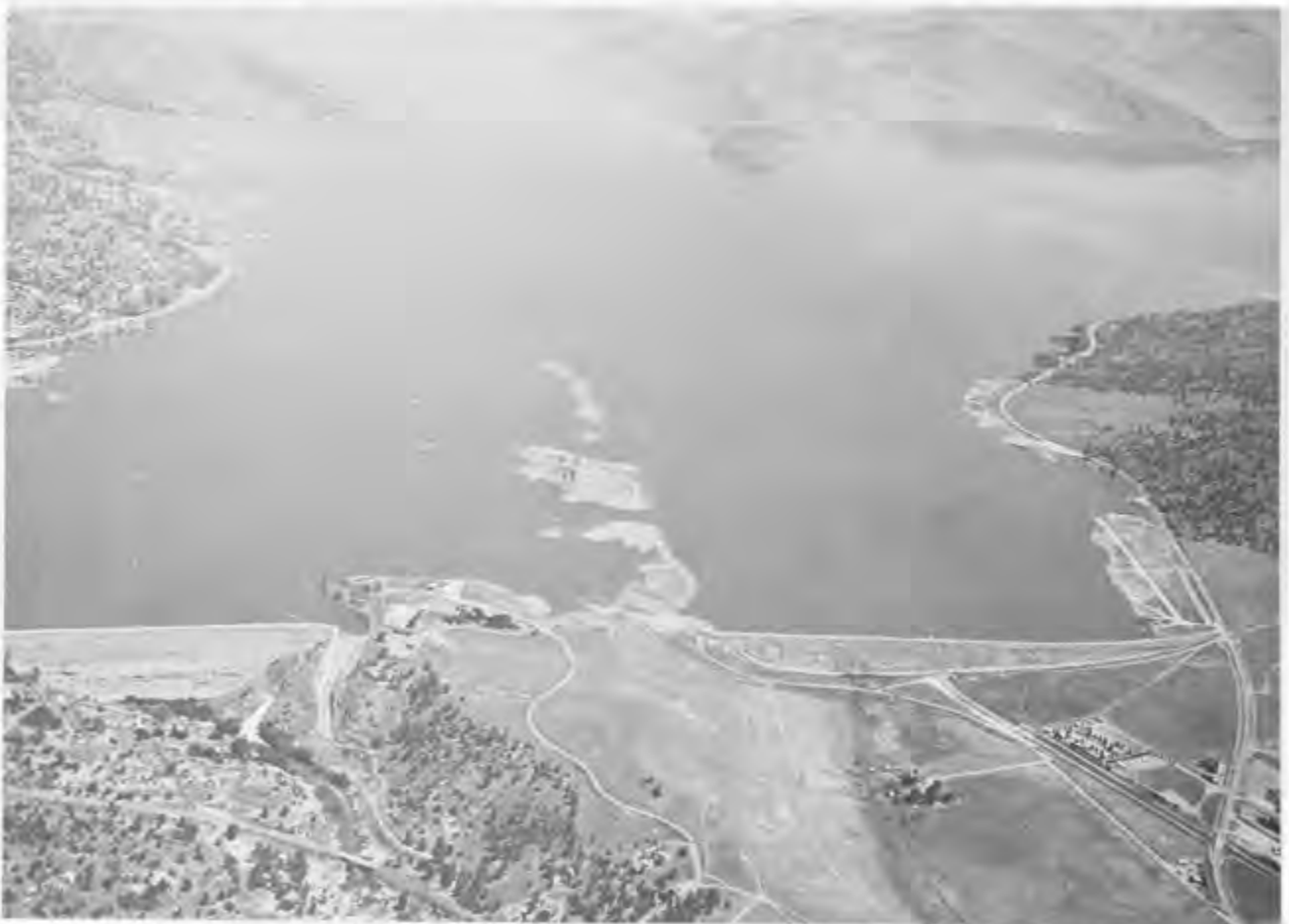
ISABELLA DAM BACKS UP A HUGE RESERVOIR OF WATER NEAR BAKERSFIELD, CALIFORNIA. THIS SACRAMENTO DISTRICT, CORPS OF ENGINEERS, DAM AND RESERVOIR OFFERS A VARIETY OF RECREATION ACTIVITIES SUCH AS BOATING, HUNTING, FISHING, SWIMMING, PICNICKING AND HIKING.
