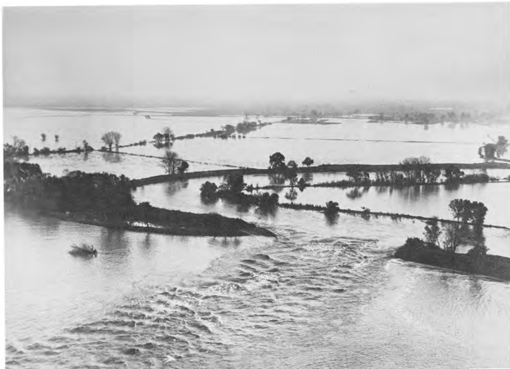
BREAK IN EAST LEVEE OF SAN JOAQUIN RIVER BELOW MOSSDALE. FLOODING OF RECLAMATION DISTRICT NO. 17 — DECEMBER 1950.
