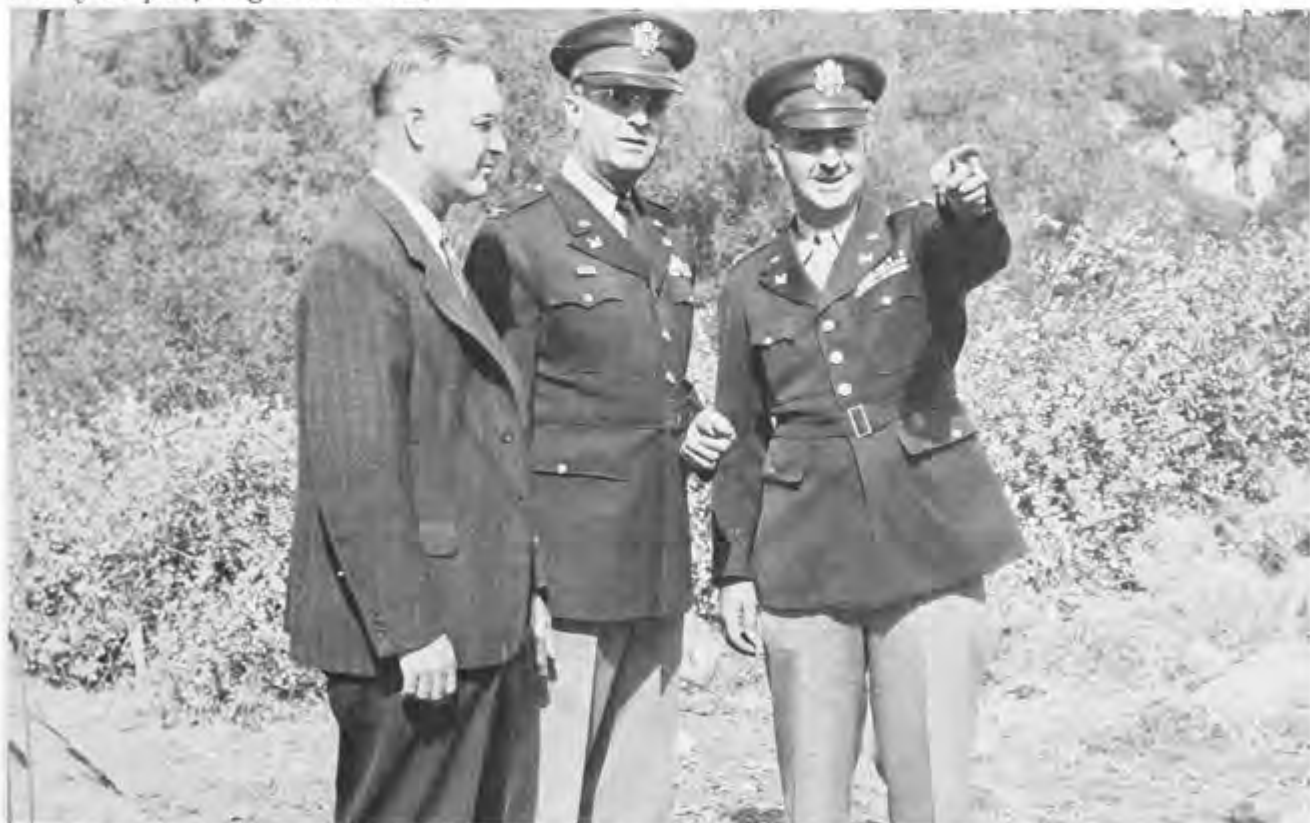
INSPECTING FOLSOM DAM SITE — 1948. LEFT TO RIGHT — JAMES L. ROSE, RESIDENT ENGINEER; COLONEL DWIGHT F. JOHN, SOUTH PACIFIC DIVISION ENGINEER; COLONEL JOSEPH S. GORLINSKI, SACRAMENTO DISTRICT ENGINEER.
