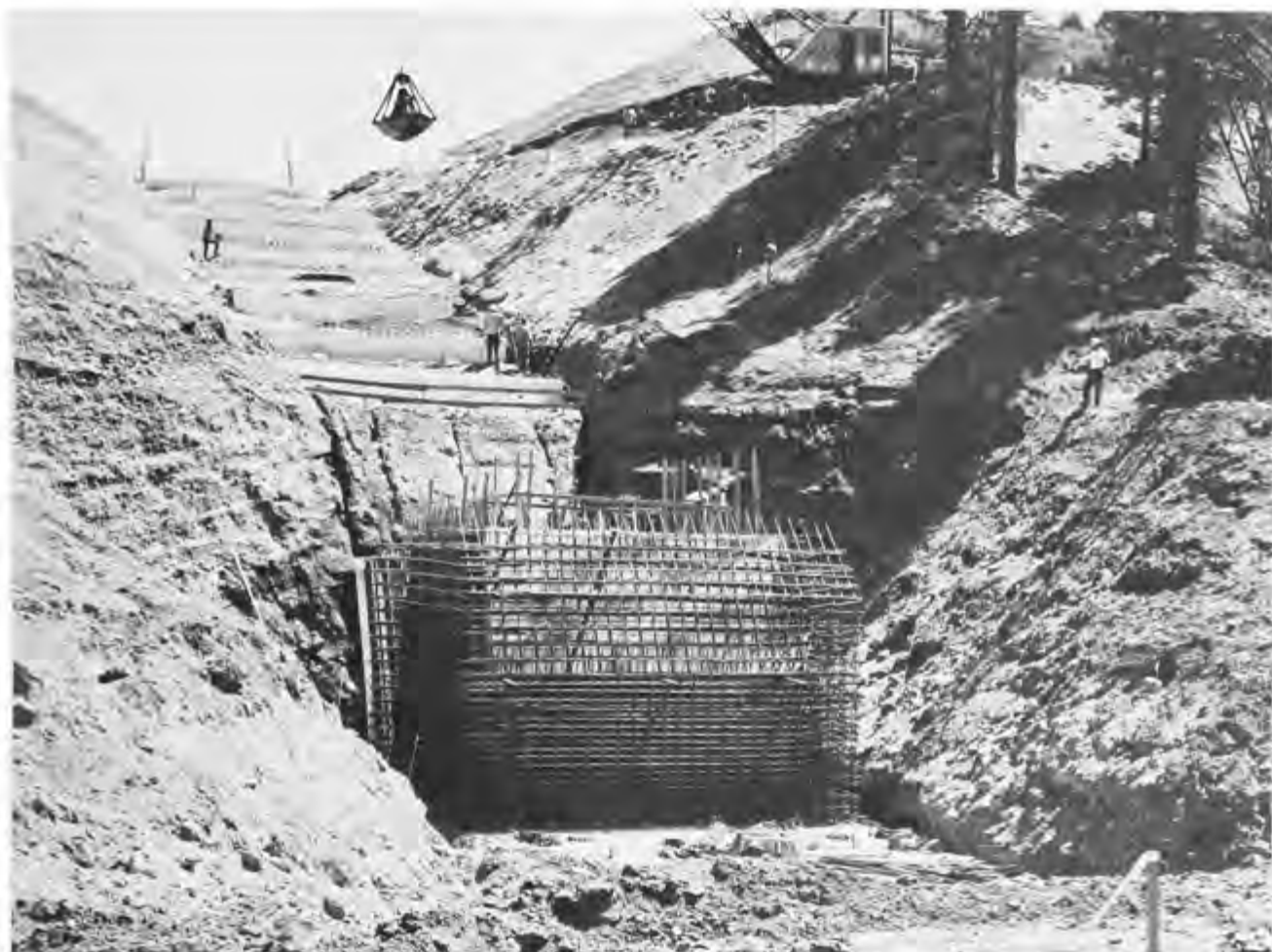
THE SPILLWAY OF THE MARTIS CREEK DAM, UNDER CONSTRUCTION BY THE PERINI CORPORATION FOR THE SACRAMENTO DISTRICT, CORPS OF ENGINEERS. PHOTO TAKE 26 AUGUST 1970.
