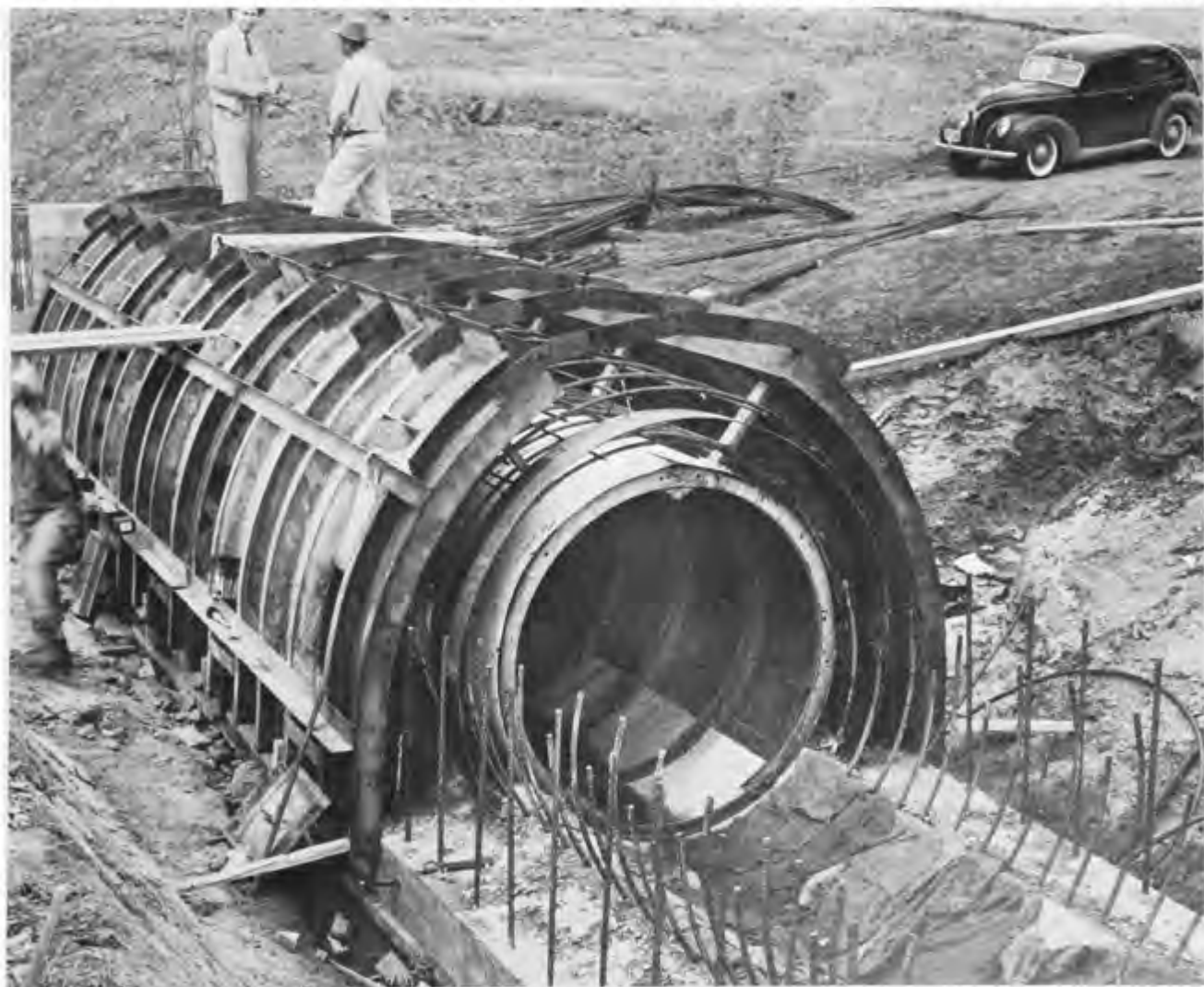
OUTLET WORKS — MARIPOSA DAM.
