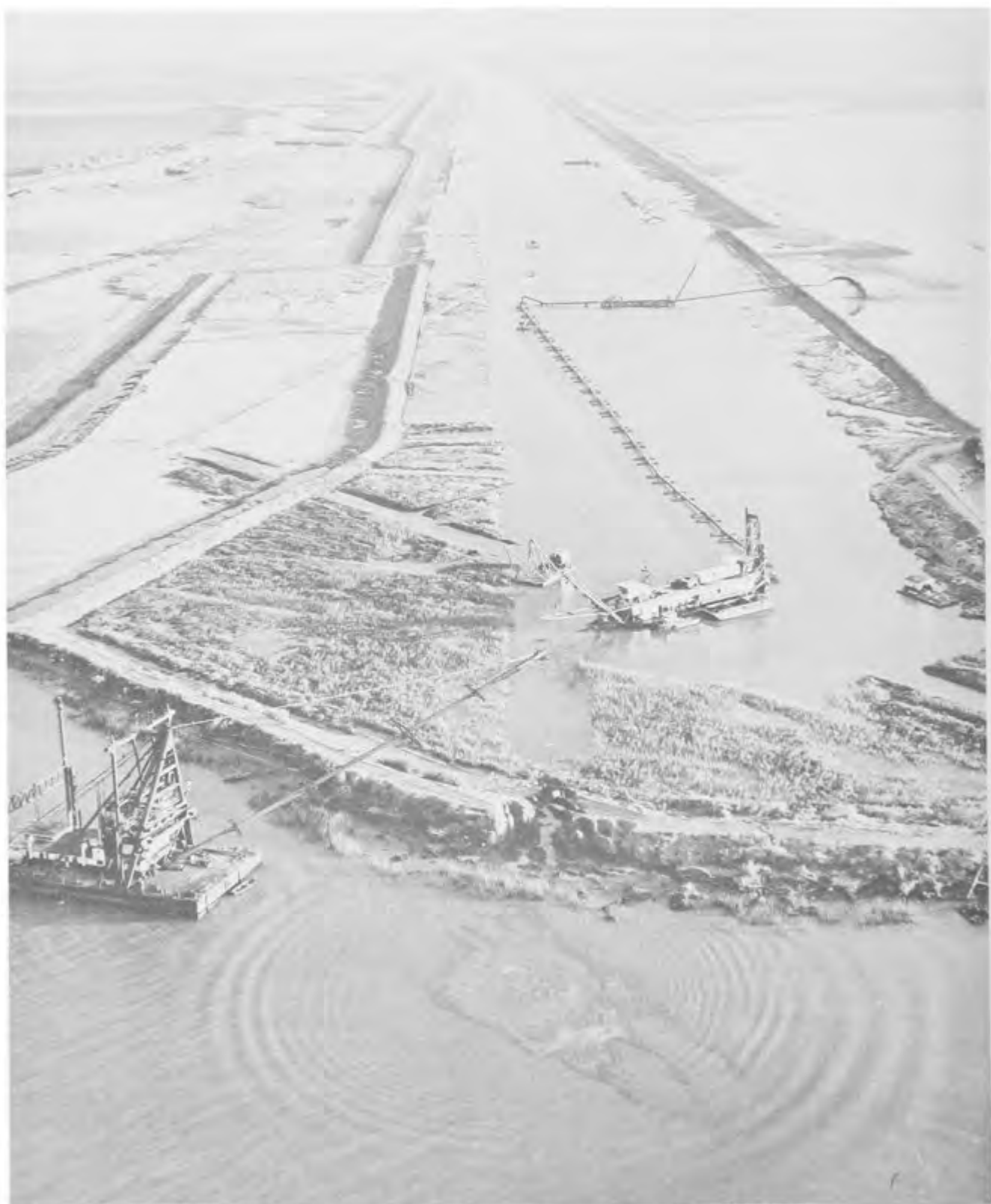
SACRAMENTO DEEP WATER CHANNEL UNDER CONSTRUCTION. (Ca 1961) (Sacramento Bee Photo)
