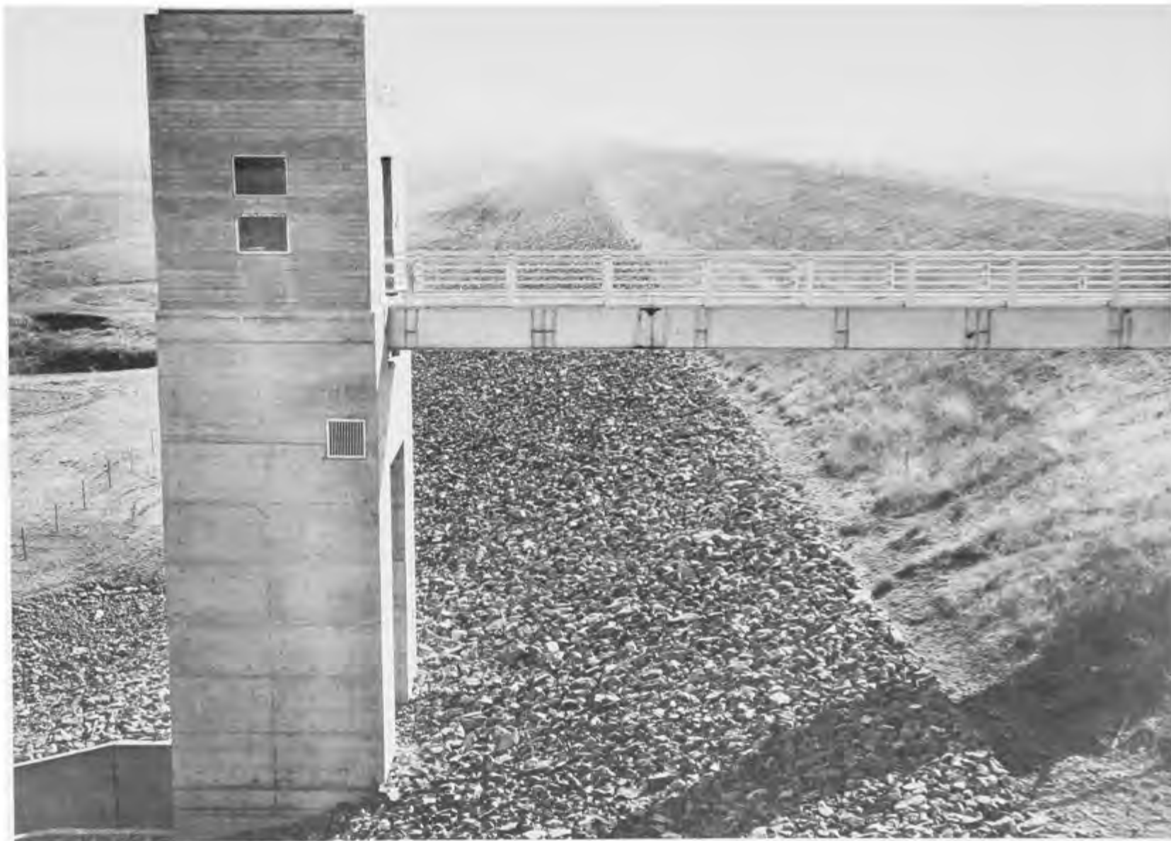
FARMINGTON DAM PROJECT NEAR FARMINGTON, CALIFORNIA. COMPLETION PHOTO — VIEW LOOKING SOUTHERLY FROM RIGHT ABUTMENT SHOWING RIP-RAPPING FOR SLOPE PROTECTION. (Army Corps of Engineers Photo)
