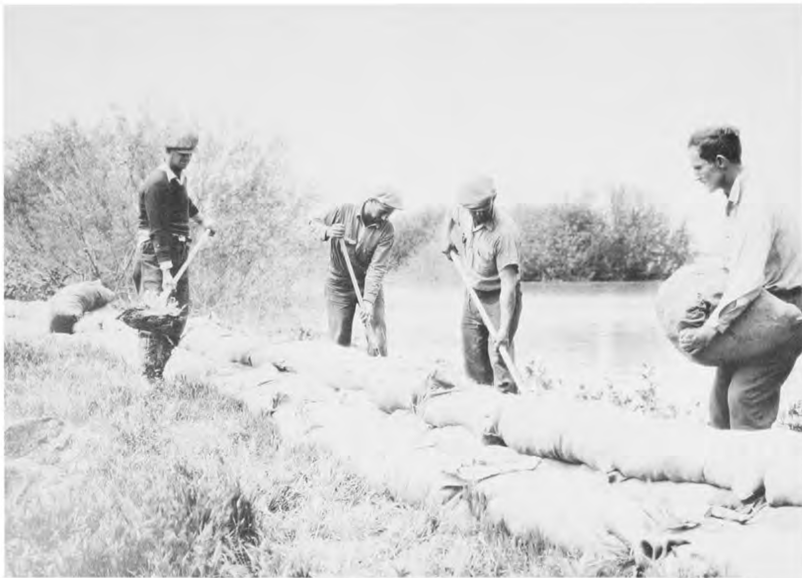
MEN WORKED HARD AND LONG DURING THE THIRTIES TO REINFORCE LEVEES ALONG THE SACRAMENTO AND SAN JOAQUIN RIVERS.
