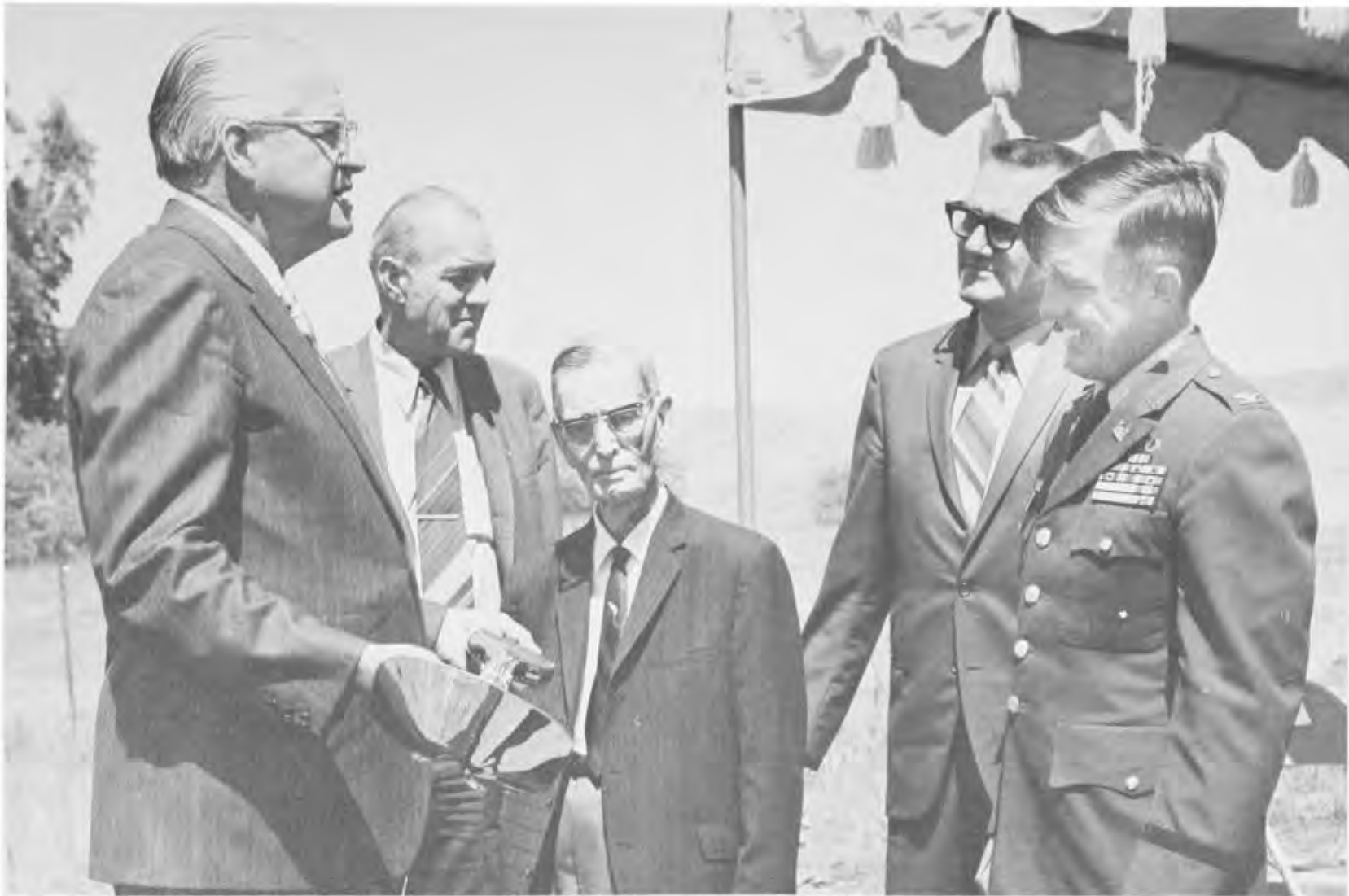
U.S. CONGRESSMAN HAROLD T. (BIZZ) JOHNSON (L.) HAS JUST ACCEPTED A CROME-PLATED AND INSCRIBED SHOVEL SYMBOLIC OF THE CONSTRUCTION START OF THE BUCHANAN DAM FROM COLONEL JAMES C. DONOVAN, ARMY CORPS OF ENGINEERS. LOOKING ON (L. TO R.) ARE: MADERA COUNTY SUPERVISOR HAROLD J. BALMAT; JUDGE H.V. EASTMAN, SECRETARY-MANAGER, CHOWCHILLA WATER DISTRICT; AND CHOWCHILLA MAYOR SAMUEL L. McCLAUGHRY.
