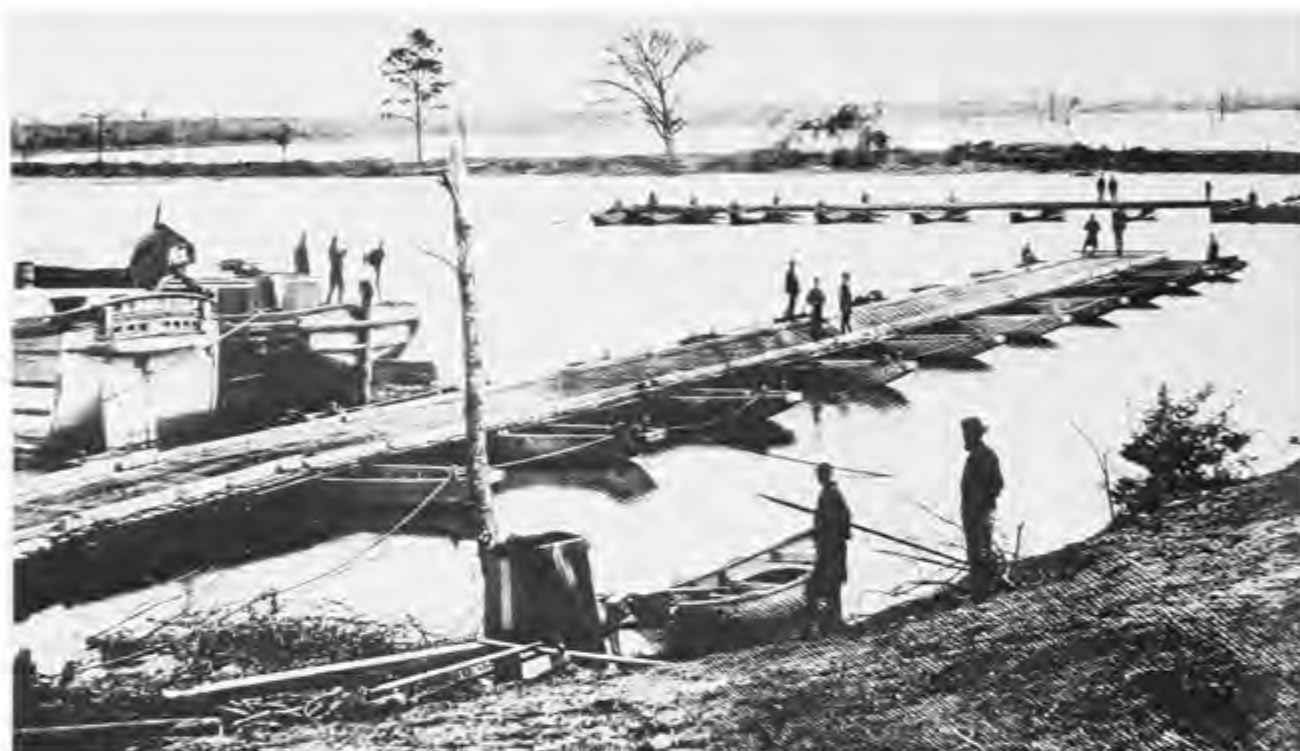
ARMY ENGINEERS CONSTRUCT PONTOON BRIDGE ACROSS JAMES RIVER, VIRGINIA, DURING CIVIL WAR PERIOD.
