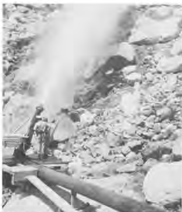
POWERFUL "WATER CANNONS" SUCH AS THIS RIPPED THE MOUNTAINS APART, AND SENT DEBRIS INTO THE RIVERS.
