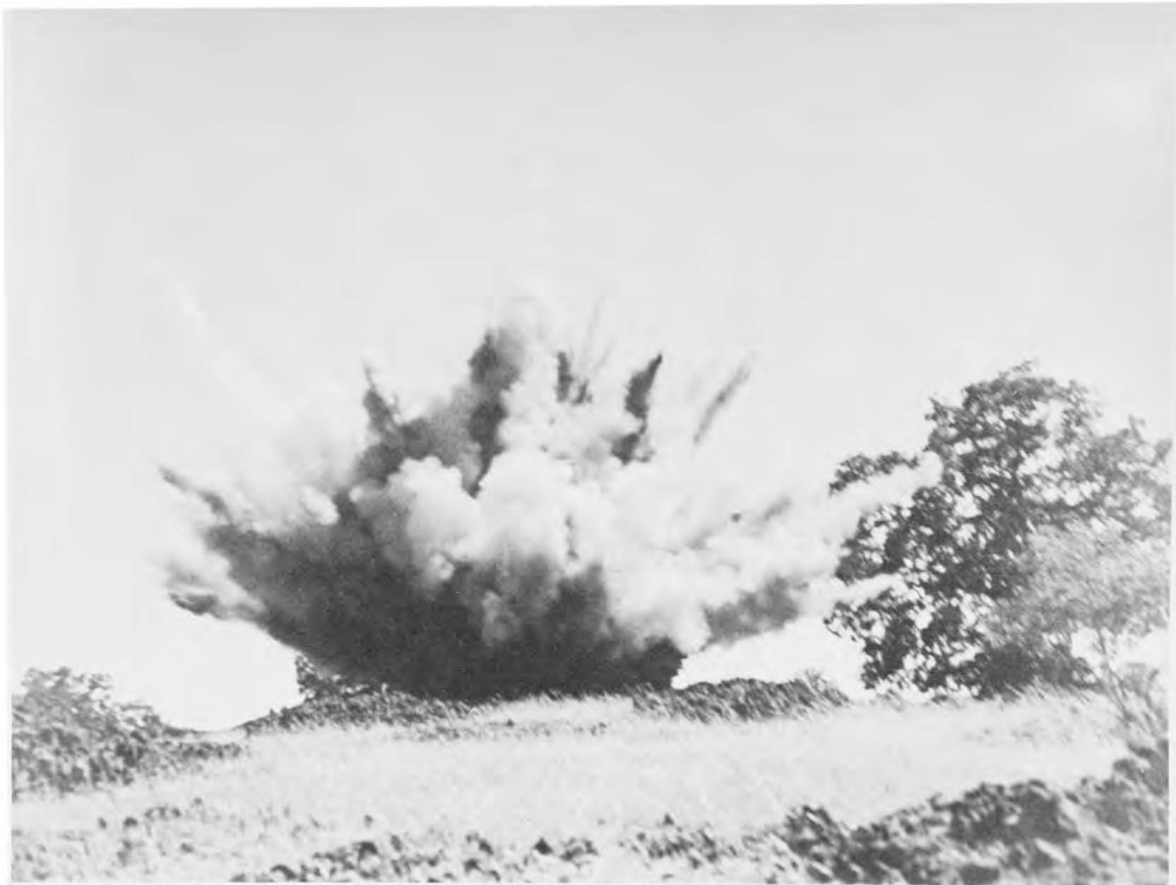
GROUND BREAKING AT BLACK BUTTE DAM SITE — JUNE 4, 1960.
