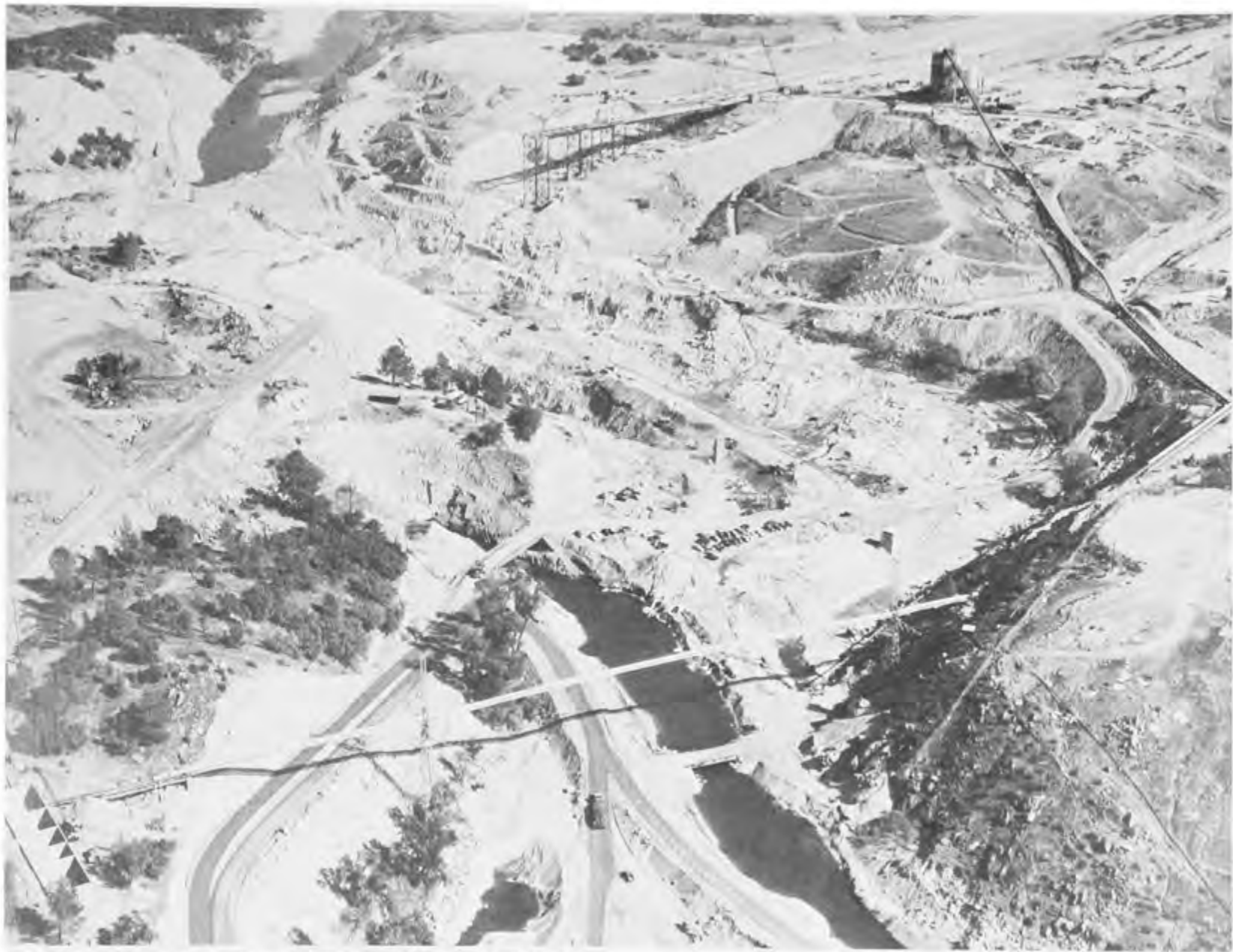
FOLSOM DAM SITE FOUNDATION EXCAVATION WORK.
