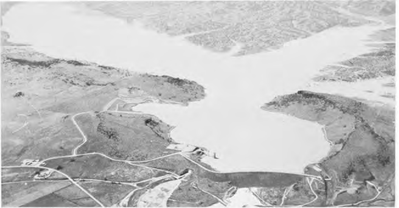
BLACK BUTTE DAM AND LAKE (Army Corps of Engineers Photo)
