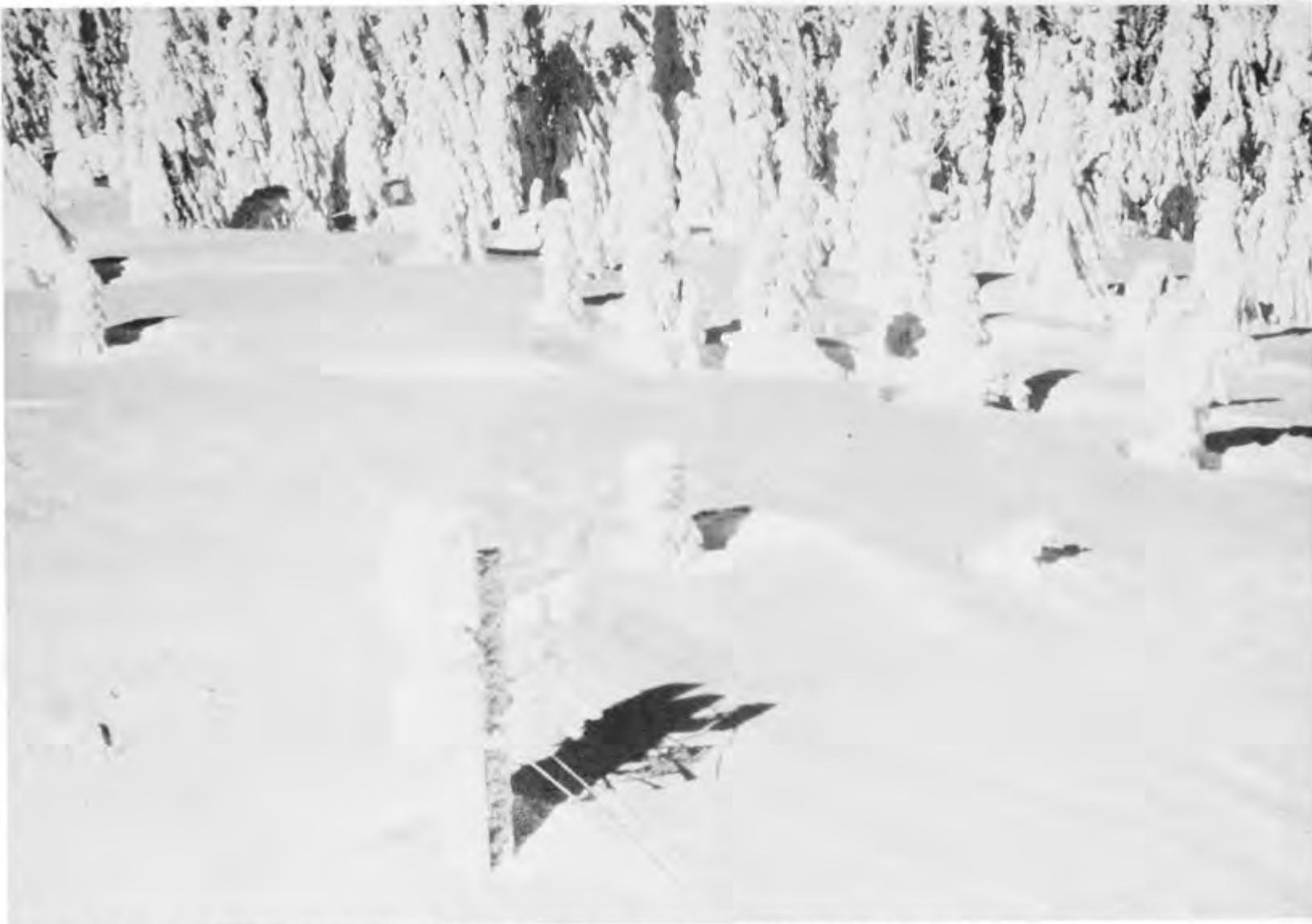
THE SHERMAN MOUNTAIN RADIO RELAY ANTENNA IN THE KERN RIVER BASIN 30 MILES SOUTHWEST OF MOUNT WHITNEY. ELEVATION HERE IS 10,000 FEET. THIS ANTENNA RELAYS SNOW WATER CONTENT INFORMATION GATHERED FROM SNOW PILLOWS TO THE ISABELLA DAM RECEIVING STATION.
