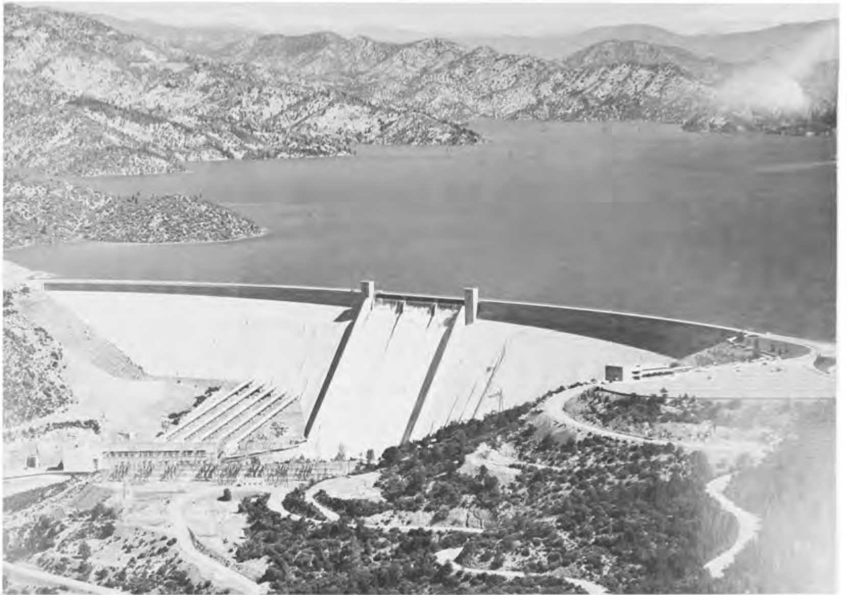
SHASTA DAM, KEY UNIT OF THE CENTRAL VALLEY PROJECT. (Bureau of Reclamation Photo)
