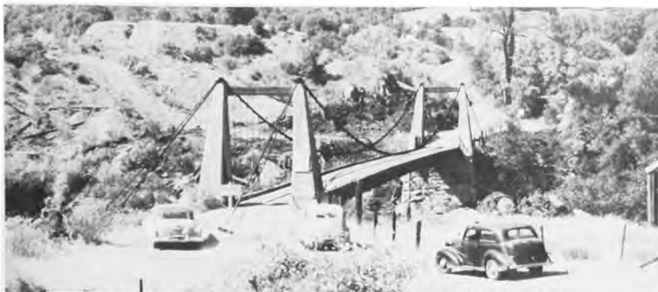
OLD BRIDGE ACROSS THE AMERICAN RIVER NEAR THE SITE OF FOLSOM DAM. (Army Corps of Engineers Photo)
