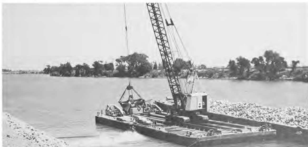
BANK PROTECTION PROJECT — SACRAMENTO RIVER (Army Corps of Engineers Photo)
