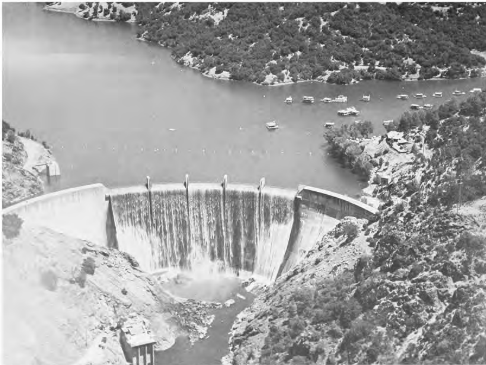
HARRY L. ENGLEBRIGHT DAM ON THE YUBA RIVER. (Ca 1969) (Army Corps of Engineers Photo)
