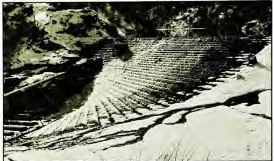
Wire basket cobbles-filled dam in Scotchman Creek for restraining tailings resulting from hydraulic mining at Omega Mine near Washington, Nevada County, Calif.
