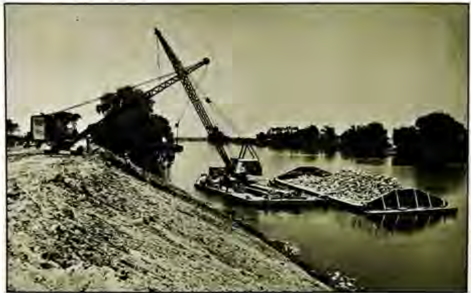
Sacramento River, bank protection work. (Corps of Engineers' photo)
