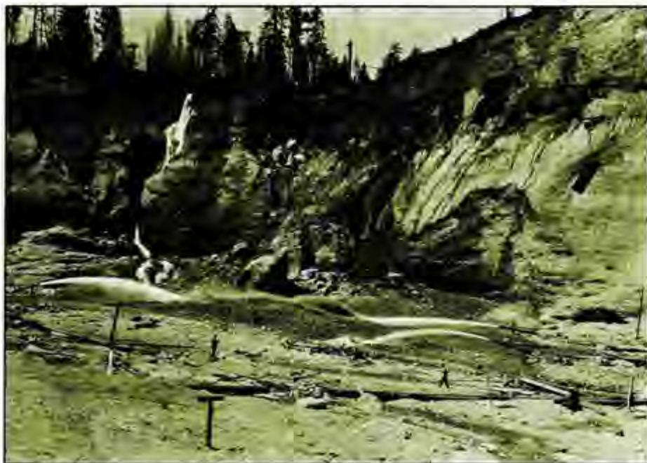
Brandy City Mine, Sierra County, showing three monitors in operation. (Corps of Engineers' photo)
