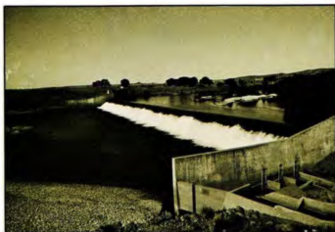
Daguerre Point Dam, 1980. (Author's photos)
