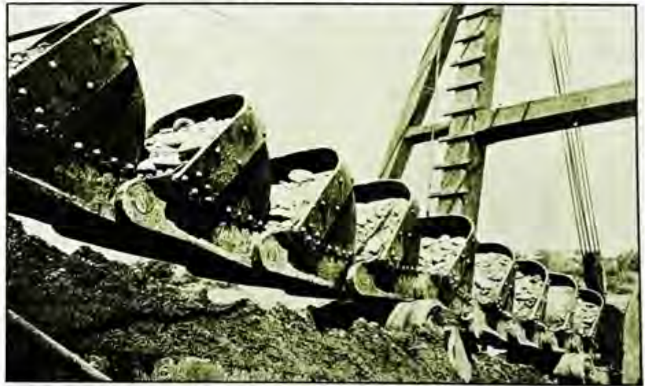
Bucket ladder of gold dredge in operation.
