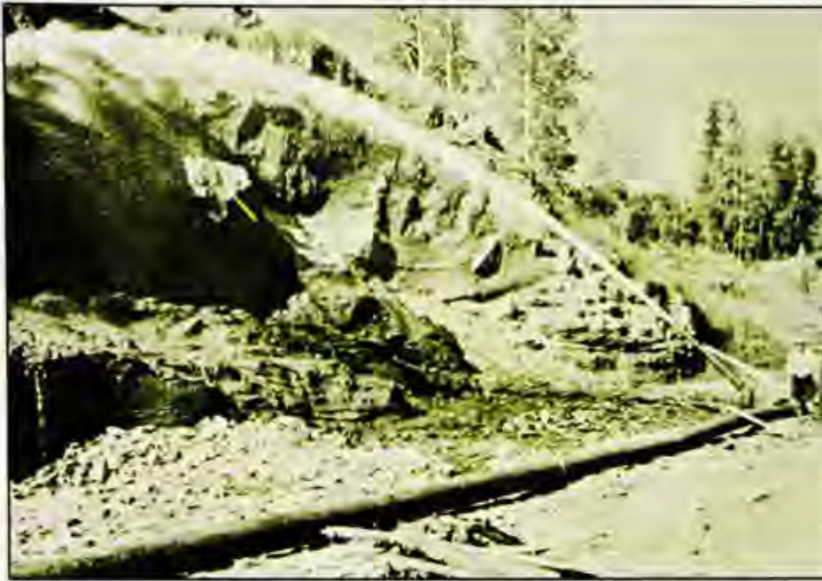
The early-day photo shows the terrible power of even a relatively small hydraulic appliance. (Corps of Engineers photo)
