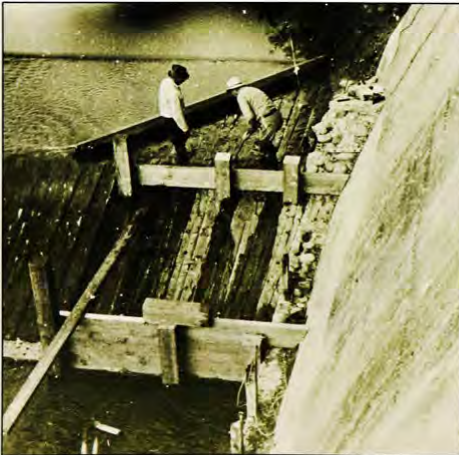
Prior to World War II, the CDC completed work on the fish ladders at Daguerre Point Dam. (Corps of Engineers' photos)
