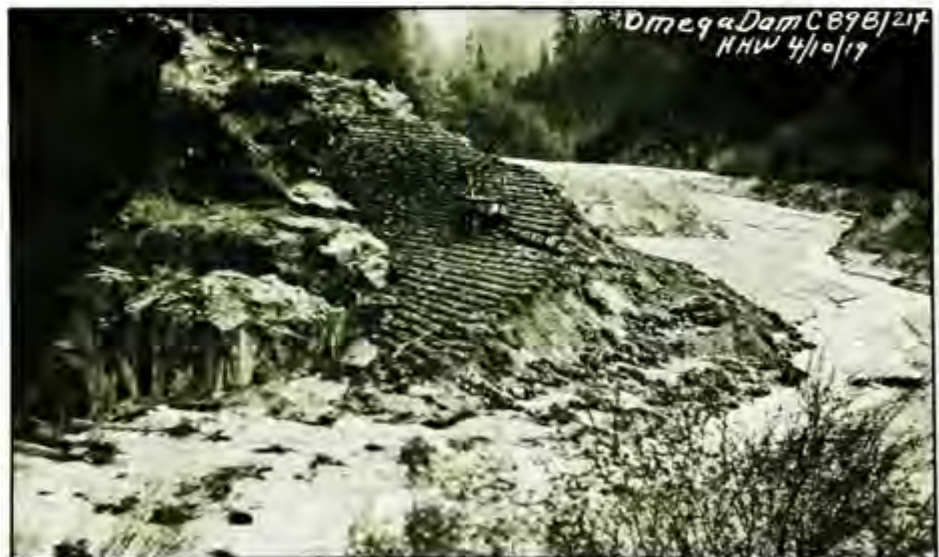
View taken April 10, 1919, after failure of above dam.
