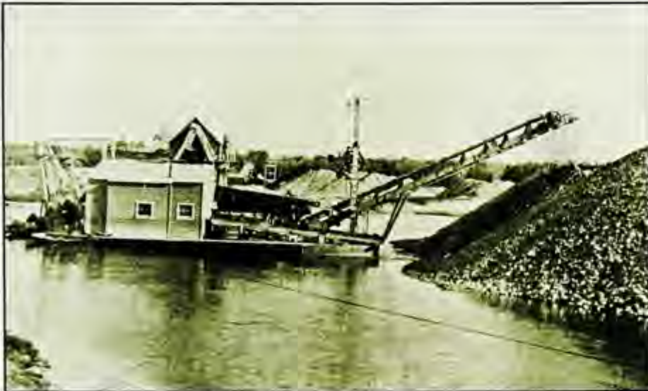
Risdon gold dredge working inland, Oroville District.
