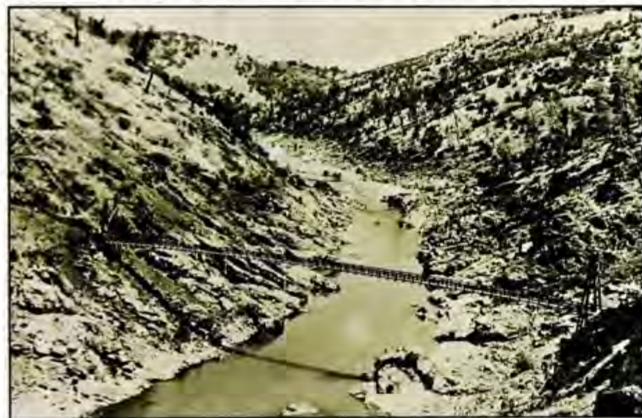
Upper Narrows Dam Site, Yuba River, July 20, 1937. (Corps of Engineers' photo)
