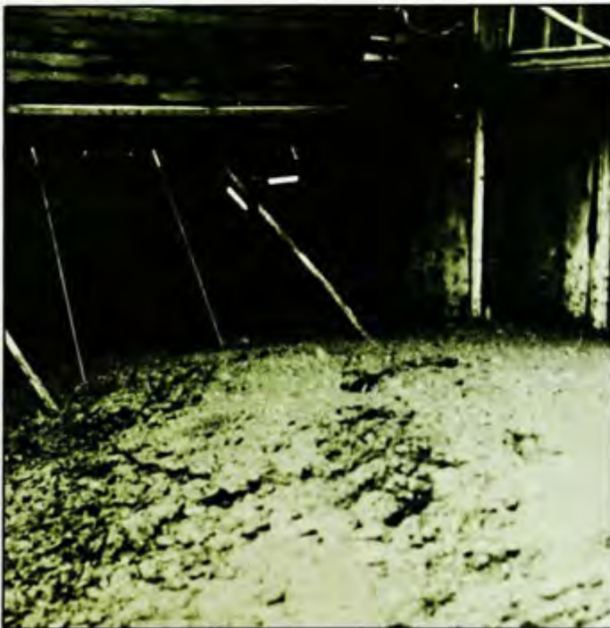
Strain meter installation with pipe supports partially covered with concrete (10/28/38).
