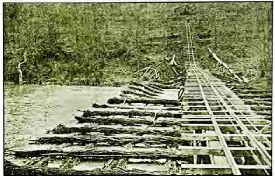
Barrier No. 2, Yuba River, Cal., October 3, 1903. Showing construction of brush fascine pockets under contract with Samuel Montgomery, dated August 17, 1903.
