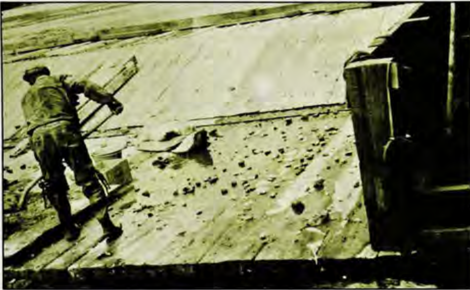
Workman above repairs planking on Daguerre Point Dam during the 1930s. (Corps of Engineers' photo)
