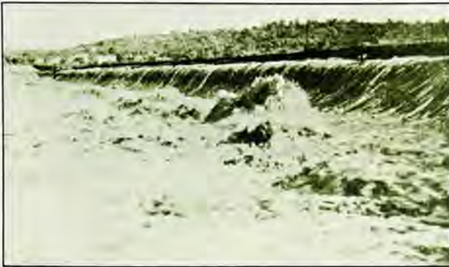
Barrier No. 1 — Yuba River, September 1901. High water passing over unfinished dam.
