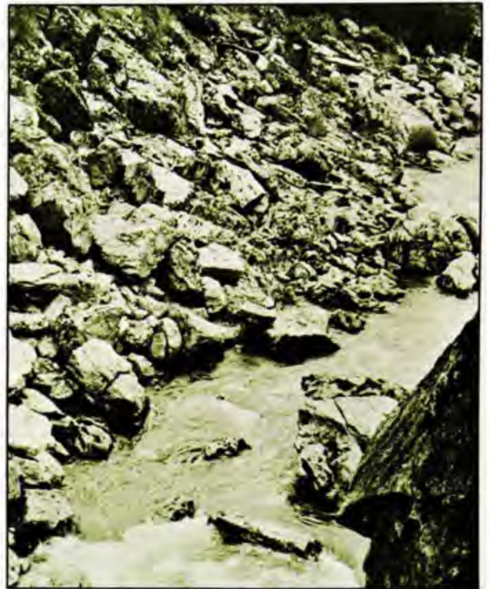
Ruck-a-Chucky dam site, 1933. (Corps of Engineers' photo)
