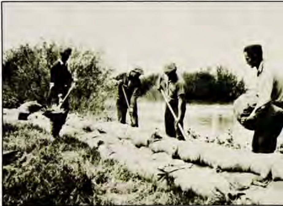
Men worked hard and long during the thirties to reinforce levees along the Sacramento and San Joaquin Rivers. (Corps of Engineers' photos)
