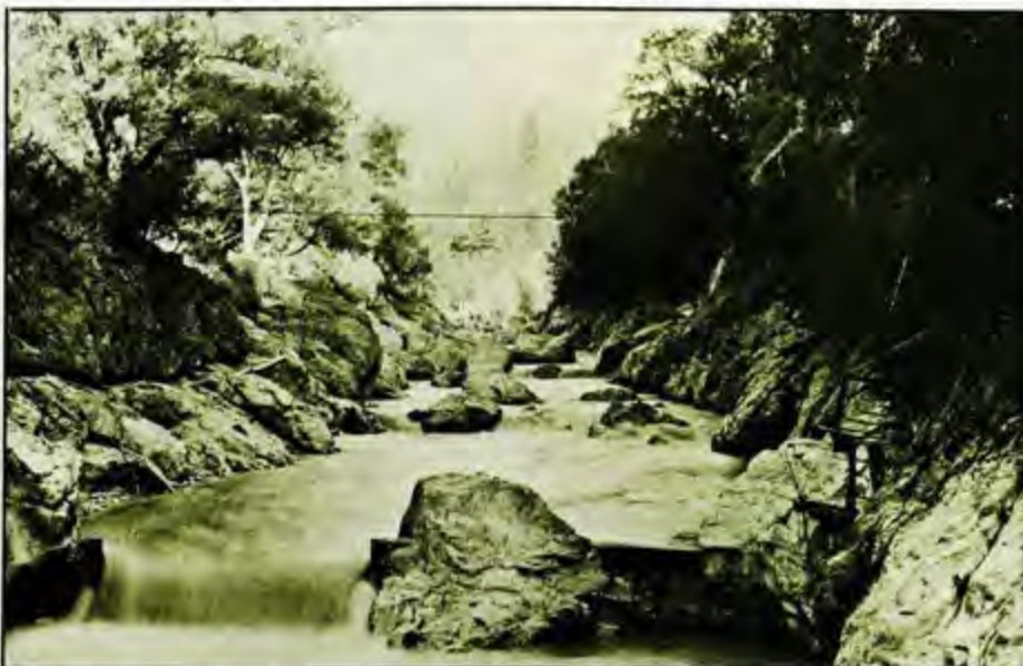
Proposed dam site on the lower Bear river, 1934. (Corps of Engineers' photo)
