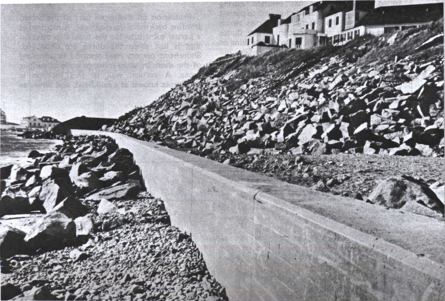
Figure 18. Vertical-face Concrete Seawall built 25 years ago at Watch Hill, Rhode Island. Seawall, combined with heavy rock riprap, protects the residence on hill at right. Photo from Portland Cement Association.
