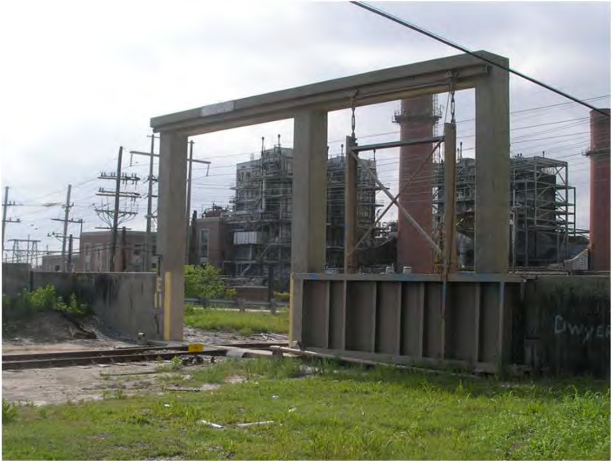
Figure F-7. Trolley Gate Closure Structure.
