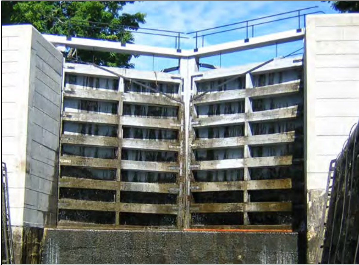
Figure B-1. Miter Gate.
