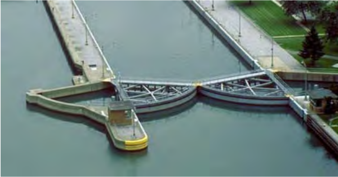
Figure B-3. Sector Gate.
