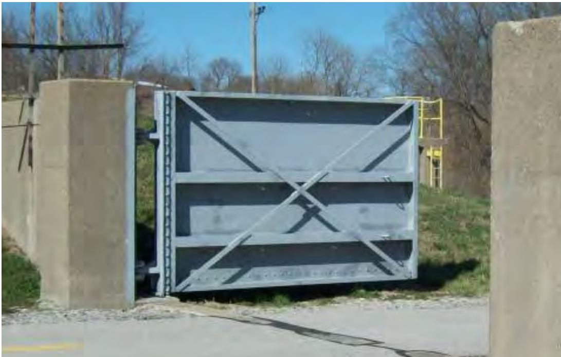
Figure F-2. Swing-Gate Closure Structure.
