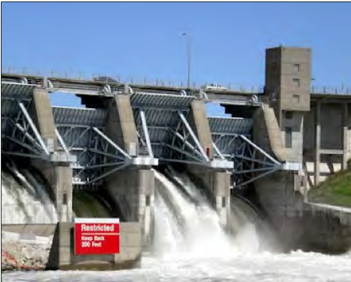
Figure B-4. Tainter Gate.
