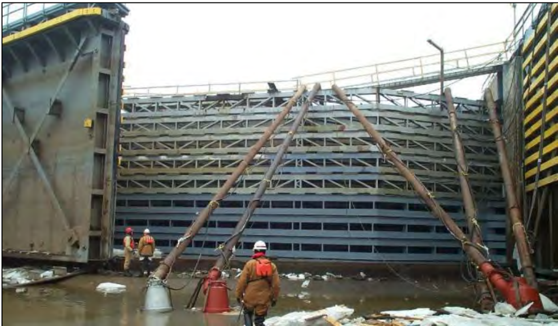
Figure B-6. Bulkhead.
