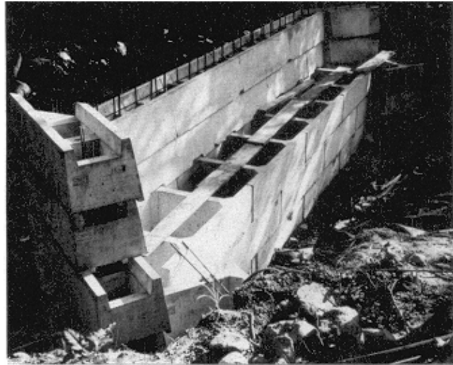
Figure 8-51. Top view of precast abutment prior to backfilling, Ulsterville Bridge
