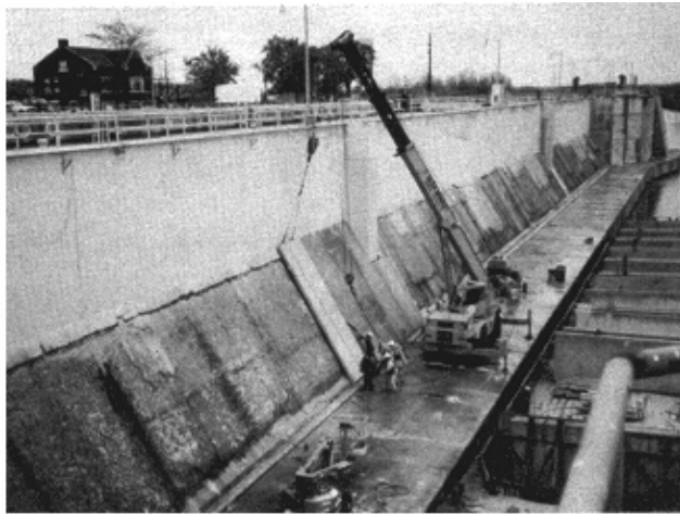
a. Installation of precast concrete panels
