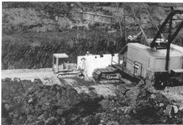
Figure 8-47. Channel section delivery and installation, Blue River Channel
