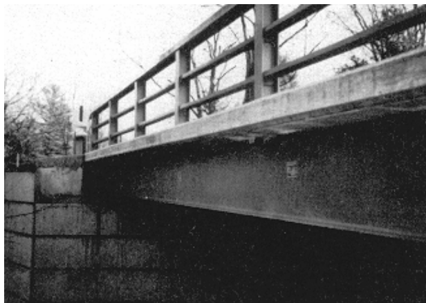
Figure 8-53. Precast abutment and deck units, Ulsterville Bridge
