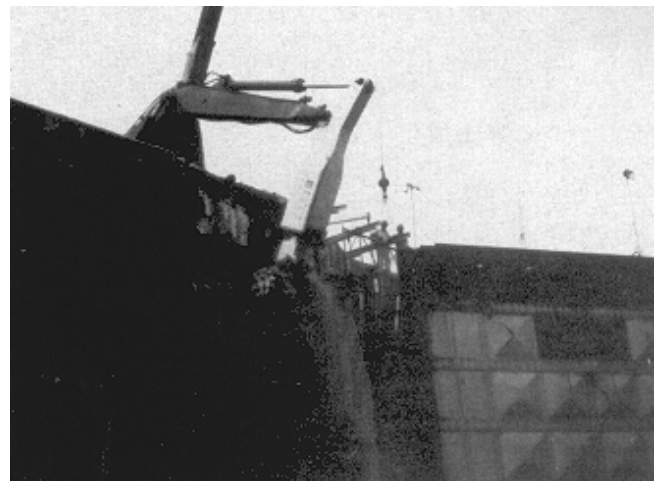
Figure 5-11. Rotary-head milling
