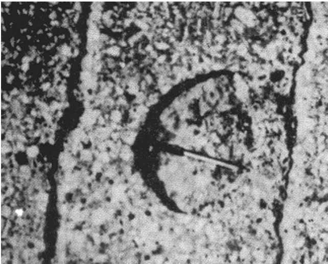
Figure 2-29. Small spall
