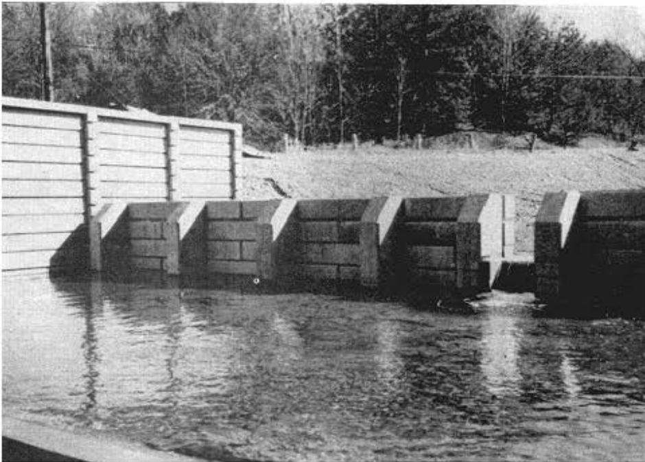
Figure 8-43. Precast concrete checkdams, Chauncy Run
