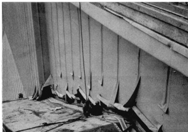
Figure 8-62. Installation of geocomposite, Pracana Dam
