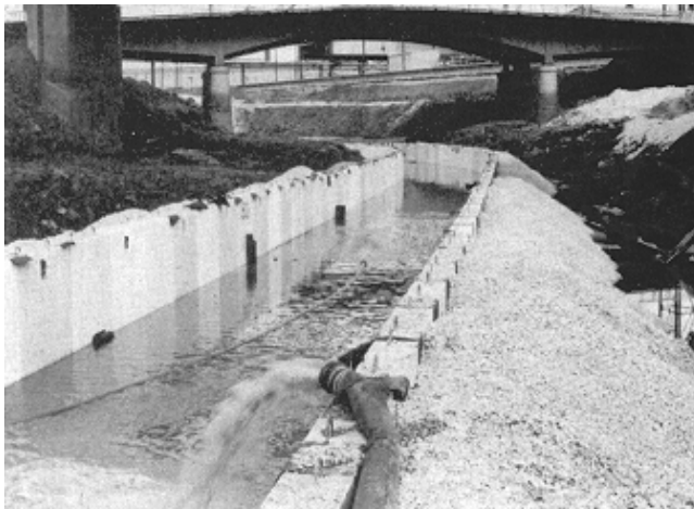
Figure 8-48. Diversion of river water through channel sections, Blue River Channel
