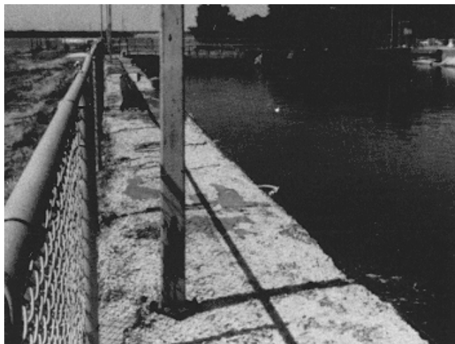
Figure 2-18. Severe scaling
