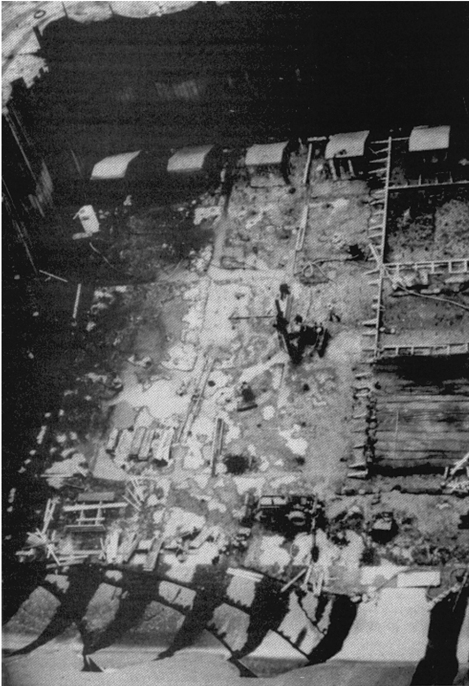
Figure 8-34. General view of repair operations, Kinzua Dam, 1974
