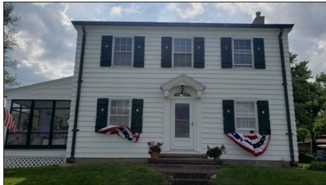
The Lock and Dam 10 lockmaster house in Guttenberg, Iowa, June 6. USACE photo by Melanie Peterson
