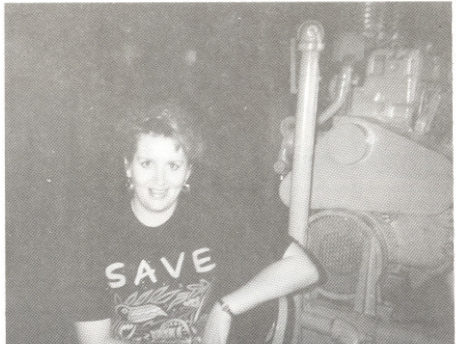
Karen Bostrom perches next to the backup generator at Lock and Dam #3, a place where her duties have changed from office to operation.
