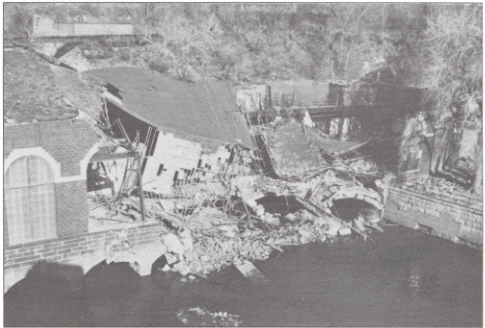
The collapse of the center portion of the hydro plant on Tuesday afternoon seemed to end the question of whether or not the structure could be repaired.
