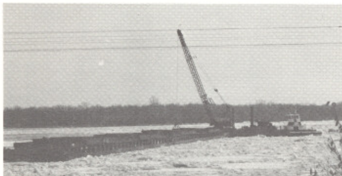
The barges were freed from the ice in Pool 7 in February.
