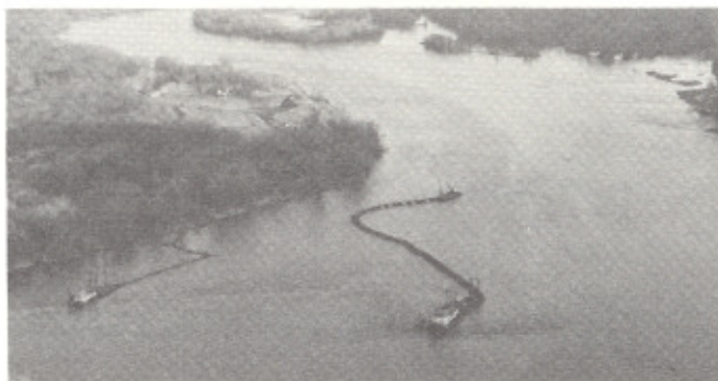
Reads Landing/Chippewa Delta dredging project.
