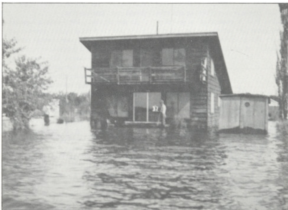
Shown above is one of the many homes that were surveyed in 1983 when the water level was 963.5 feet. Since that time, the lake has risen almost four feet.
