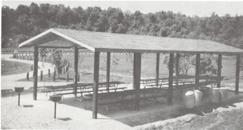
A second picnic shelter was added to the main day use area at the Eau Galle Recreation Area in May. The new pitched-roof wood structure shelters eight picnic tables and is immediately accessible from the main parking lot by a handicap ramp. This new shelter and the original nine-table wooden arch shelter are now equipped with electrical outlets.
