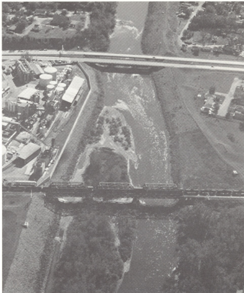
Two set of twin bridges across the Minnesota River will be relocated as part of the Mankato project.
