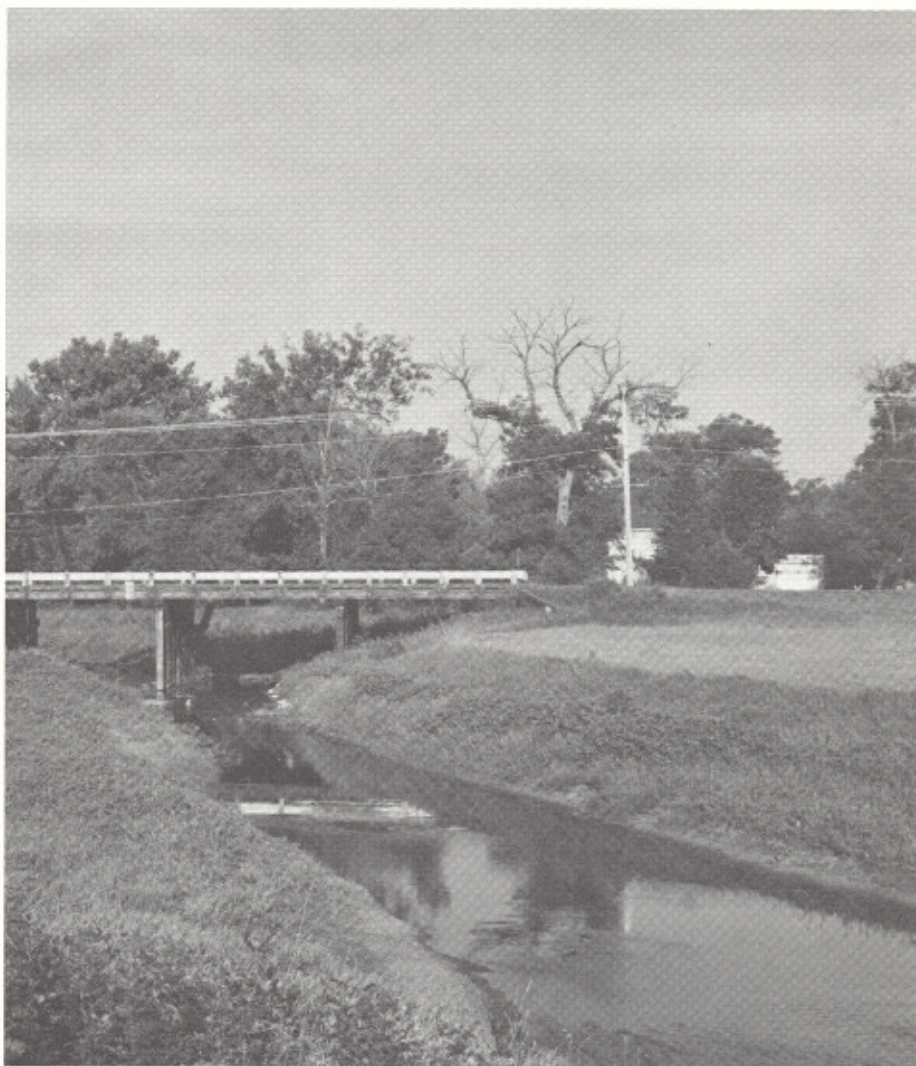
During high water the Redwood River (shown above) overtops a county highway.
