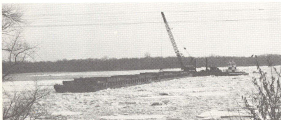
BARGES that were stuck in the ice at Pool 7, were forced to shore by the J.F. Brennan Company, February 26, 1984, and were tied to trees to secure them from floating away. After the ice cleared, the Brennan Company took the barges to La Crosse, Wis. This operation was completed March 3, 1984.
