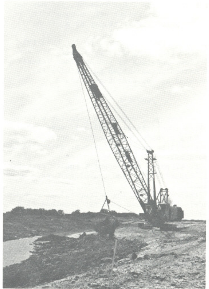
Channel excavation on South Branch. (Photo courtesy of Construction Branch)
