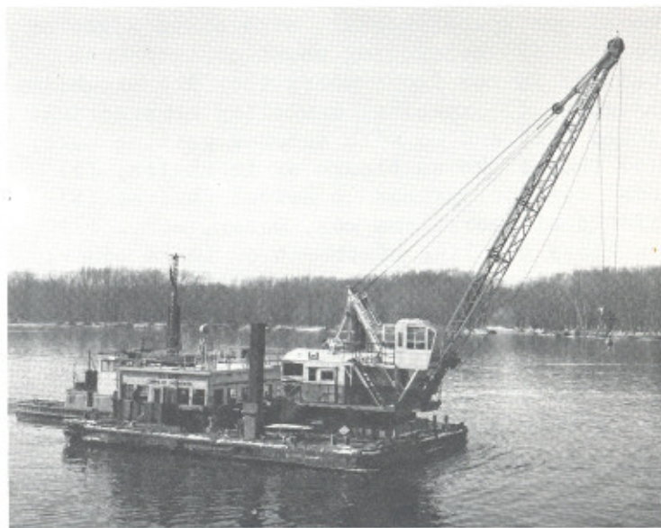
The Derrickbarge Hauser. (Photo by Lyle Nicklay, AS-P)
