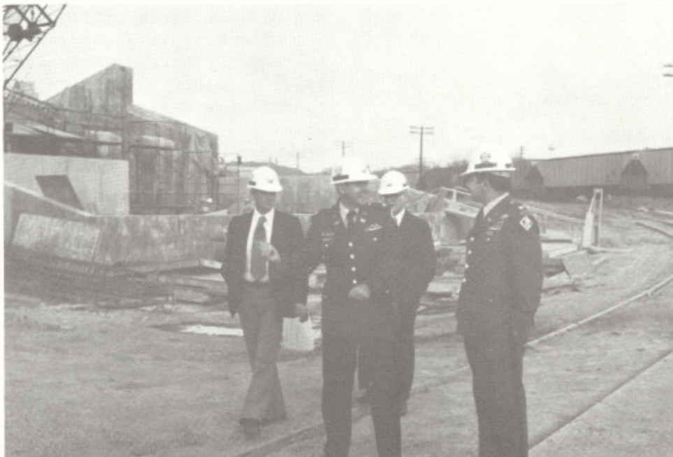
TOURING THE WORK AT THE MANKATO-NORTH MANKATO Flood Control Project were (from left to right) James Kursu, ED-P; North Central Division Deputy Division Engineer Col. Charles Shreves; Peter Fischer, ED; and Lt. Col. Stephen Draper, DD. Col. Shreves visited the St. Paul District in early November to receive briefings on district activities and operations. (Photo courtesy of James Kursu)
