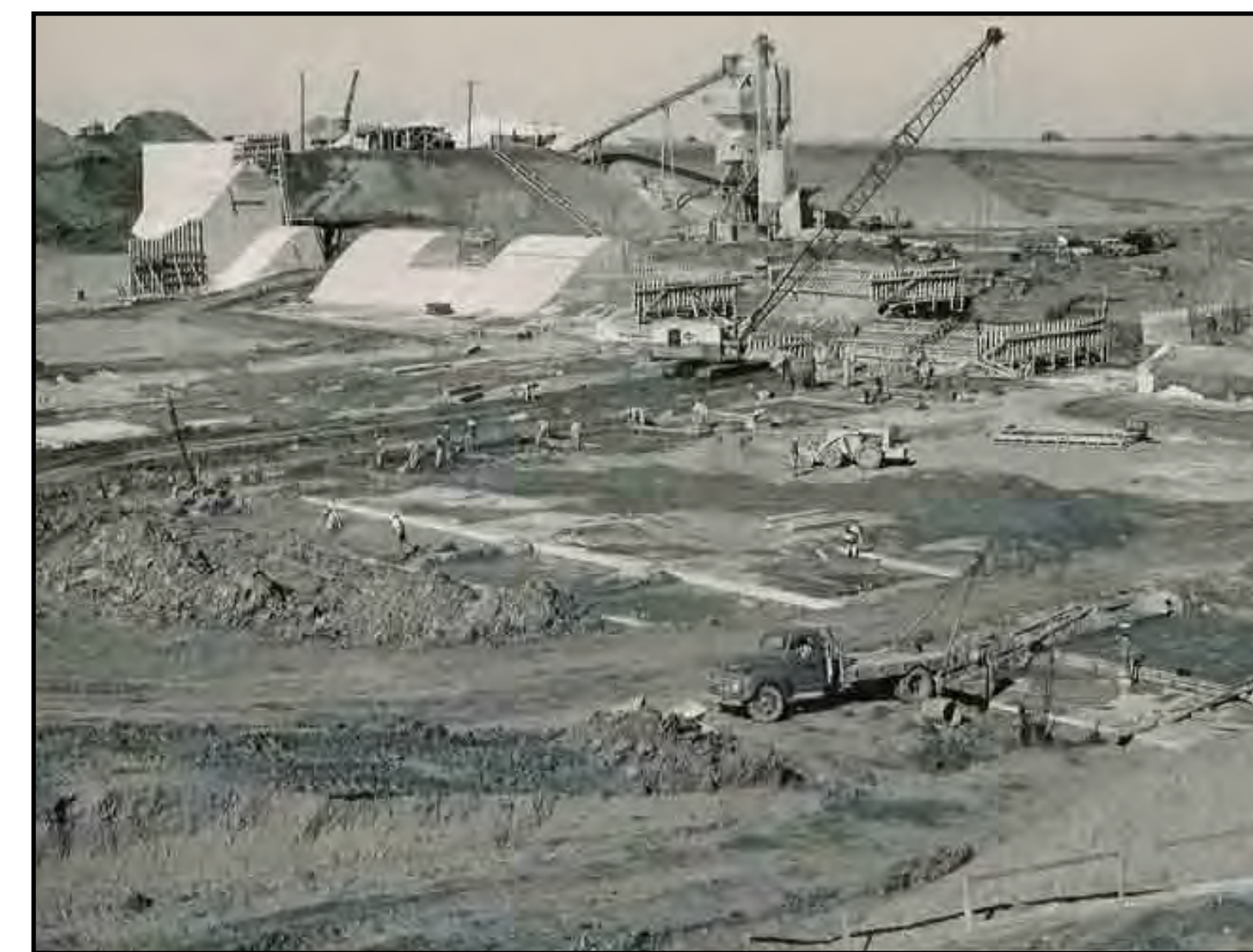
Construction of the Lewisville Dam (1952)
