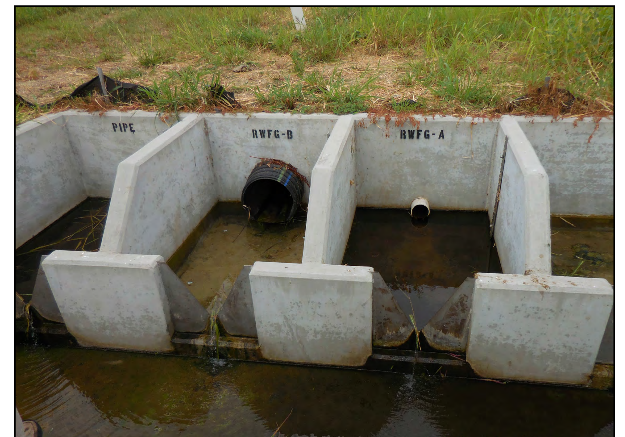
Existing Relief Wells at the Lewisville Dam
