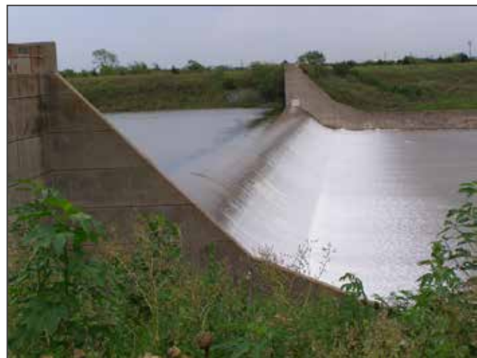
Figure 1-5 Lewisville Dam: View of Spillway Ogee Weir Looking Left
