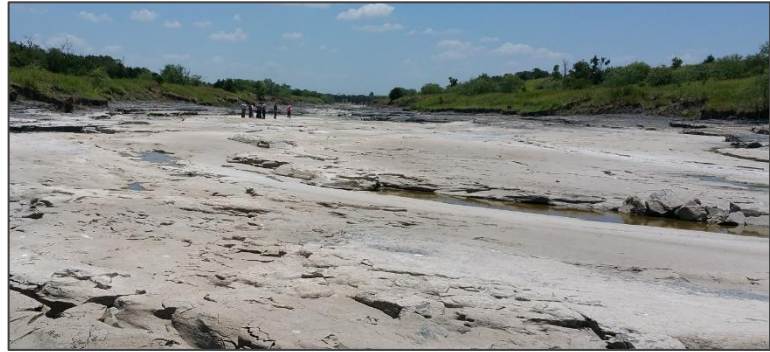
Figure 4.3-1 Spillway Channel Downstream of the Apron
