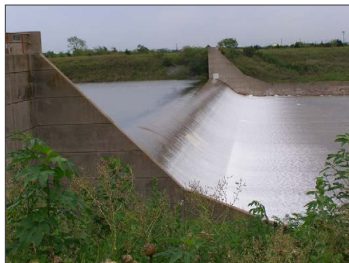
Figure 1-5 Lewisville Dam: View of Spillway Ogee Weir Looking East
