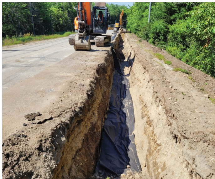
The contractor digs a trench to run the waterline.
