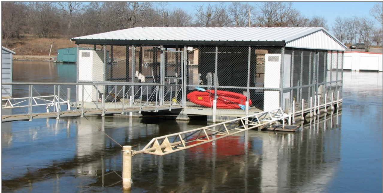
Photo 4.3 An Approved Chain Link Enclosure
