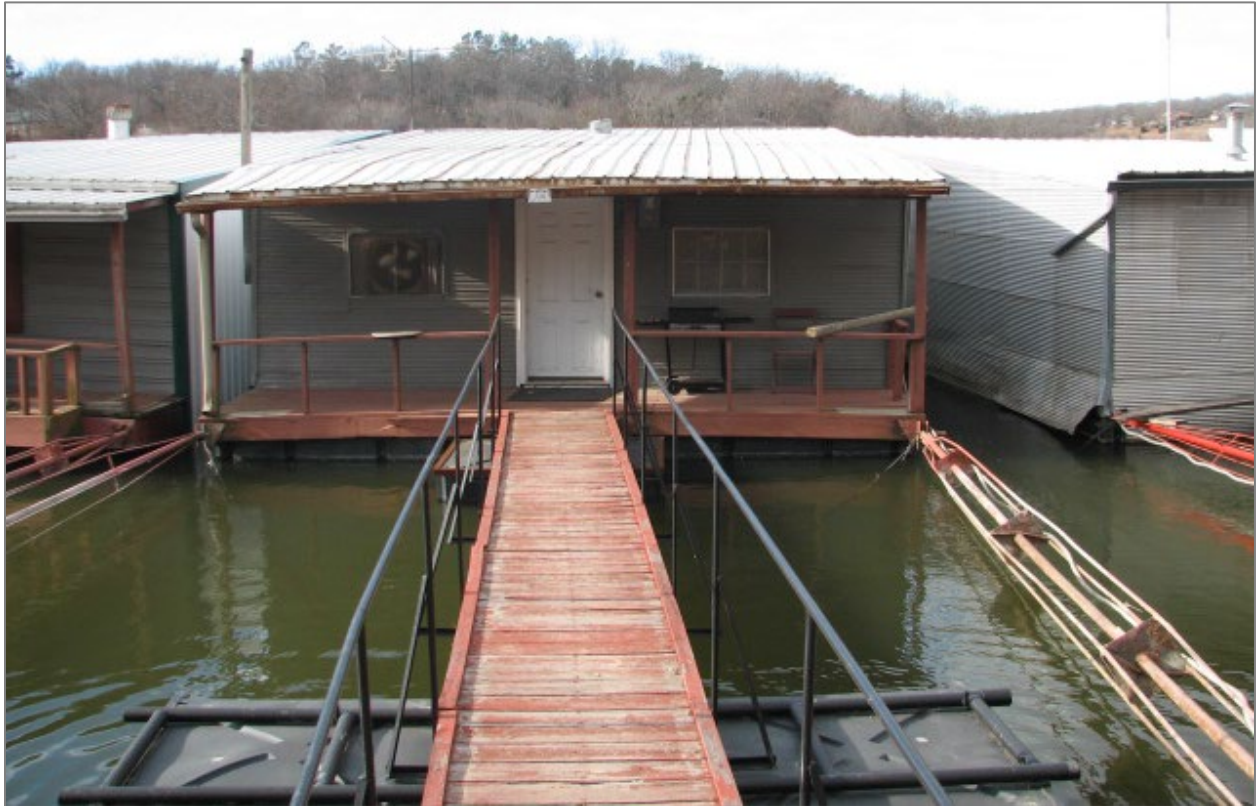
Photo 1.1 Older Facility Doesn't Meet Current Spacing and Construction Requirements
