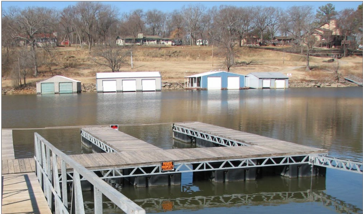
Photo 4.2 Example of Flotation on a Private Floating Facility
