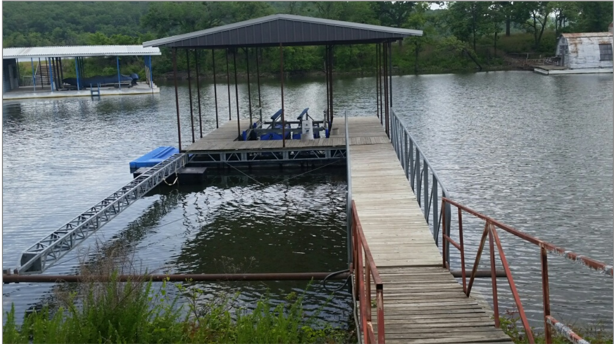
Photo 4.1 Example of Private Floating Facility, Walkway, and Stiff Arm
