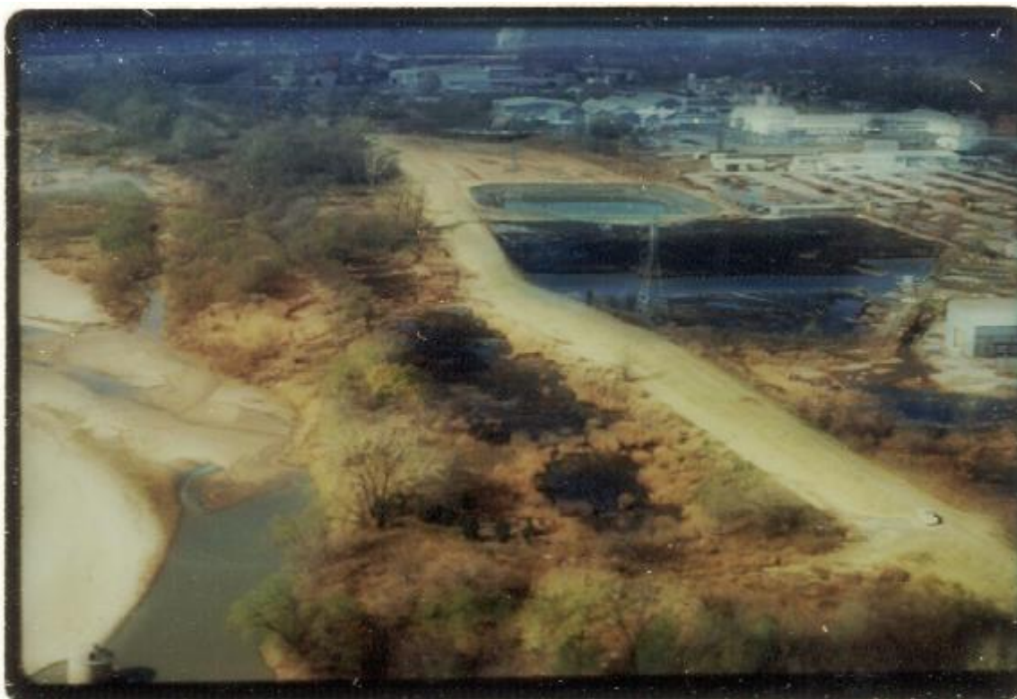
Figure 10: Sand Springs Petrochemical Site Photograph Prior To Excavation of Sludge, Looking west
