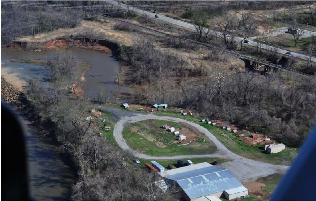
Figure 7: Prattville Creek & FFA Hog Farm looking Southeast, from Arkansas River Corridor Projects Site Reconnaissance Summary April 30, 2009; CH2M HILL
