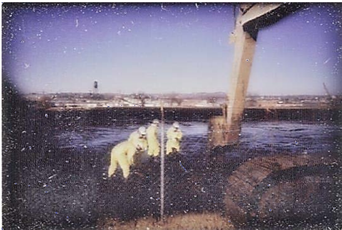
Figure 11: SSPC, Looking North during one of the Sludge Excavations (approximately 1989 to 1991)
