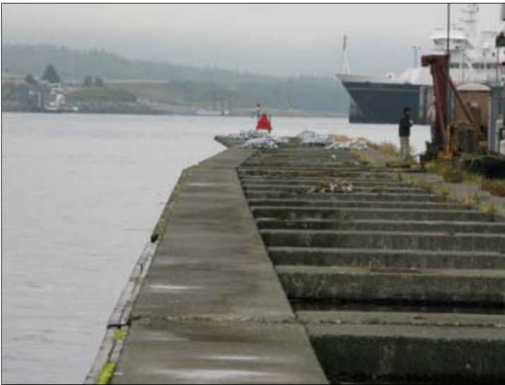
(Left) Failure of the cross-lateral tension cable system between the four modules of the large floating breakwater section caused an overall misalignment. (Right) Replacing all cross-lateral cables corrected the problem.
