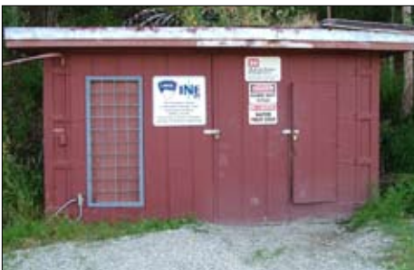
The entrance portal is one of three buildings at the site of the permafrost tunnel.
