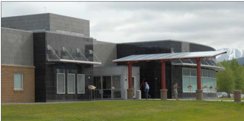
Fish art decorates the outside main entrance to the 36,390-square-foot Fort Richardson Health Clinic. The building’s location is oriented to take advantage of sunlight exposure to lower heating costs and brighten the atmosphere inside.
