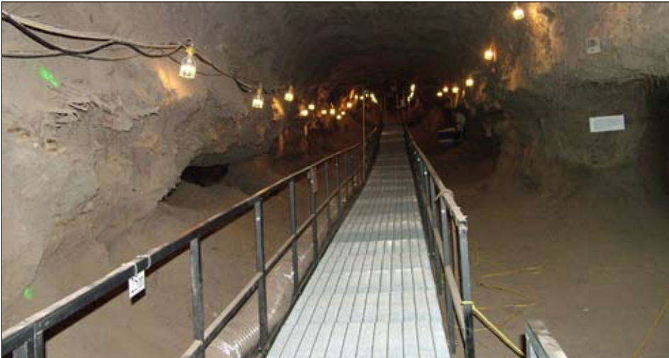
The main path inside the permafrost tunnel reaches 360 feet into the hillside. Near the entrance, a side tunnel excavated later to study underground mining techniques, drops more steeply for 200 feet to frozen gravels and bedrock.
