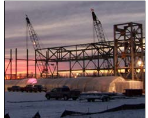
Shelters allowed welders to assemble the steel frame in cold weather (above). A high light-reflective floor is one of the improvements to the new Hangar 6. (U.S. Army Corps of Engineers photos)
