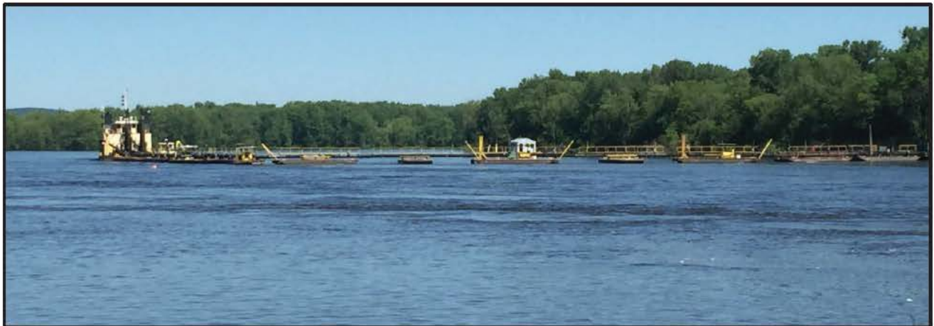
Figure 5. Dredging operations at the Chippewa Delta Cut in Lower Pool 4, July 22, 2016
