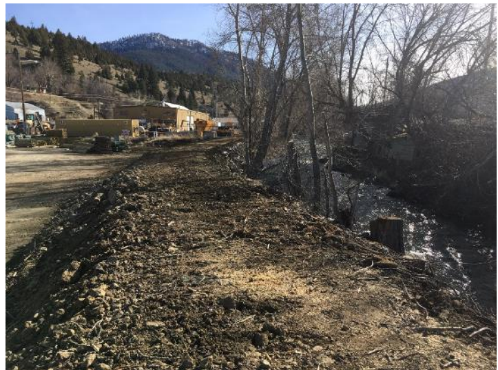
Temporary Berm Constructed in Canyon City
