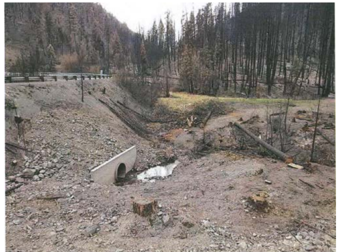
Vance Creek culvert before replacement
