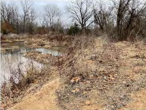
West – Below Lock 16
