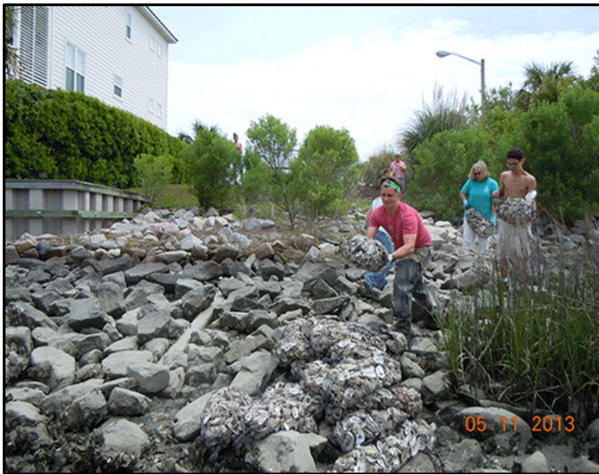
Figure F-5 Volunteer group working with the CORRI program to place bagged recycled oyster shells in Hog Inlet to restore the oyster reef habitat in this part of the estuary.
