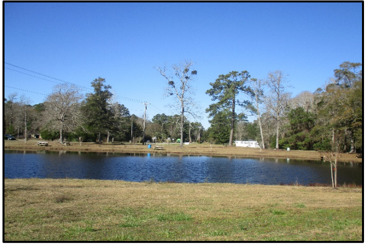
Figure A-8. Stormwater pond within the Riverside Dr. neighborhood.
