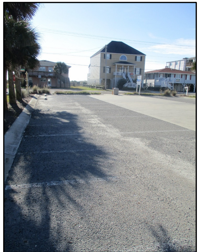
Figure E-4 Pervious concrete pavement at a beach access parking lot at 53 rd Ave North and Ocean Blvd.
