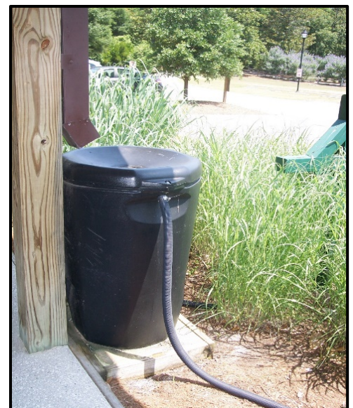
Figure F-2 Typical rain barrel setup for a small to medium sized residential building or a small commercial building.
