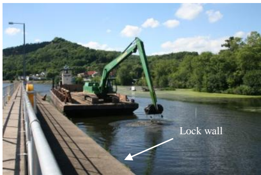
Dredging along the lock wall. 500 cubic yards were removed. USFWS
