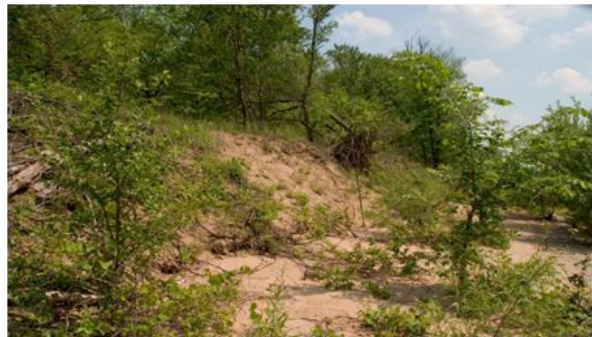
Figure . Archeological site erosion USACE
