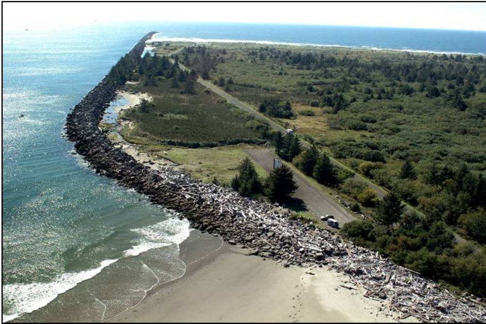
Figure A1- 99. North Jetty Root – Looking West
