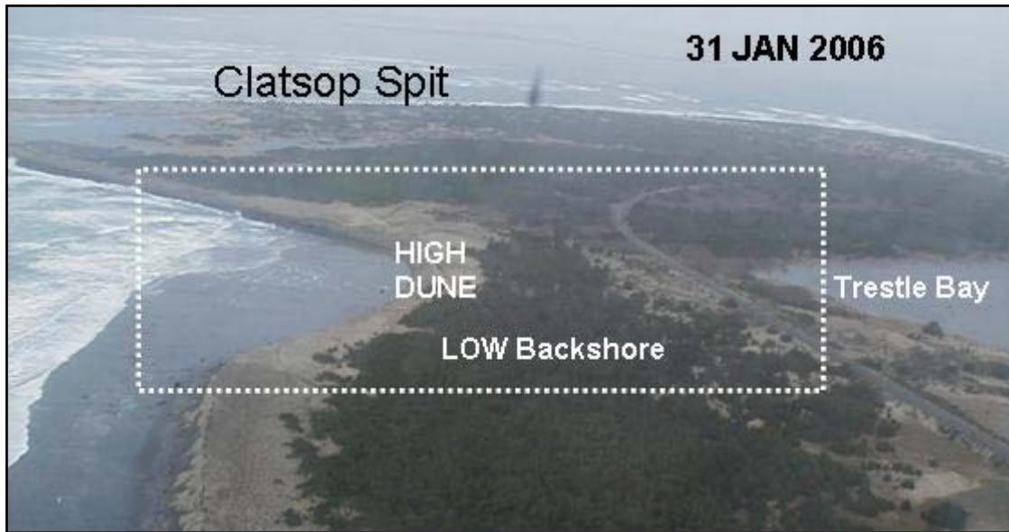
Figure 19. Clatsop Spit and South Jetty Root Erosion
