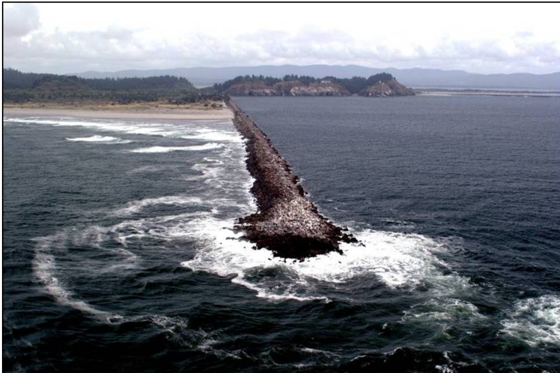
Figure A1- 107. North Jetty Head
