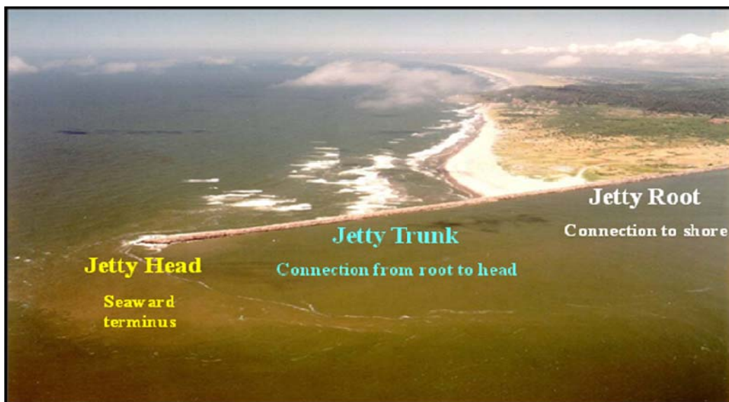
Figure 3-12. North Jetty, View to the North
