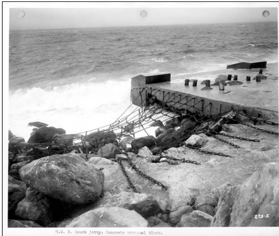
Figure A1- 49. South Jetty concrete monolith construction photos – 1940s
