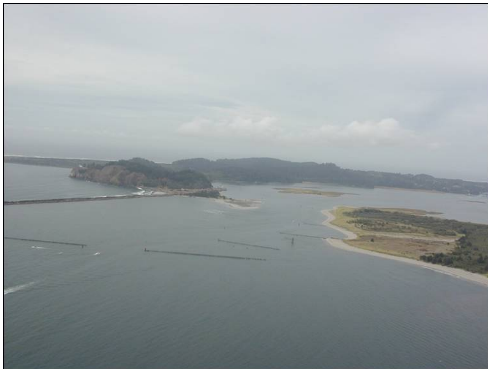
Figure A1- 143. Jetty A and Ilwaco Channel
