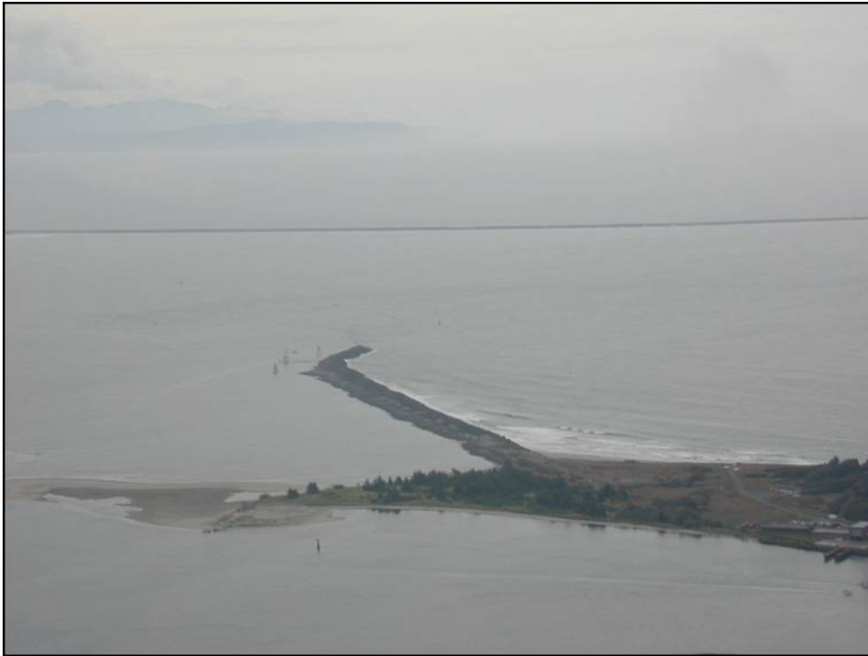
Figure A1- 144. Jetty A and Root
