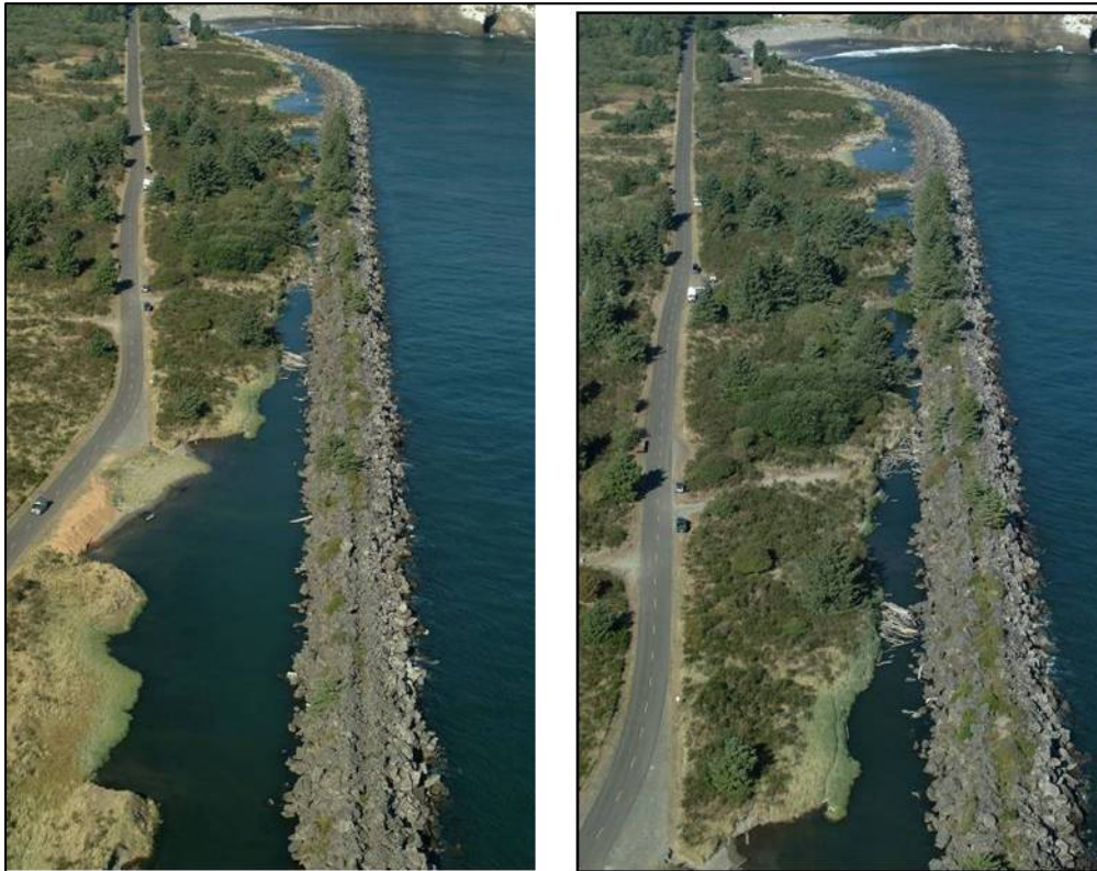
Figure A1- 101. North Jetty Root – Looking East
