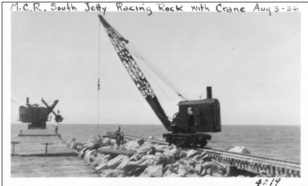
Figure A1- 50. South Jetty repair photos – 1930s.
