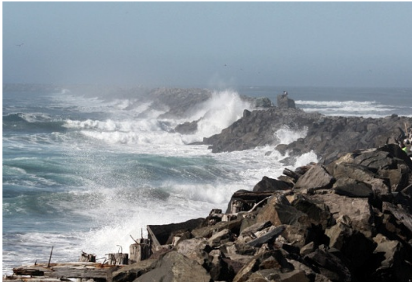
Figure 20. Photograph of the South Jetty in September.
