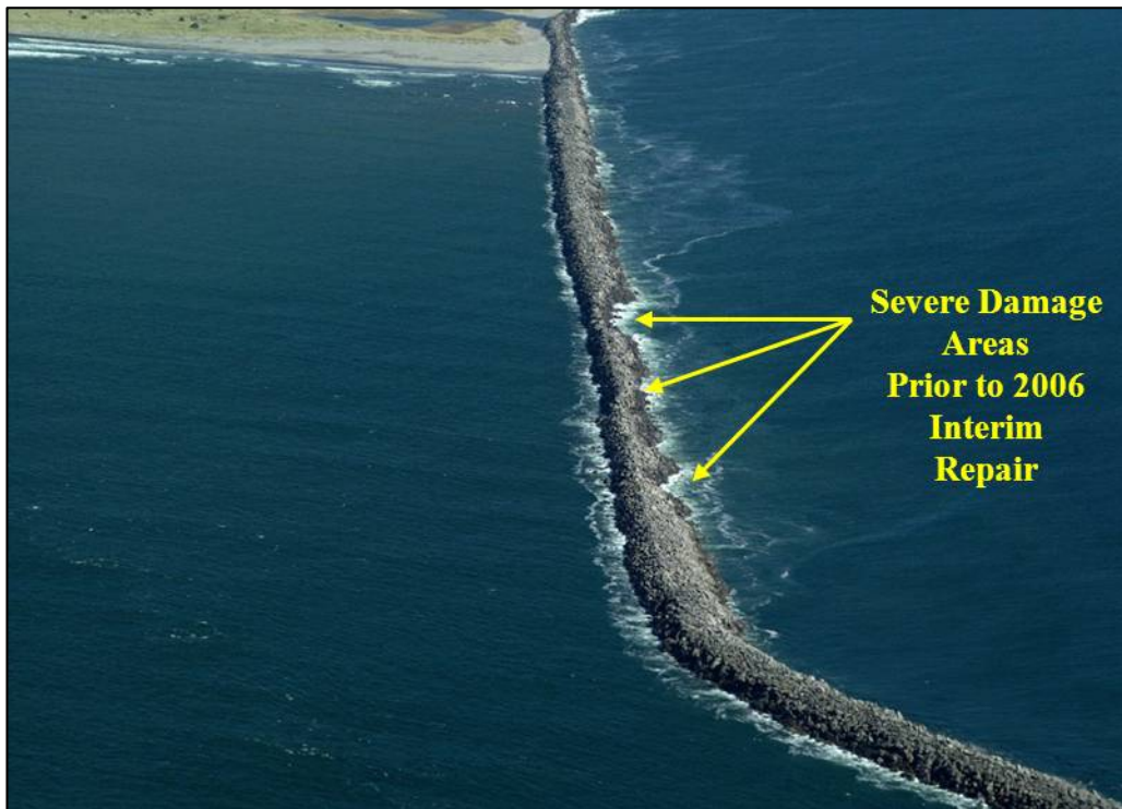
Figure A1- 122. South Jetty Inner Trunk
