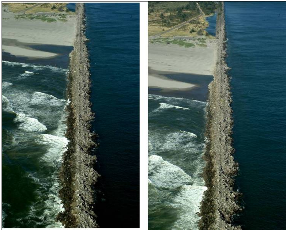
Figure A1- 102. North Jetty Trunk - Looking East
