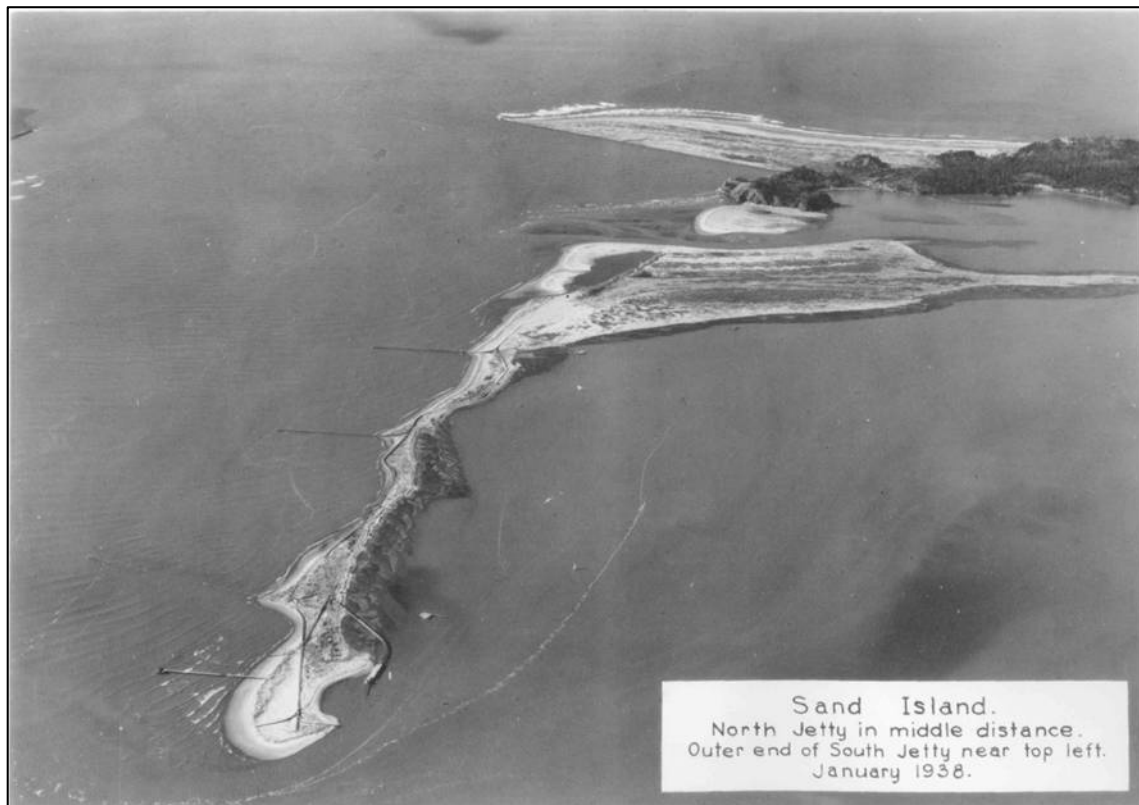
Figure A1- 9. Sand Island Pile Dikes
