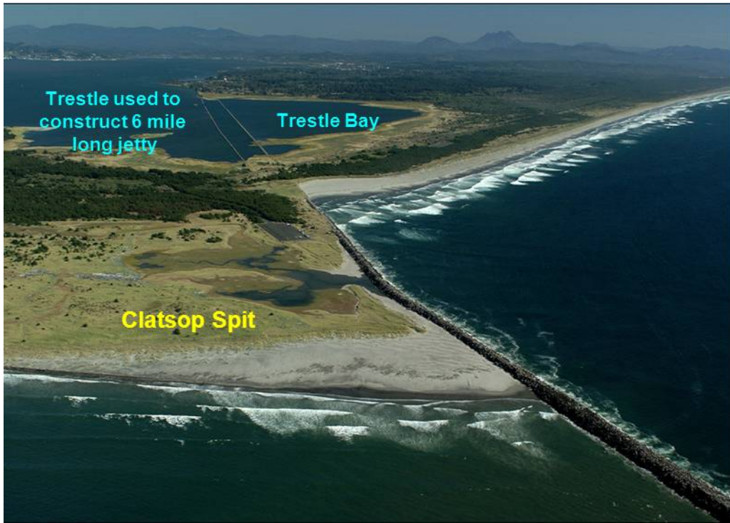
Figure A1- 120. South Jetty Root and Trestle Bay
