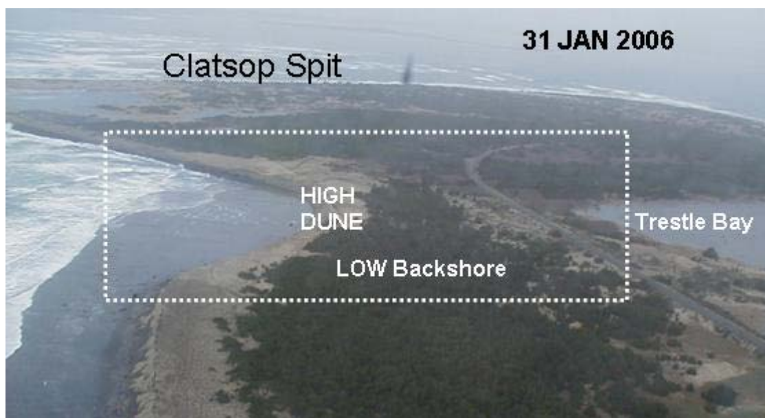
Figure 11. Clatsop Spit and South Jetty Root Erosion
