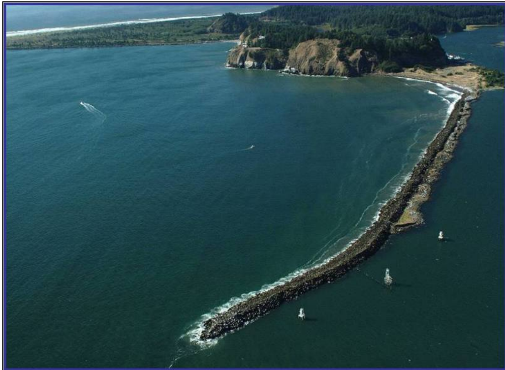
Figure A1- 8. Jetty A
