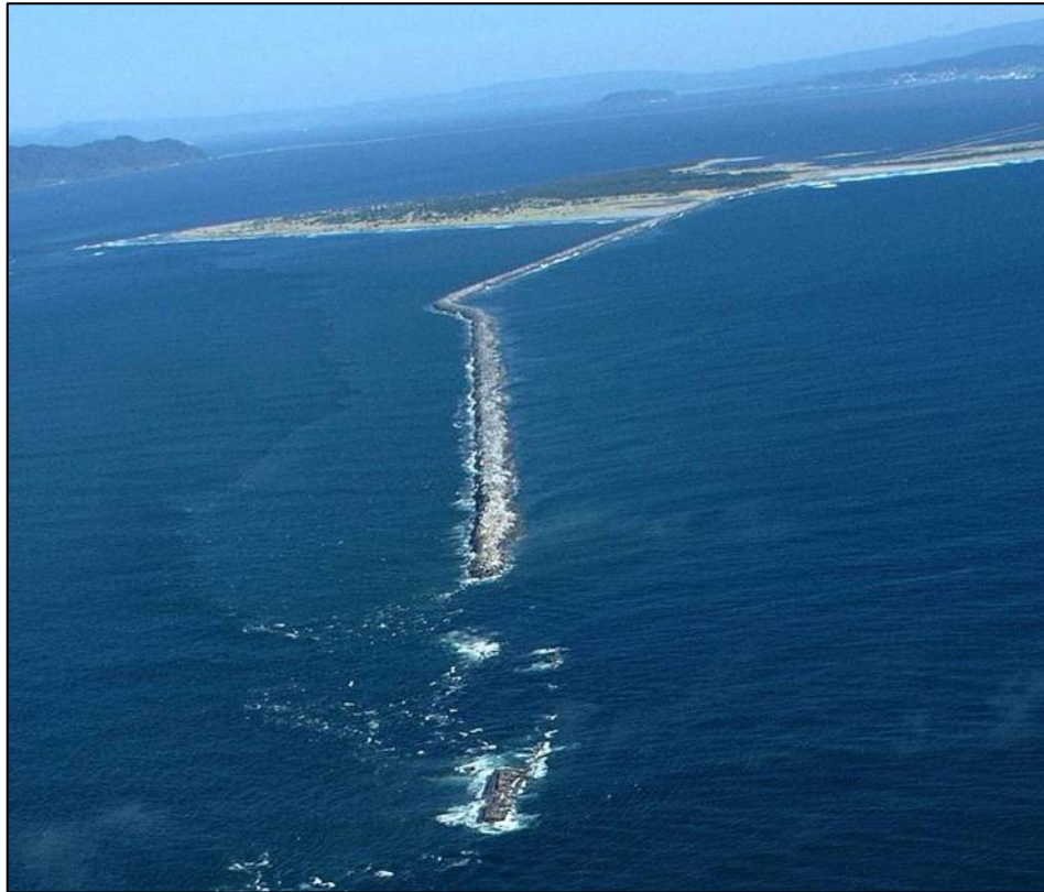
Figure A1- 128. South Jetty Seaward Trunk and Head
