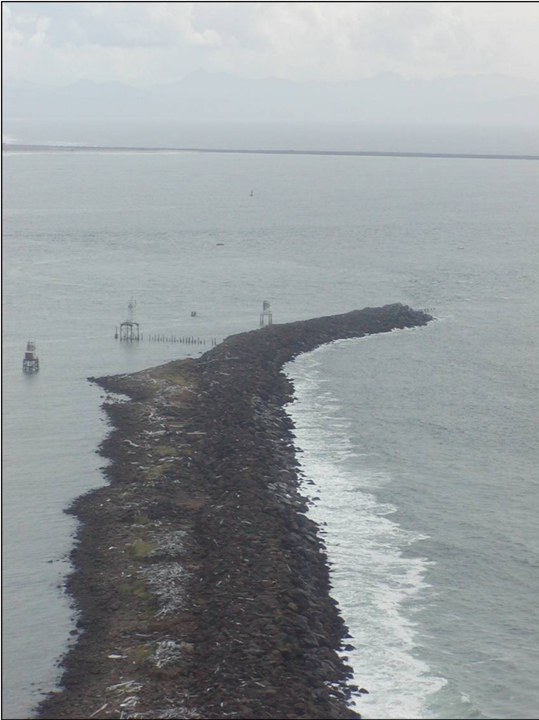
Figure A1- 145. Jetty A Trunk
