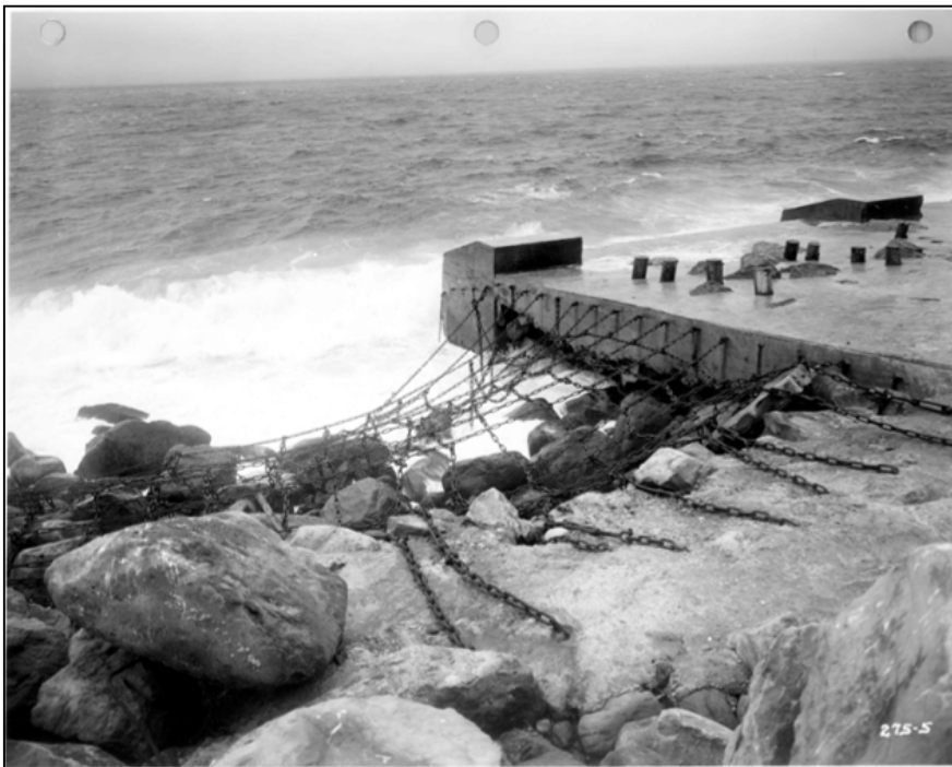
Figure 1-20. Concrete Monolith Construction at Seaward End of the South Jetty
