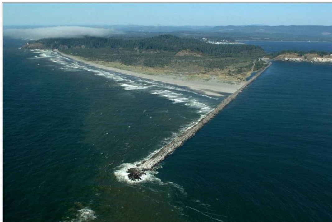
Figure A1- 6. North Jetty
