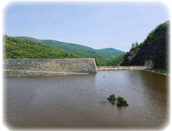
Ball Mountain Dam holding back water during the July flood.
