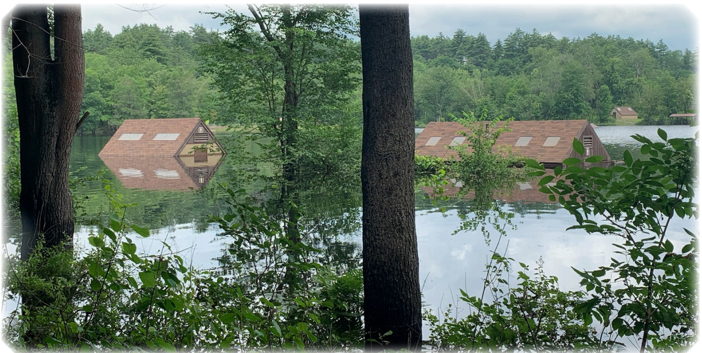
Surry Mountain Beach change house and rest room were under water during the flood.
