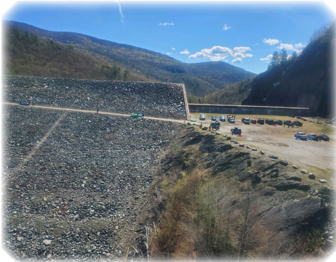
Ball Mountain Dam in May 2023 before the flooding.
