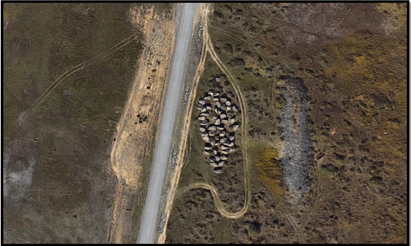
Figure 10. Stockpiles of stones, large (left) and small (right), from an earlier South Jetty repair, at the second staging area for the South Jetty.
