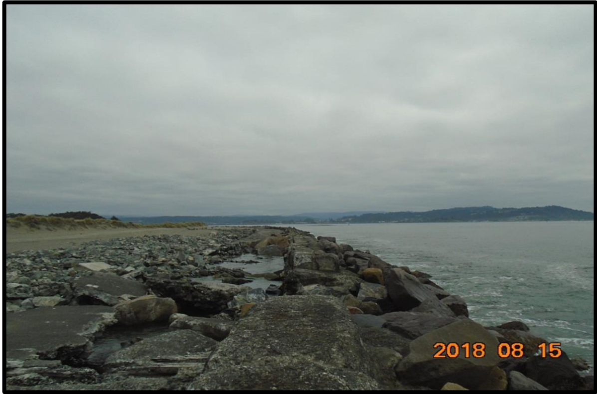
Figure 3. Photo of concrete cap in need of repair (Type 1).
