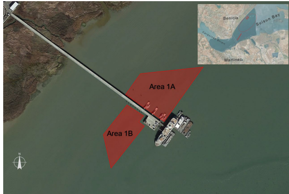
Figure 2. Overhead view of Area 1.
