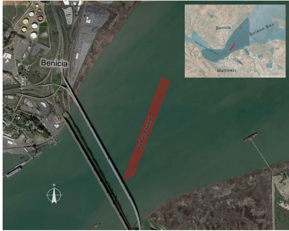
Figure 3. Overhead view of the Pass Area.
