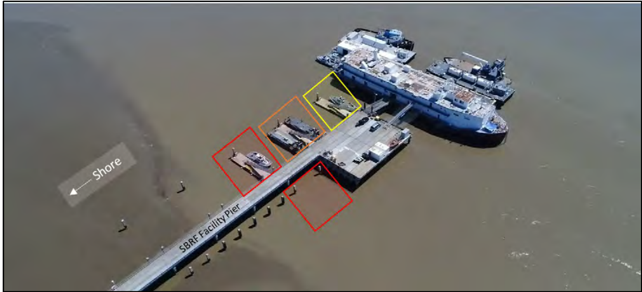
Figure 4: Overhead view of SBRF facility pier during low tide in 2018.
