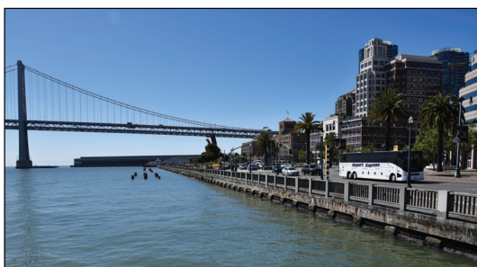
The San Francisco waterfront along the Embarcadero is protected by a seawall more than a century old.
