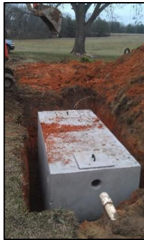
Example of Septic Tank Replacement
