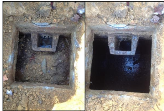
Example:Septic Tank Maintenance: Before and After
