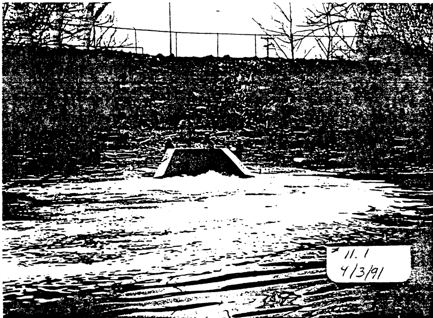
Figure 1. Storm Sewer Outfall, Glassport, PA 36 Inch Diameter Cast Iron Pipe Monongahela R.M. 15.7
