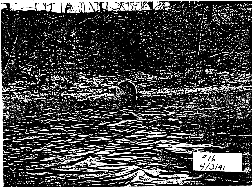
Figure 2. Sanitary Sewer Outfall, McKeesport, PA 54 Inch Reinforced Concrete Pipe Monongahela R.M. 17.8
