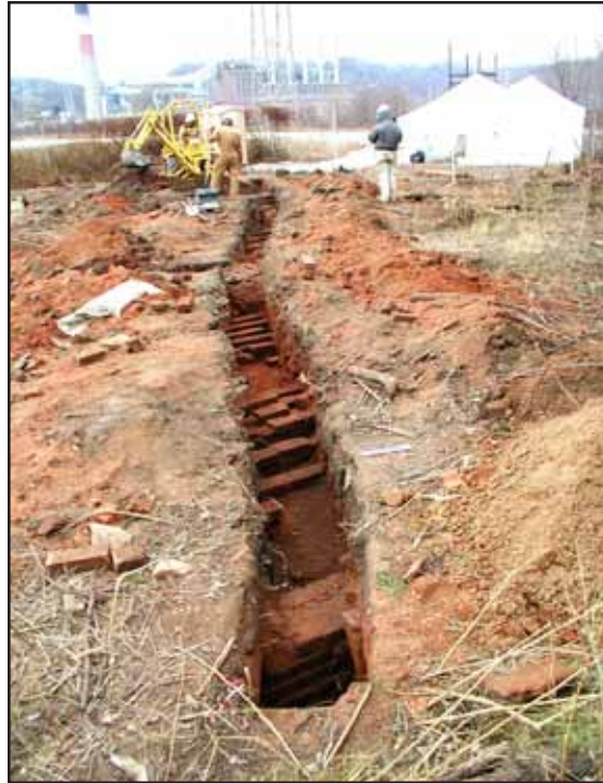
A trench cut by the backhoe, with part of the factory exposed.
