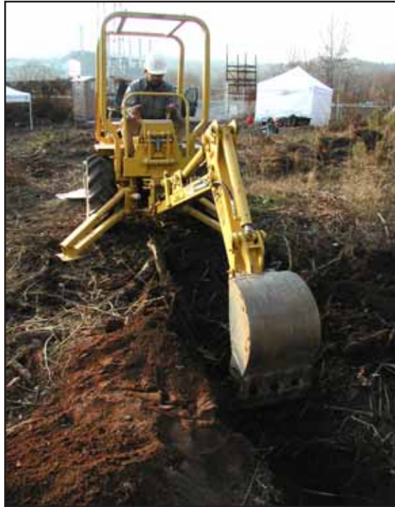
A backhoe at work on the site.
