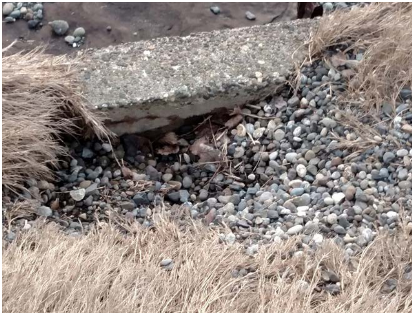
(Left and Right) Damage to the Alki Seawall is seen as coastal storms and erosion continue to threaten public infrastructure located in and around the project footprint. (Photos by Dallas Edwards)
