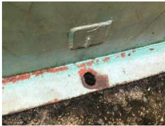
Missing Anchor Bolt
