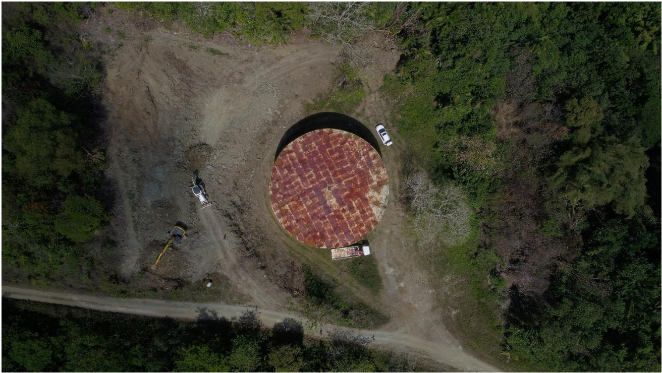
Tank 2 Site Photo ( Aerial View )
