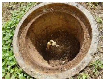
Disconnected Cathodic Protection
