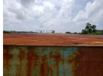
Through-Hole Corrosion on Roof
