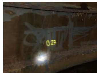
Typical Vertical Weld Pitting
