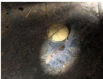
Level Float Disconnected
