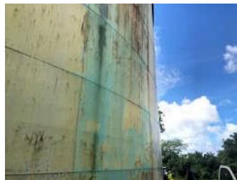
Typical Shell Plate Pitting
