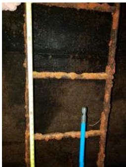
Corroded Internal Vertical Ladder
