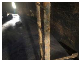
Corroded Internal Ladder
