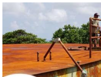
Damaged Level Gauge
