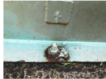
Typical Cathodic Protection Disconnection
