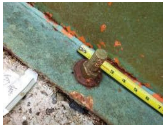
Disconnected Cathodic Protection
