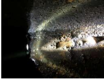
Typical Failed Coating on Bottom Welds
