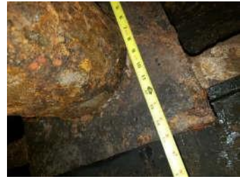
Through-Hole Corrosion on Roof
