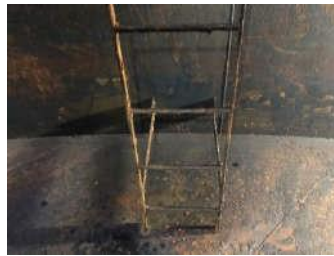
Corroded Internal Ladder
