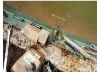
So Sealant Present on Bottom to Foundation Interface
