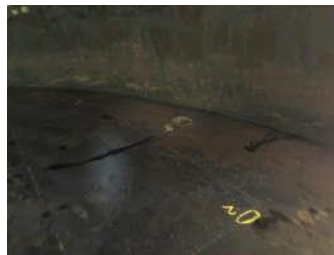
Bottom Butt-Weld Corrosion
