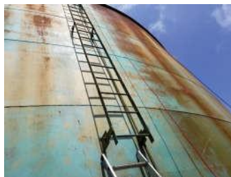
No Fall Arrest System on External Vertical Ladder
