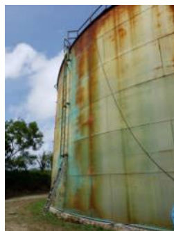
No Fall Arrest System on External Vertical Ladder
