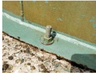
Missing Anchor Bolt
