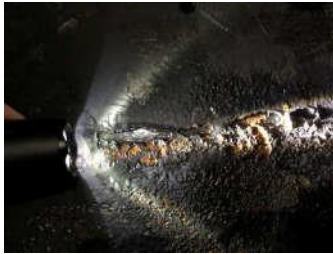
Typical Failed Coating on Bottom Welds
