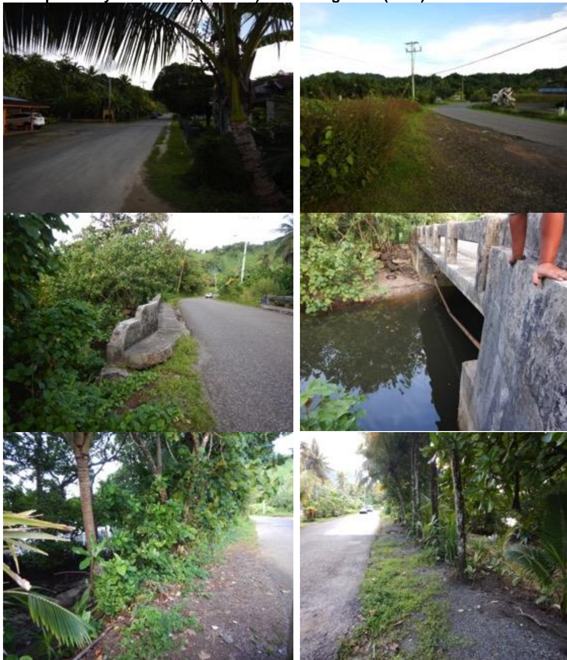
Figure 15: Representative photos of the road easement associated with the fiber cable terrestrial alignment, (a) road in close proximity to BMH, (b) road in close proximity to the CLS, (c and d) main bridge and (e & f) coastal shoreline.
