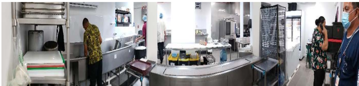
Temporary Kitchen Project: A container was manufactured with required specifications
