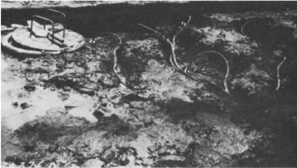
Figure C-6. Boundary Strain Meters in Place (courtesy of the Tennessee Valley Authority).
