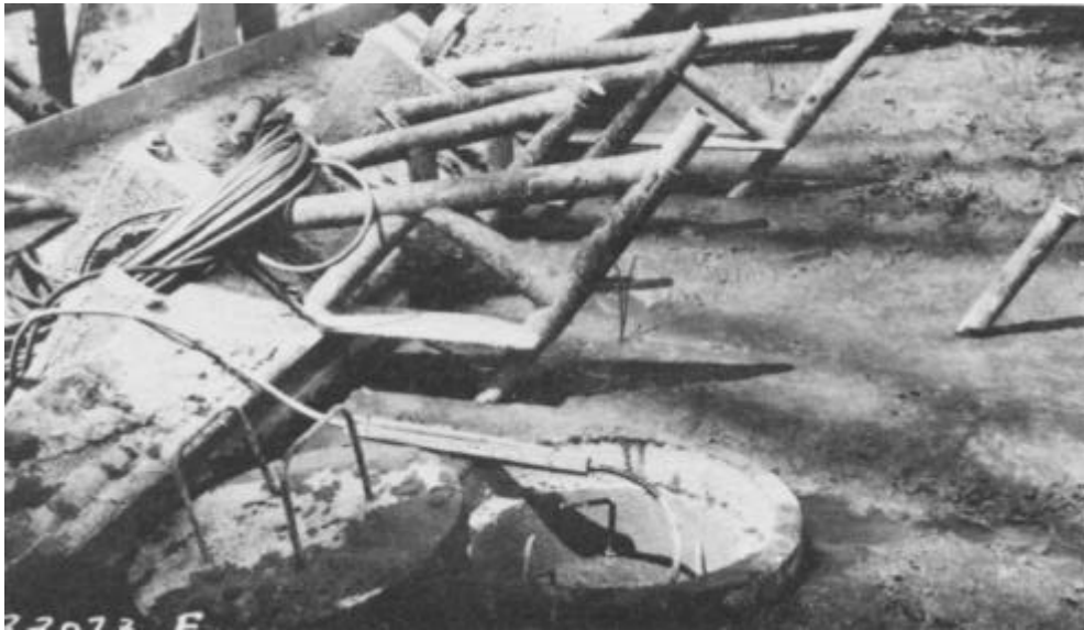
Figure C-9. No-Stress Meter Cavity and Cover (Courtesy of the Tennessee Valley Authority).
