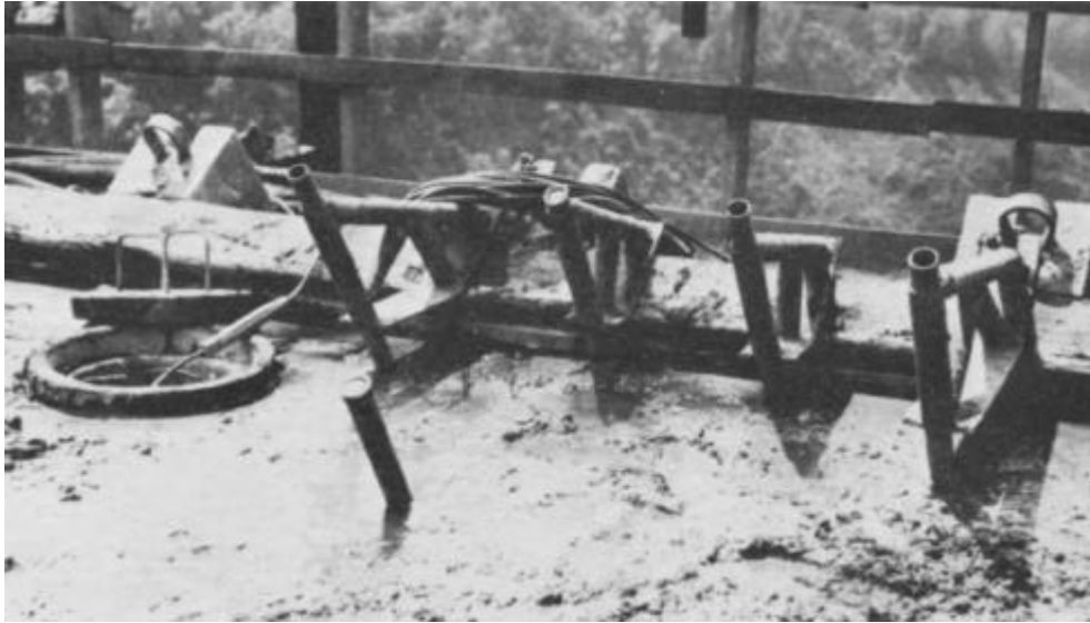
Figure C-5. Pipe Brackets for Locating Boundary Strain Meters - After Concrete is Placed (courtesy of the Tennessee Valley Authority).
