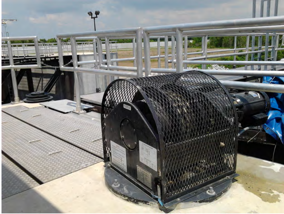
Figure 5-4. Backup winch system
