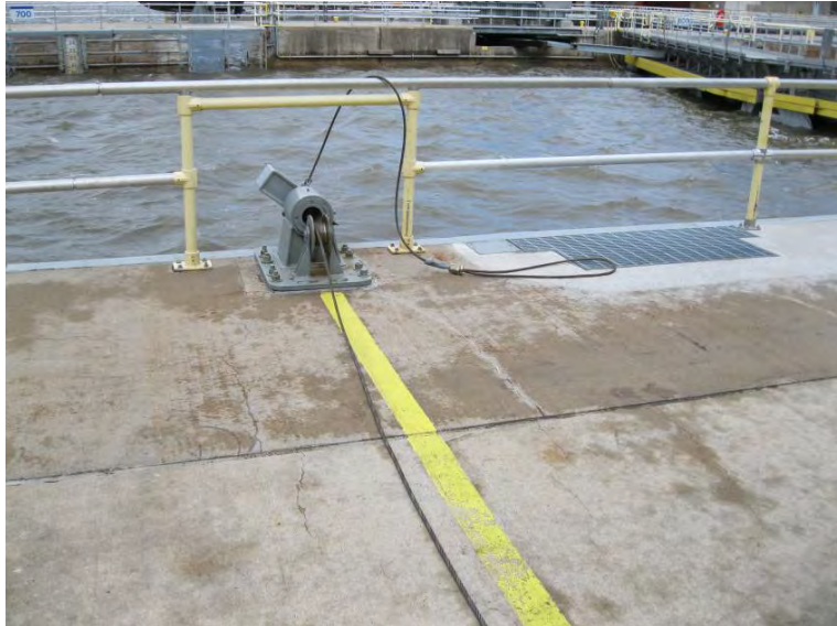
Figure 10-3. Fairlead for the tow haulage winch
