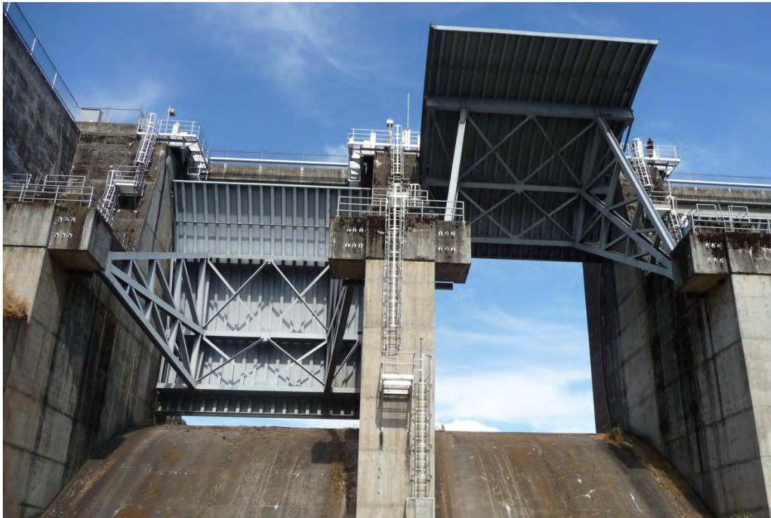
Figure 9-1. Conventional spillway tainter gate
