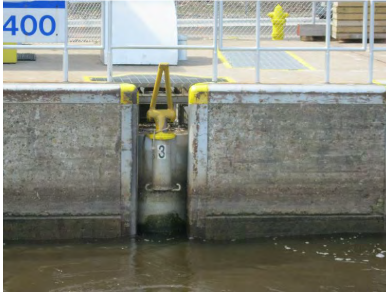
Figure 10-17. Single Bitt System
