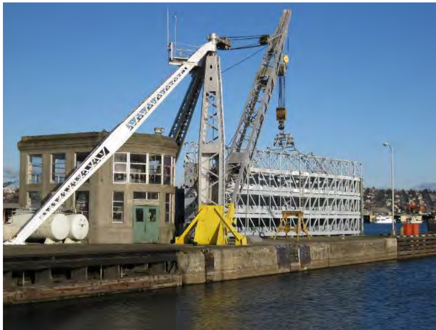
Figure 10-44. Emergency bulkhead crane system, Chittendon Lock, Lake Washington Ship Canal
