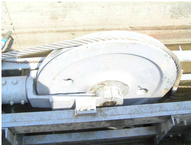
Figure 2-41. Wire rope sheave
