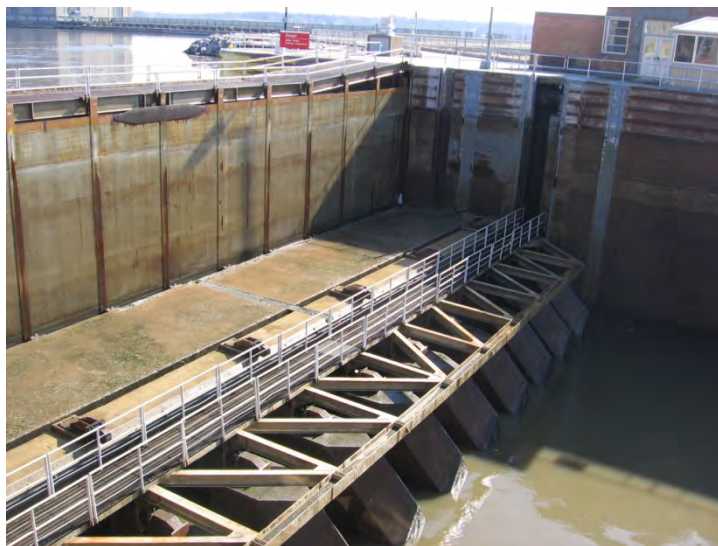
Figure 7-6. Single-leaf emergency gate
