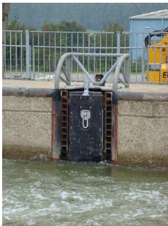
Figure 10-20. Born Locks, bollard is pressed against the end stop and the water level is raised to highest point
