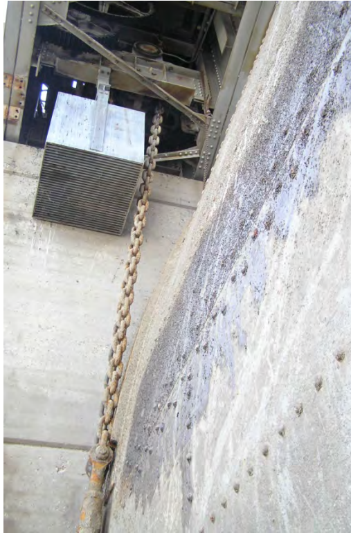
Figure 2-31. Pocket wheel chain hoist with chain locker
