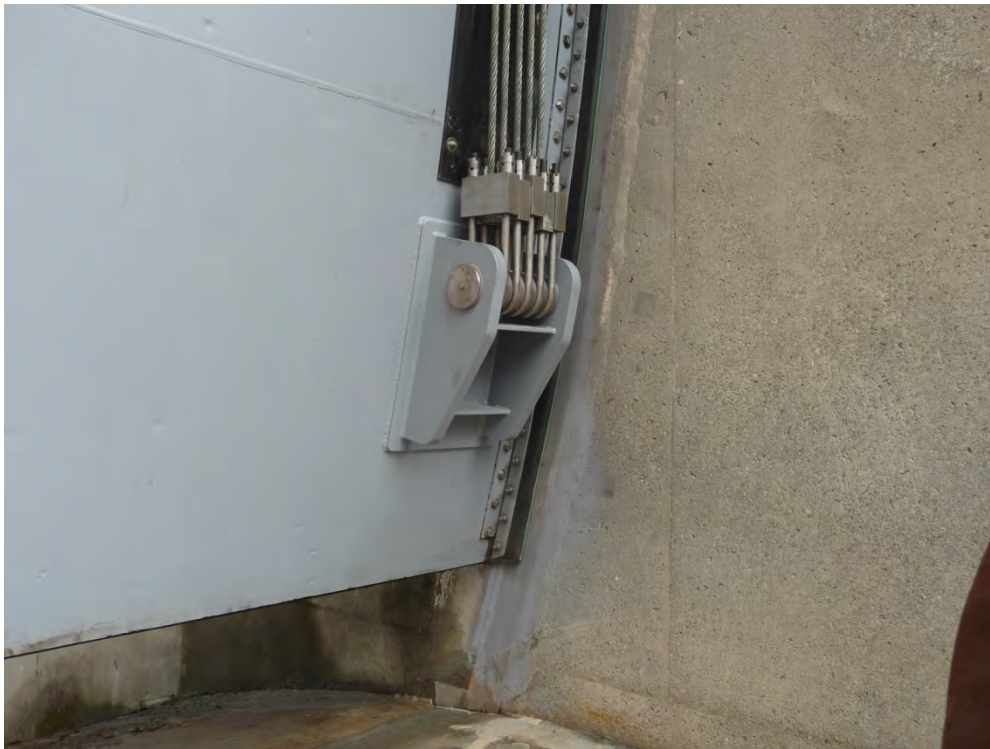
Figure 9-6. Wire rope gate connection
