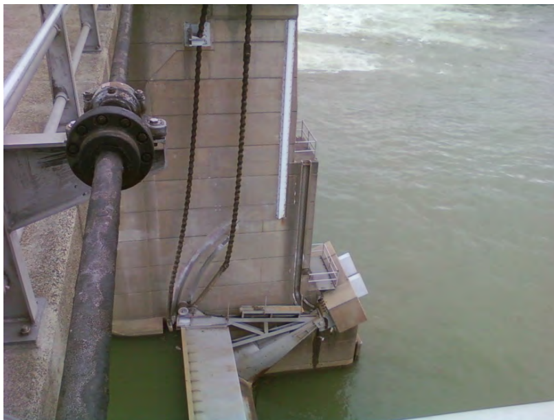
Figure 7-9. Multiple-section, radial crest gate
