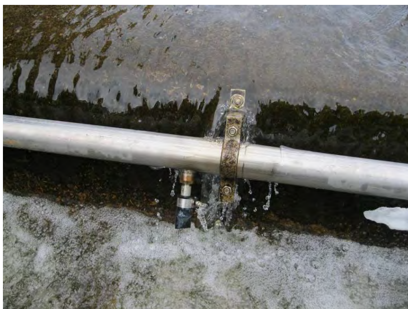
Figure 10-13. Rubber pinch-type check valve
