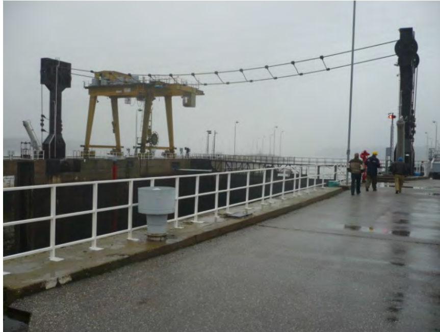
Figure 10-34. Fender net, Djerdap Lock
