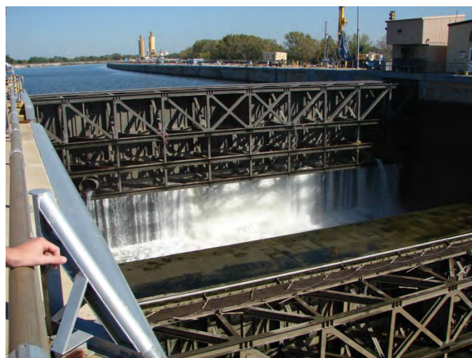
Figure 7-4. Emergency gate used for lock closure
