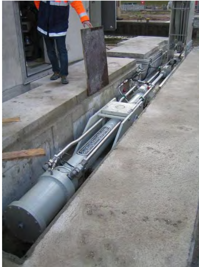
Figure 10-31. Hydraulic-driven arrestor system, Germany
