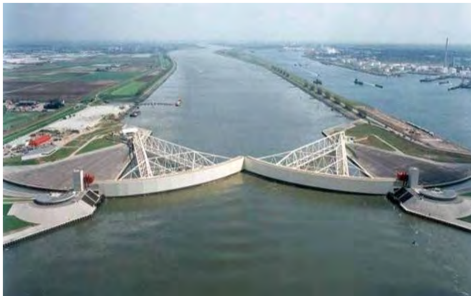
Figure 8-1. Buoyant sector gates of the Maeslant Barrier, Netherlands, in closed position (courtesy of R.A. Daniel, Rijkswaterstaat, Division of Infrastructure, Netherlands)
