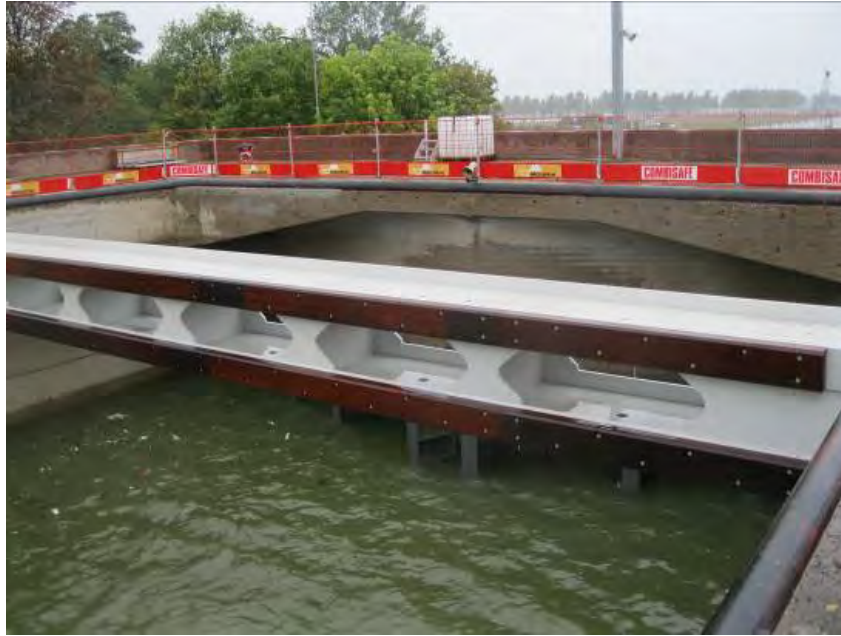
Figure 10-30. Ship arrestor, Born Locks
