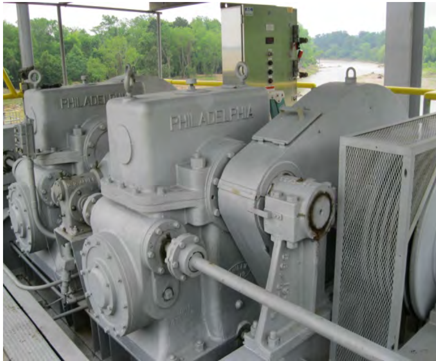
Figure 9-5. Wire rope electric motor hoist
