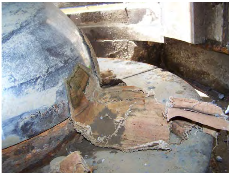
Figure 2-5. Failed pintle bushing
