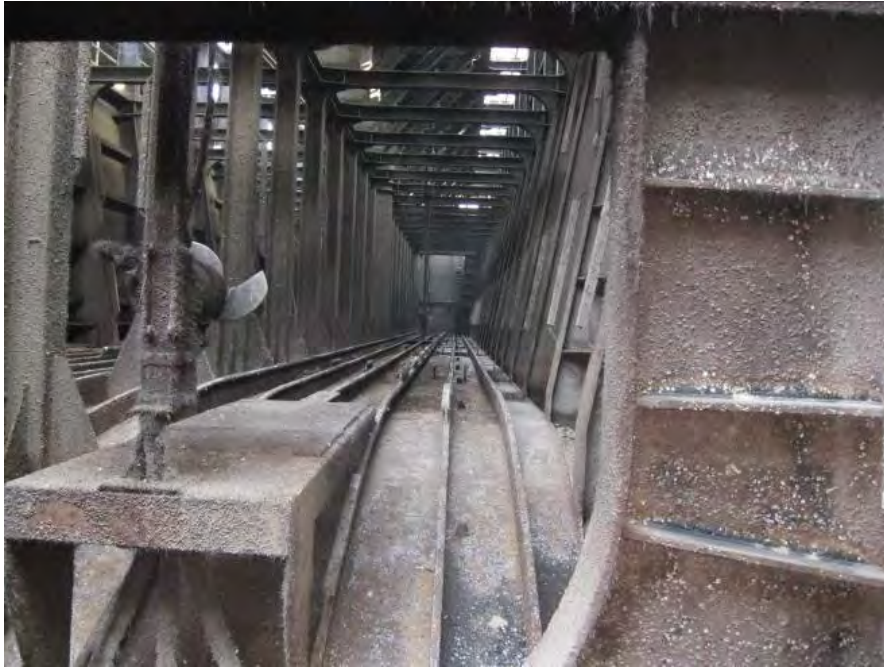
Figure 8-8. Zandvliet Lock, Belgium, mixer for sediment control
