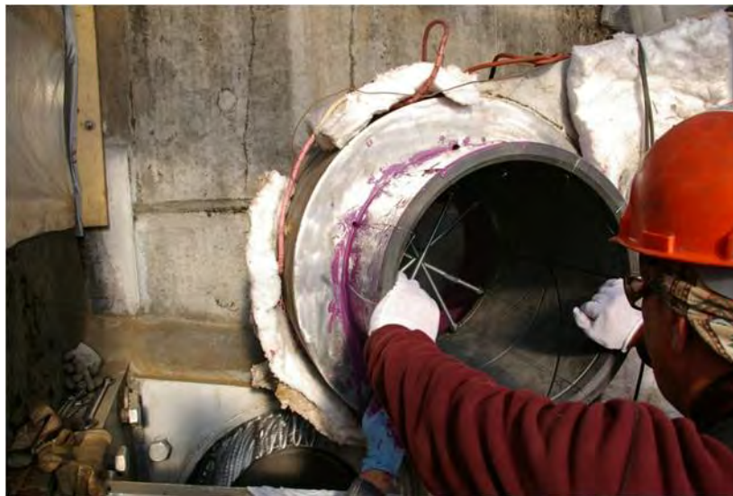
Figure 2-10. Epoxy-bonded bearing
