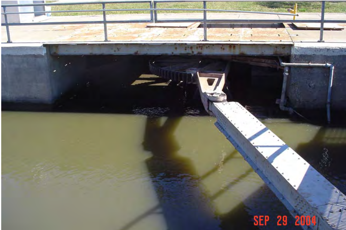
Figure 4-4. LaGrange Lock, Illinois River, Ohio linkage
