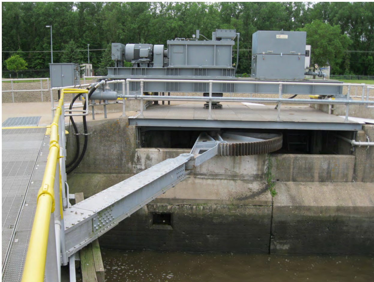
Figure 4-7. Modified Ohio River linkage with raised machinery
