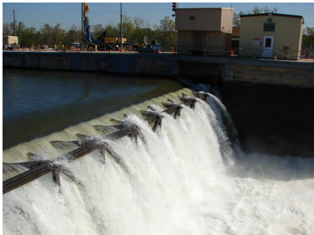
Figure 7-5. Flow over emergency gate
