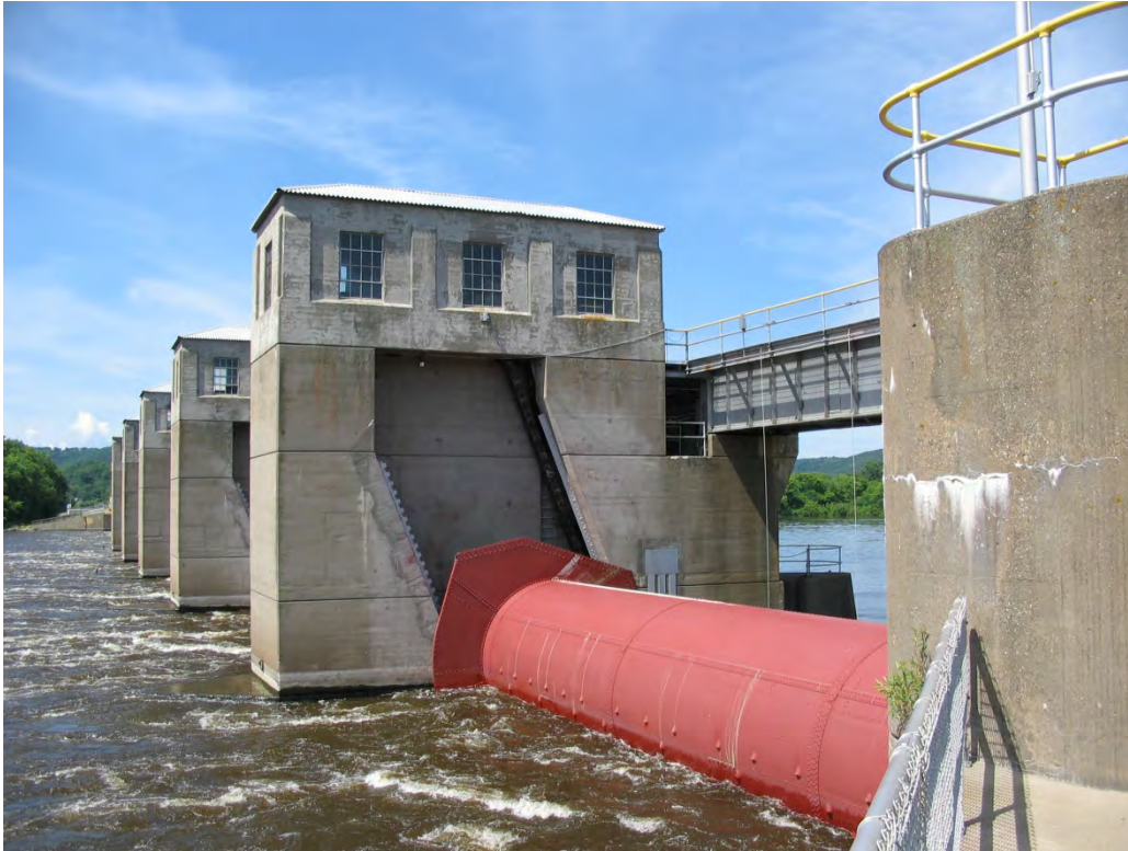
Figure 9-23. Roller gate
