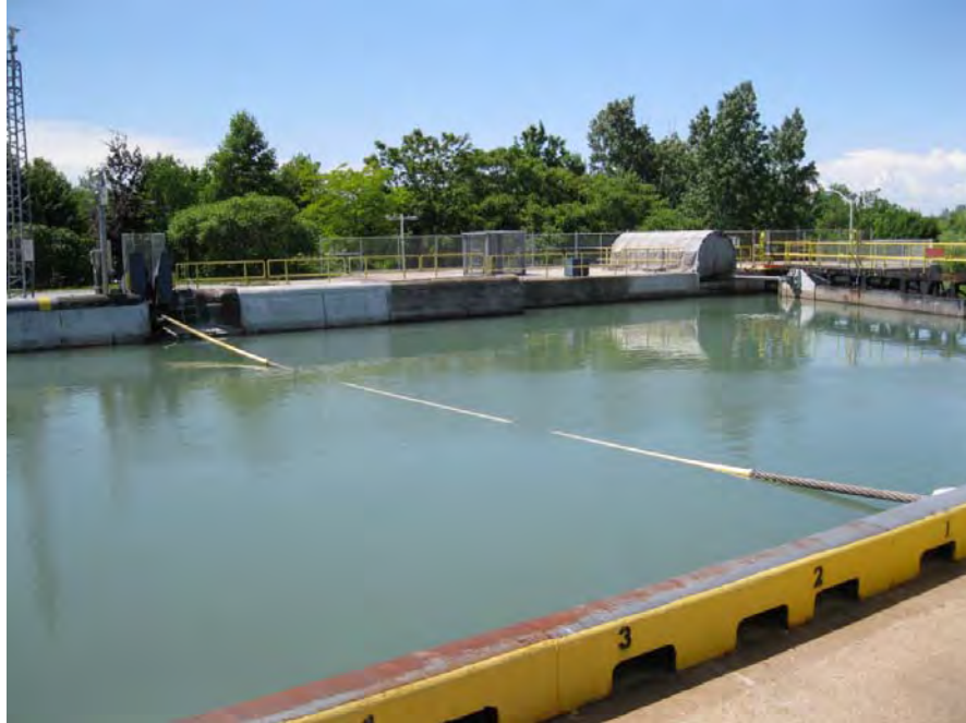
Figure 10-32. Cable set in position, St. Lawrence Seaway
