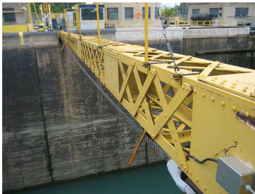
Figure 10-27. Boom and cable, St. Lawrence Seaway
