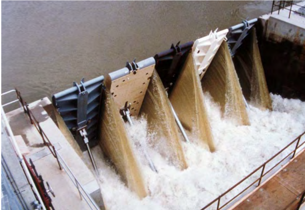
Figure 9-19. Full-scale Olmstead Dam wicket gate prototypes (retractable hydraulic cylinder and direct-connect cylinder styles shown)
