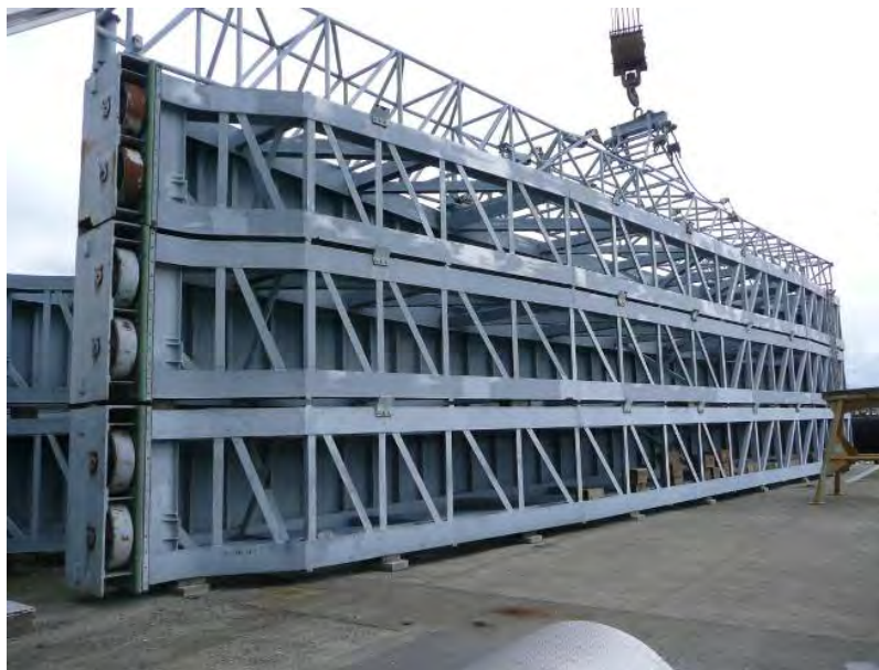
Figure 10-48. Emergency bulkheads, Chittendon Lock, Lake Washington Ship Canal
