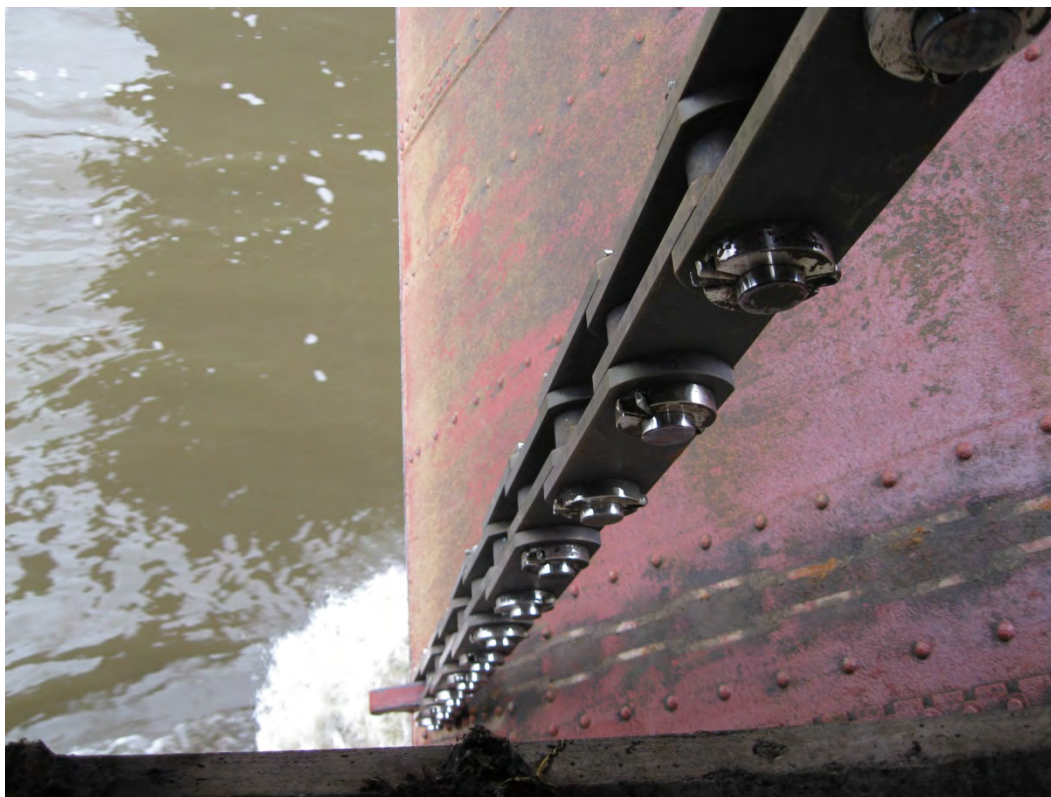
Figure 2-38. Engineered chain installation on a tainter gate
