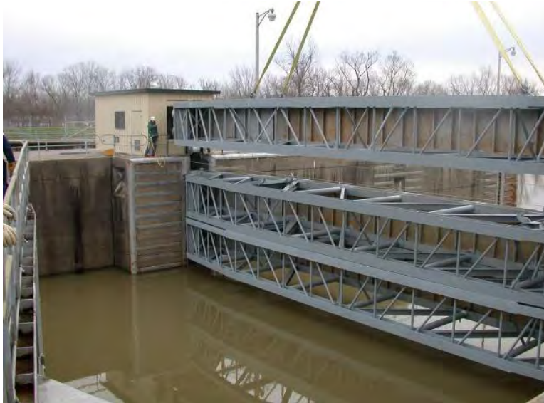
Figure 10-45. Emergency bulkhead system, Old River Lock between Mississippi and Atchafalaya rivers
