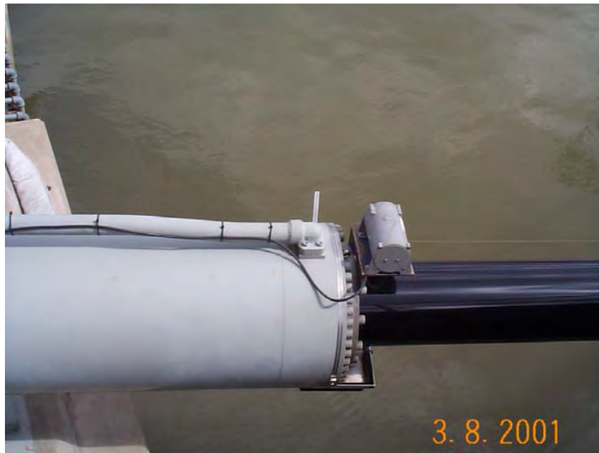
Figure 3-2. Miter gate cylinder with string pot for position sensing
