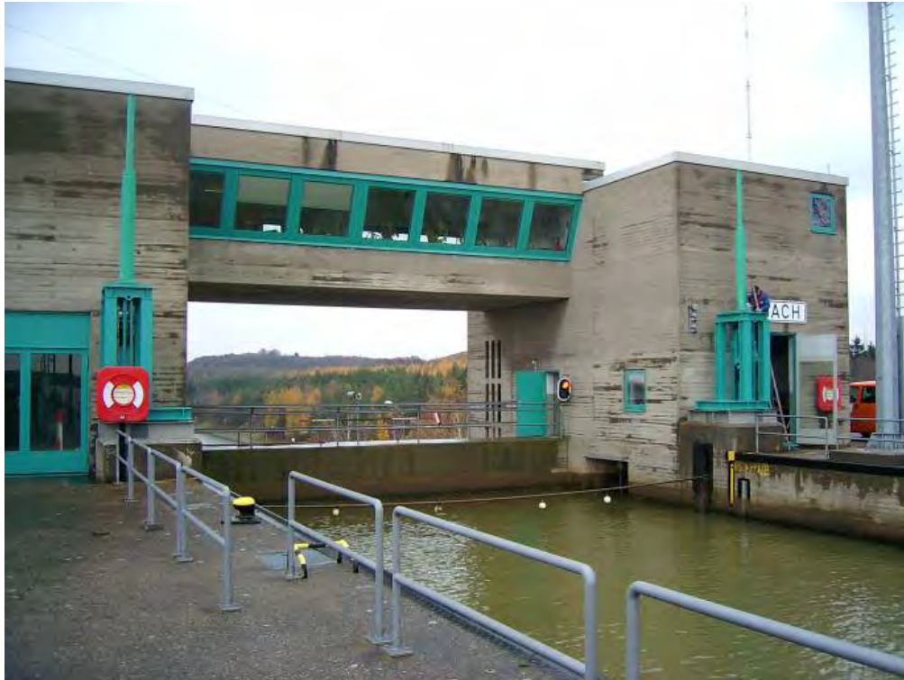
Figure 10-29. Elastomeric ship arrestor system, Lock Eibach, Germany
