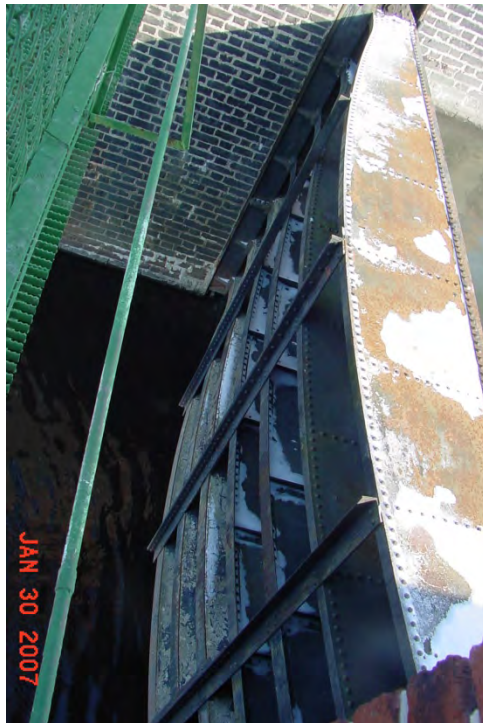
Figure 7-8. Single-section, vertical crest gate
