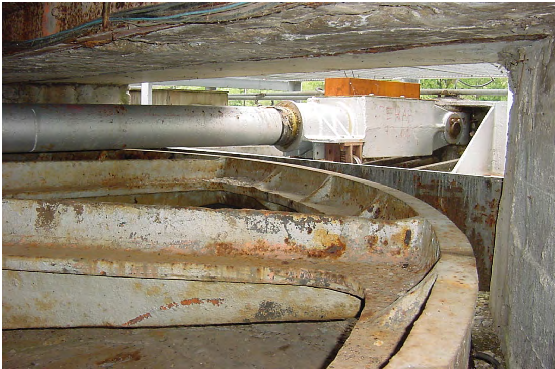
Figure 4-2. Dresden Lock, Illinois River, Panama Canal linkage
