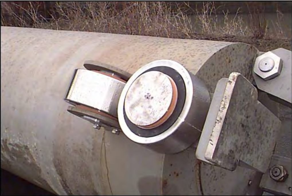
Figure 2-9. Greaseless floating mooring bit roller
