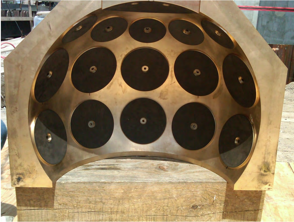
Figure 5-7. Pintle bushing, Caernarvon Canal, New Orleans
