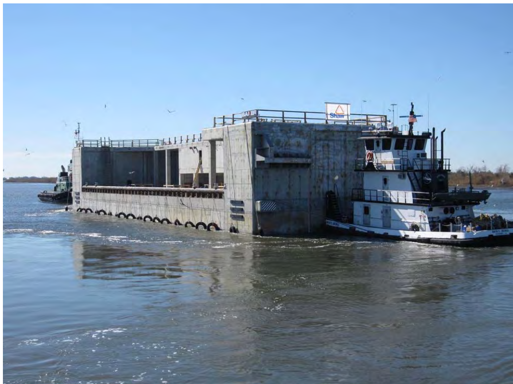
Figure 8-2. New Orleans IHNC surge barrier barge gate
