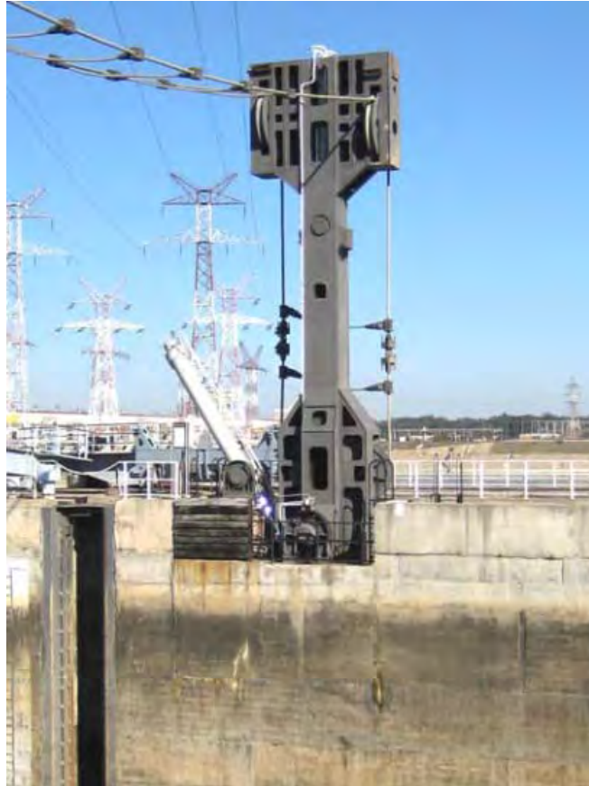
Figure 10-35. Gate protection structure: arms and net lifted to let the ships pass
