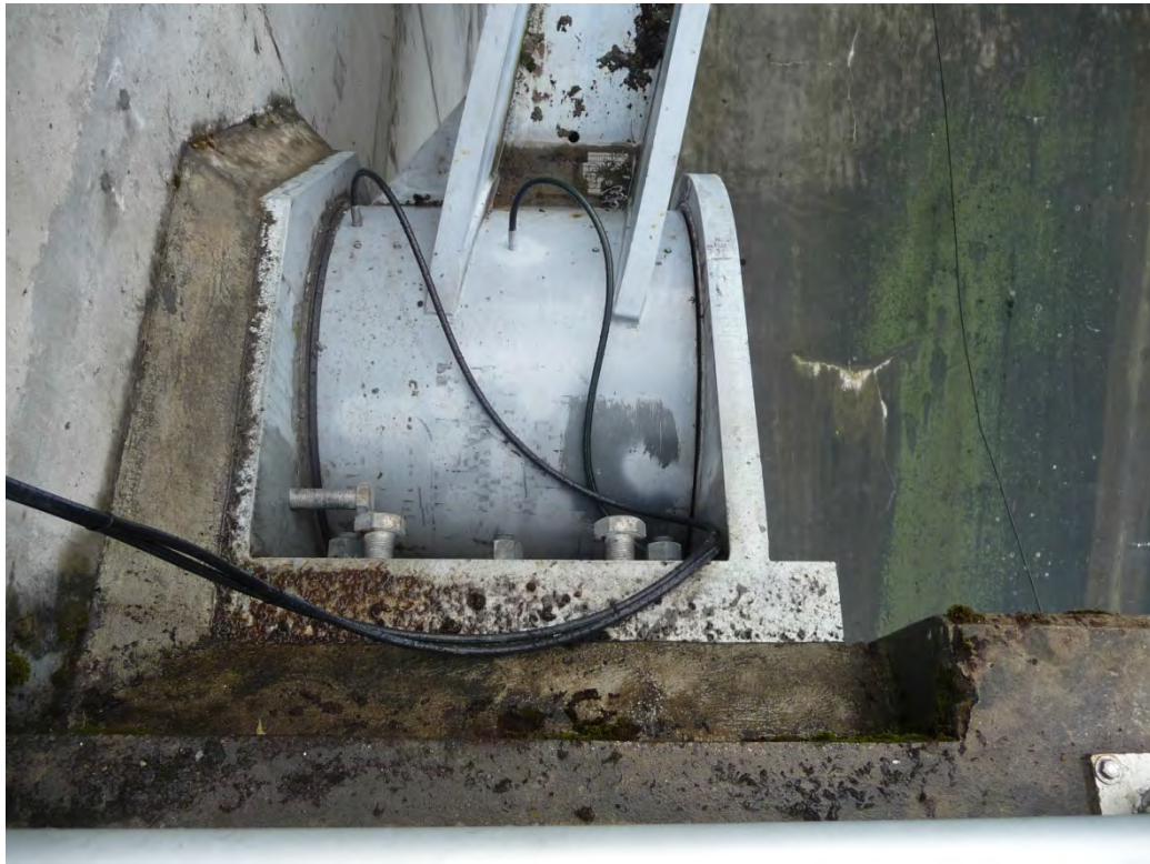
Figure 9-4. Straight sleeve-style trunnion bearing
