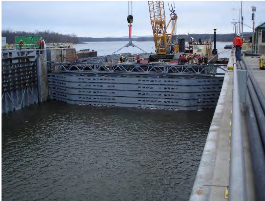
Figure 10-40. Maintenance bulkheads installed by floating plant
