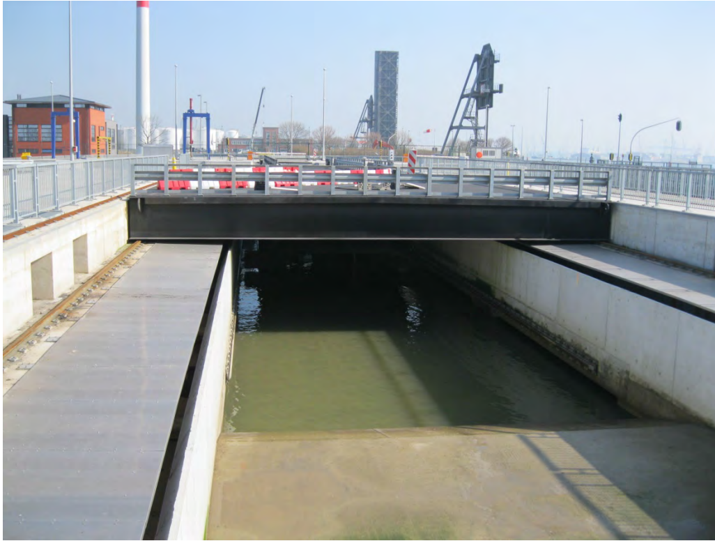
Figure 8-7. Wheelbarrow gate, Van Cauwelaert Lock, Antwerp, Belgium
