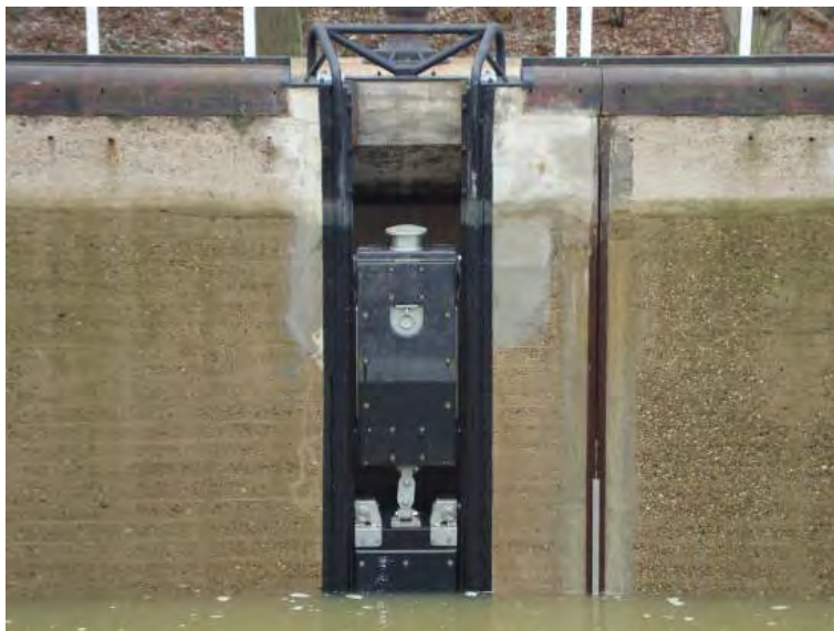
Figure 10-19. Born Locks, bollard is travelling with the water level
