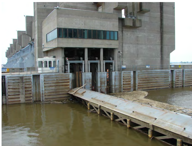
Figure 7-3. Multiple-leaf vertical lift gate
