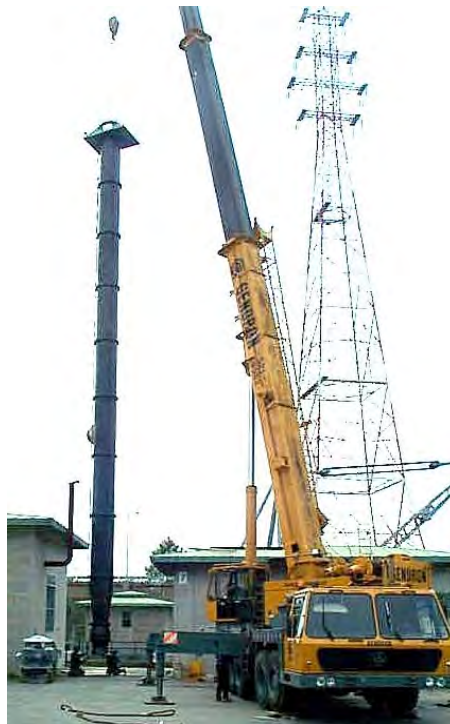
Figure 10-23. Setting a vertical pump, St. Lawrence Seaway
