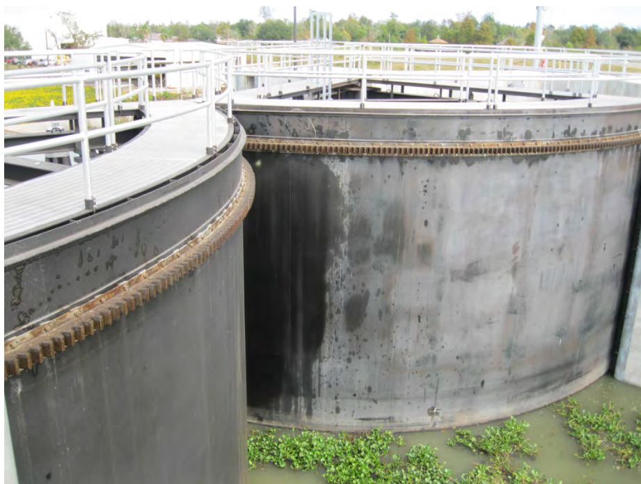
Figure 5-1. New Orleans Caernarvon Canal sector gate
