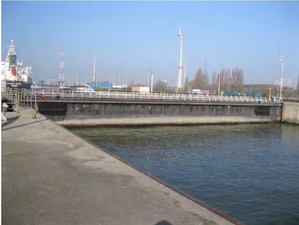
Figure 8-4. Zandvliet Lock, Belgium, rolling gate in closed position
