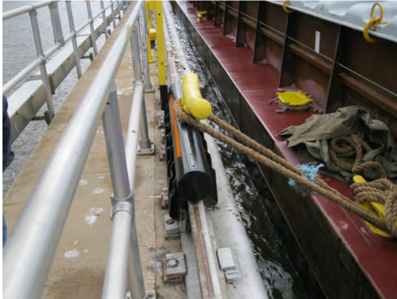
Figure 10-5. Travelling kevel
