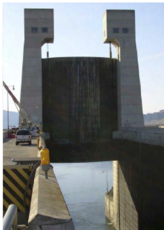
Figure 7-2. Vertical overhead gate
