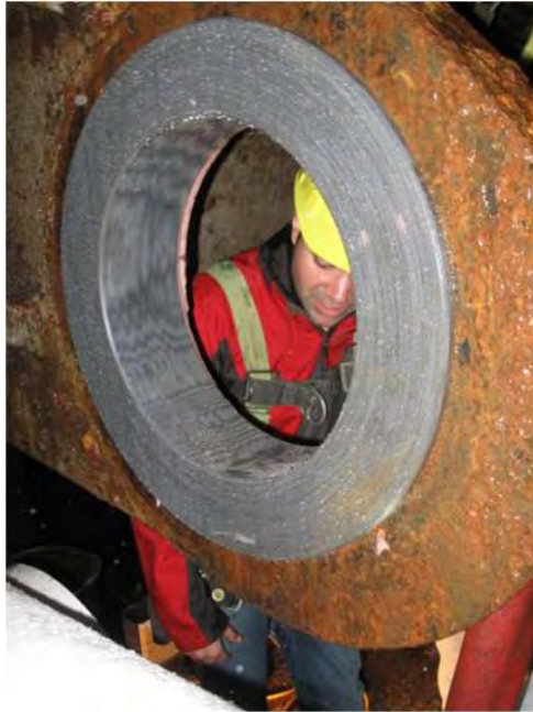
Figure 2-6. Greaseless tainter valve trunnion bearing
