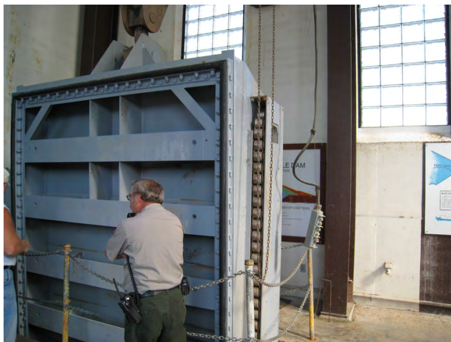
Figure 7-10. Tractor-style gate
