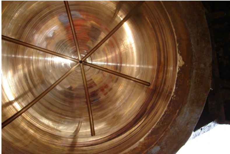
Figure 2-13. Aluminum bronze pintle bushing
