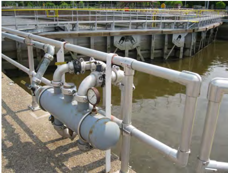
Figure 10-11. Typical diffuser supply system and manifold
