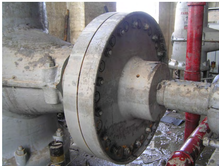
Figure 2-19. Elastomeric coupling
