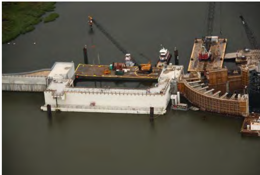
Figure 8-3. New Orleans IHNC barge gate set in position
