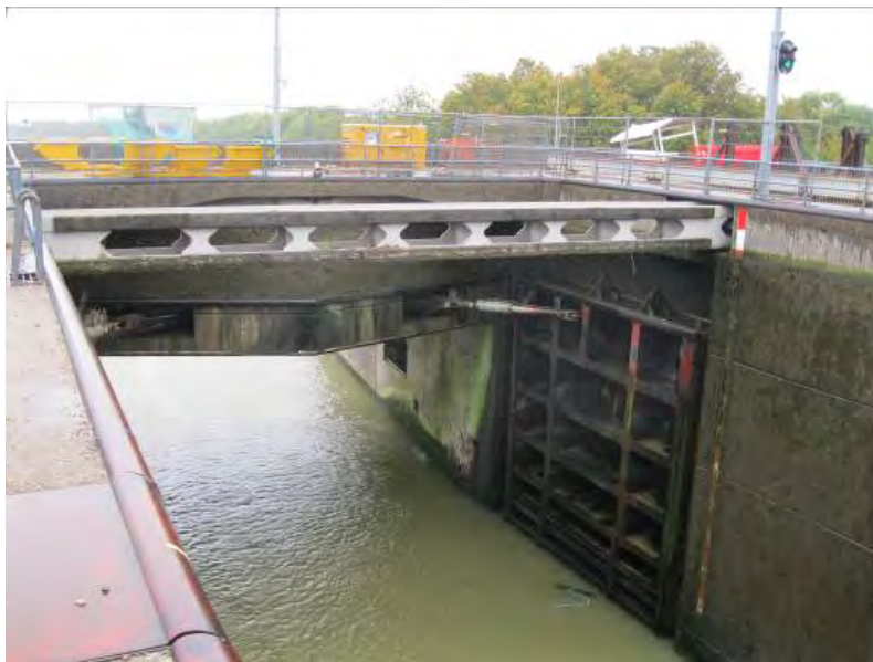
Figure 10-26. Born Locks near Maastrich, Netherlands, fixed arrestor boom
