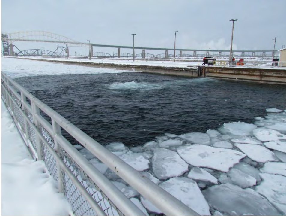
Figure 10-10. Soo Locks, air curtain system in operation
