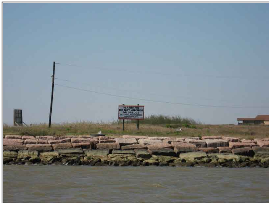
Photo 6 - View of sign within the entrance channel indicating a gas and petroleum pipeline crossing, facing north-east.
