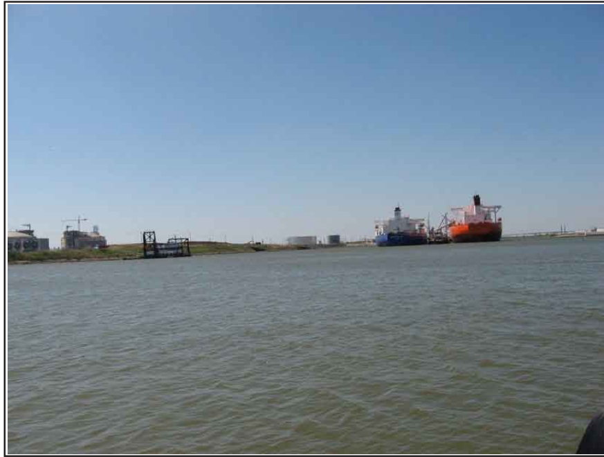
Photo 3 - View of two tankers being offloaded at a facility located adjacent to the Brazosport Turning Basin, facing southwest.
