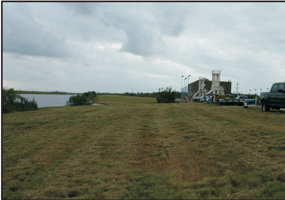
PHOTO 12 General overview of project area, facing west
