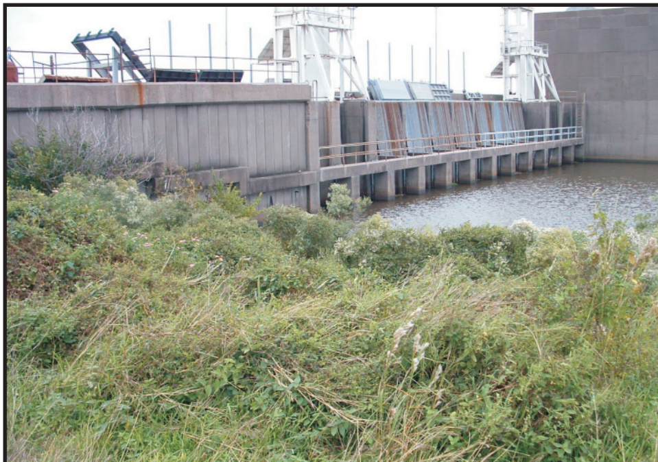
PHOTO 9 East bank of Alligator Bayou, facing southwest
