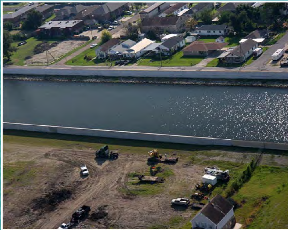
Reconstructed Levees, New Orleans, Louisiana
