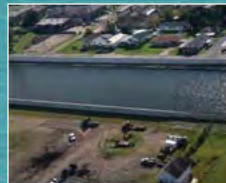
Reconstructed Levees, New Orleans, Louisiana
