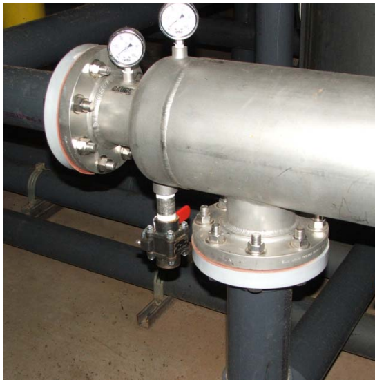
Figure 10-3- Inlet and Outlet Piping
